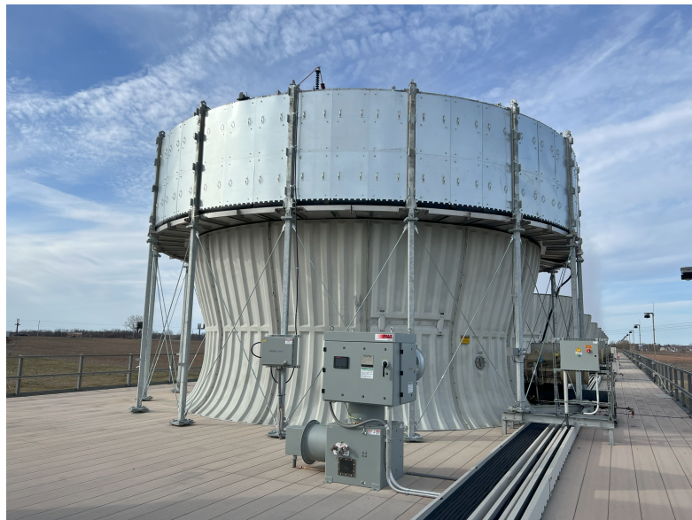
Figure 3 - WaterPanel™ system installed on the fan exhaust of the cooling tower at our partner site
