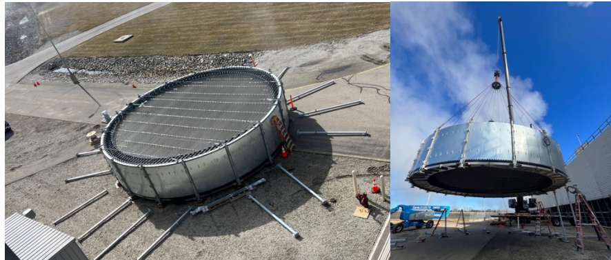
Figure 2 - The WaterPanel™ unit was assembled on the ground, lifted into place utilizing a crane to install the columns to mount the unit over the fan exhaust of the cooling tower
