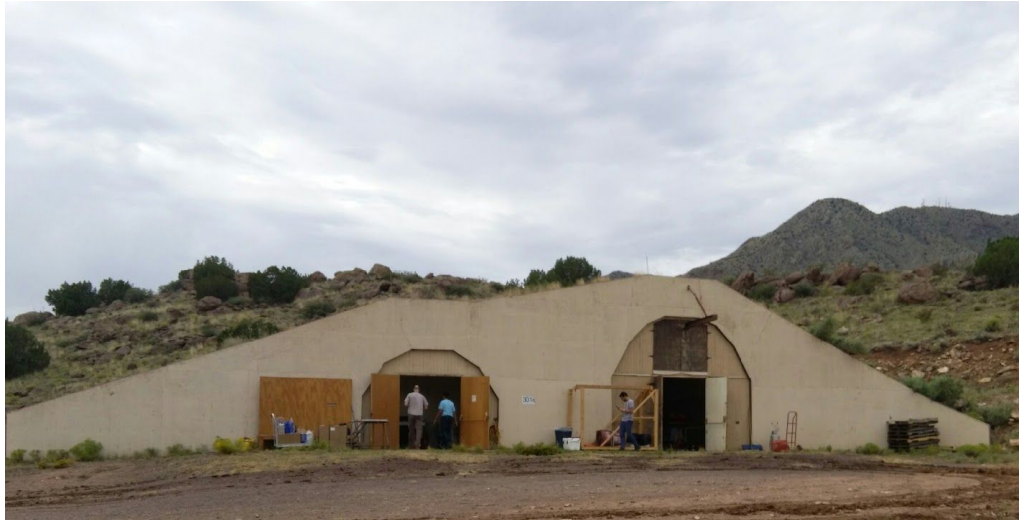
Figure 1. The “2-ton Bunker” near Torres Laboratory. This earth-covered site features a pair of rooms, divided by a robust wall. In the larger room (right) the GB is installed. The smaller room (left) will be exclusively occupied by personnel during testing, allowing safe, remote operation and observation of the experiment.
