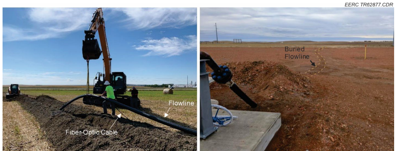
Fig. 3. Images showing the installation of the fiber-optic cable along the CO 2 flowline (left) and the buried flowline and flowline riser at the RTE-10 injection well pad (right).
