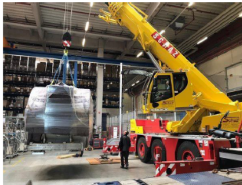
Figure 5-3. 50t Mobile Crane
