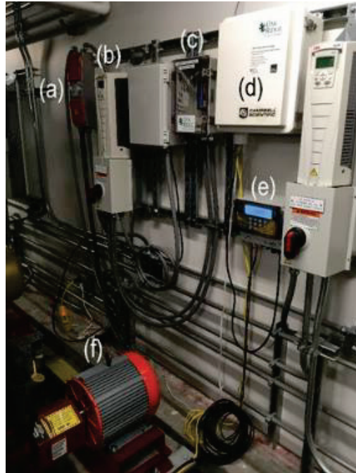
Fig. 13. Equipment and instrumentation for motor performance field demonstration: (a) SMC motor drive, (b) ABB motor drive, (c) power meter, (d) data acquisition system, (e) flow meter display/transmitter unit, (f) SMC motor.
