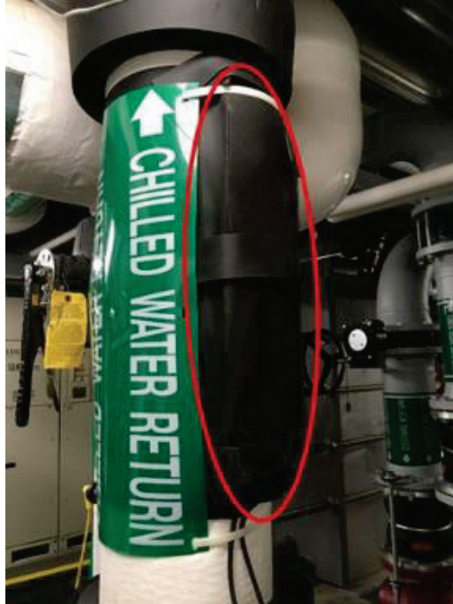
Fig. 12. Location of ultrasonic flow meter (red oval).
