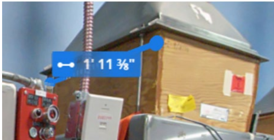
Figure 17. Y Axis Measurement of Hood Filter
