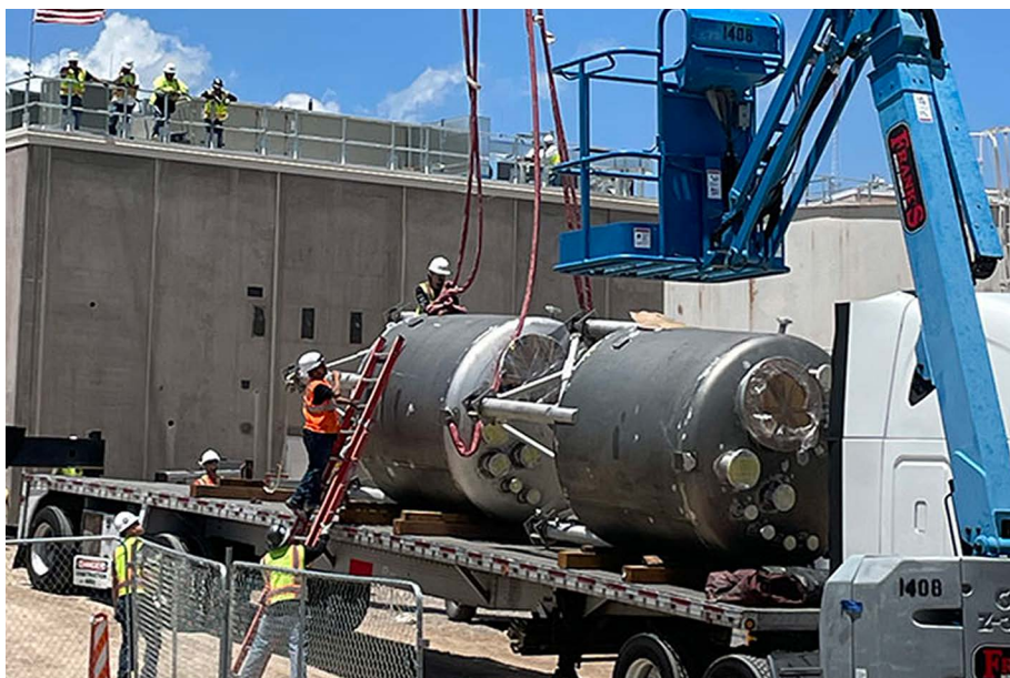
Construction at the new transuranic liquid waste facility. Specially fabricated 2,000-pound tanks were installed that will hold contaminated water during waste processing.
