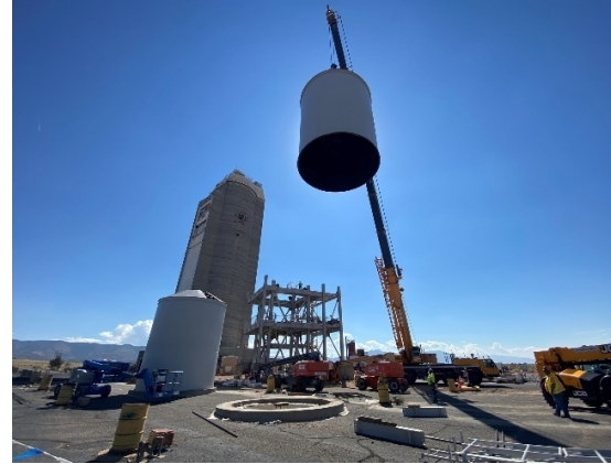
Installing "cold" storage bin
