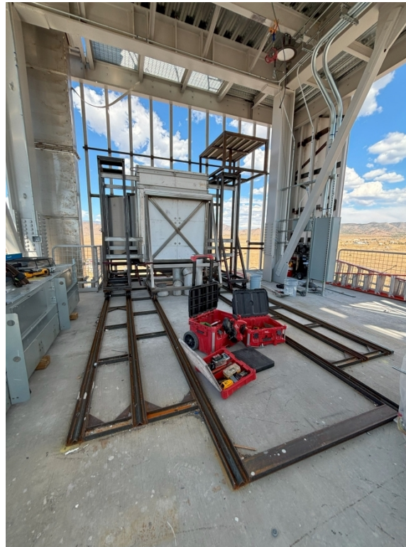
Receiver cavity mounted on a rail system
