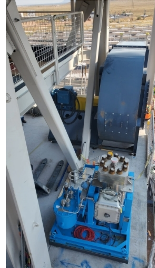
sCO 2 blower (heat rejection) (top) and sCO 2 pump (bottom)
