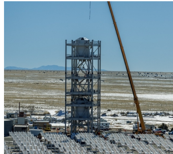
Completed installation of hot storage bin
