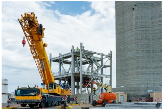
Completed first structural steel splice
