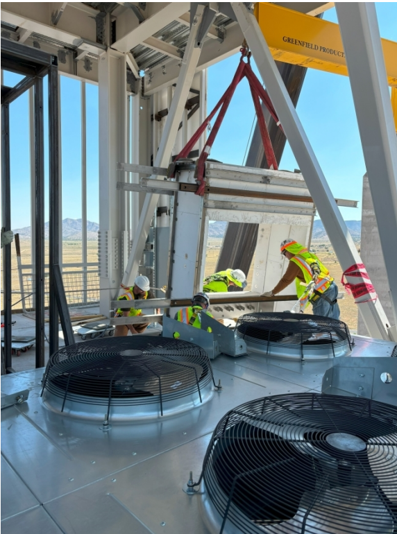
Receiver cavity being lifted into the tower
