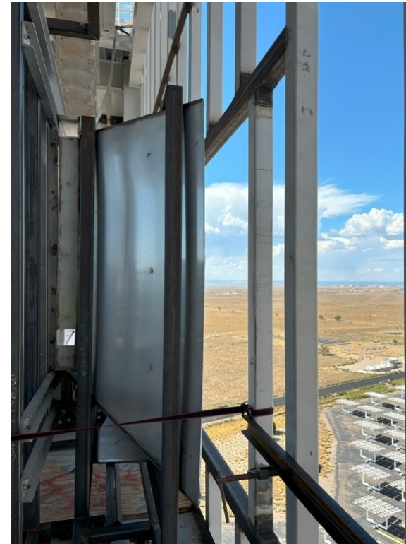
SNOUT interface with spillage board rails
