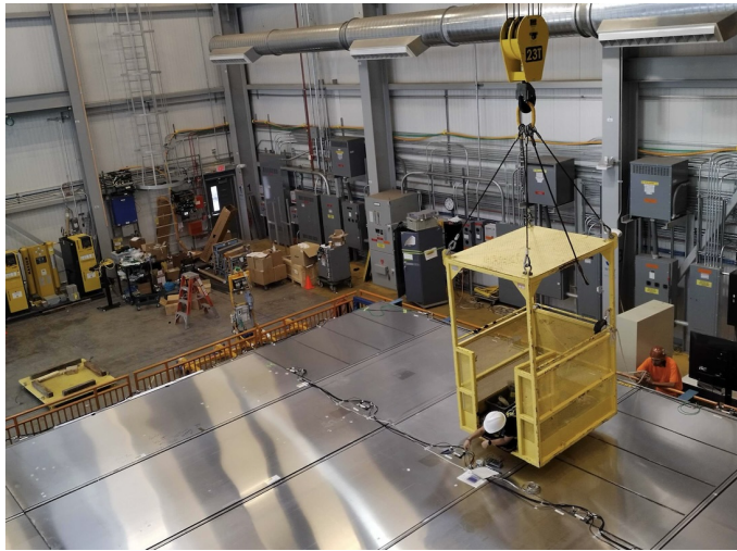
Figure 5.2: Photo of me working from the basket to ground the modules of the CRT Top High.
