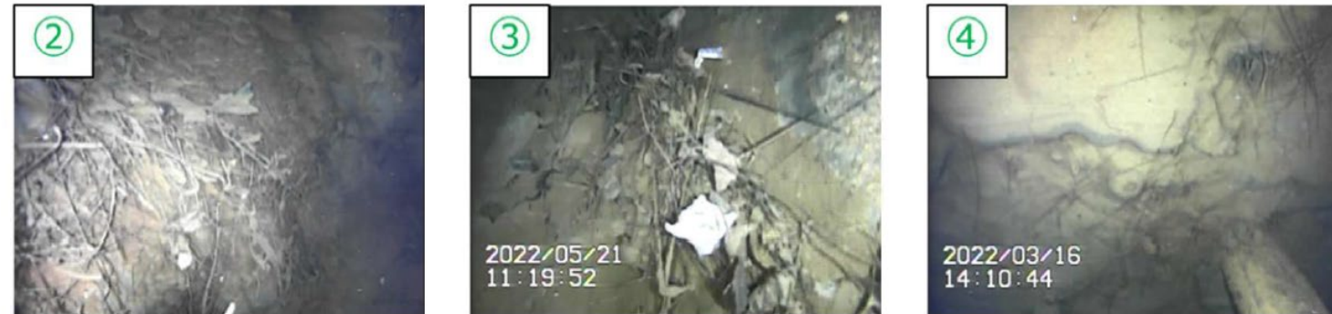
Figure 7. Thread-like deposits (point ② to ④ in Figure 5) [3]
