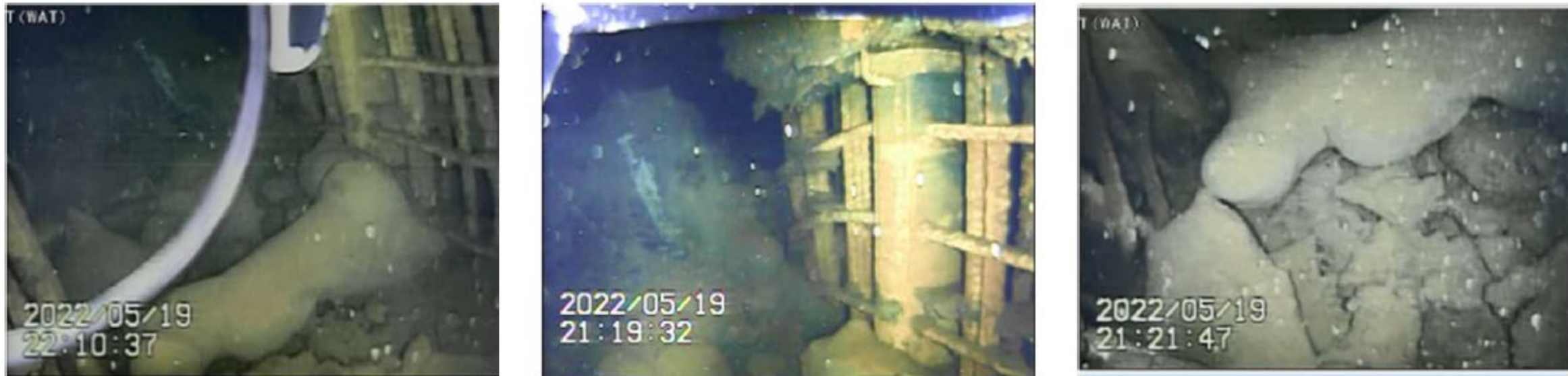
Figure 6. Bulky deposits (around point ① in Figure 5) [3]
