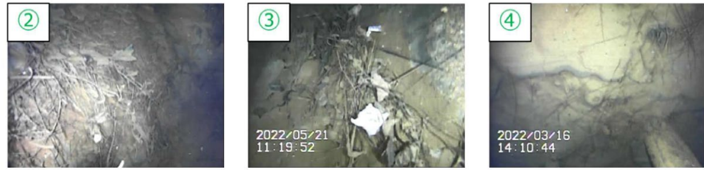
Figure 6. Bulky deposits (around point ① in Figure 5) [3]
