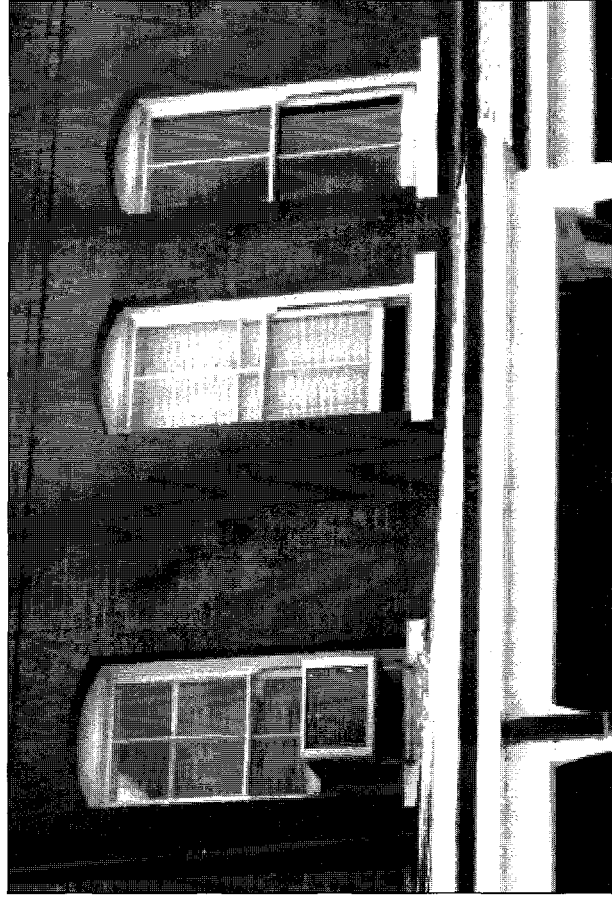
The open window in the center provides free ventilation and cooling. Ironically, the unnecessary air conditioner on the left prevents similar use of that window and damages the building's historical integrity.
