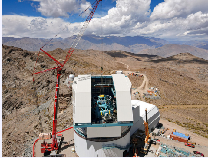
Construction at the Vera C. Rubin Observatory. Credit: ESA/Hubble, Rubin Observatory/NSF/AURA.
