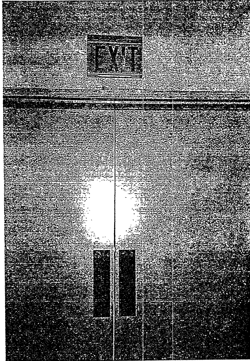
Figure 9a. Notice large gap in between doors
