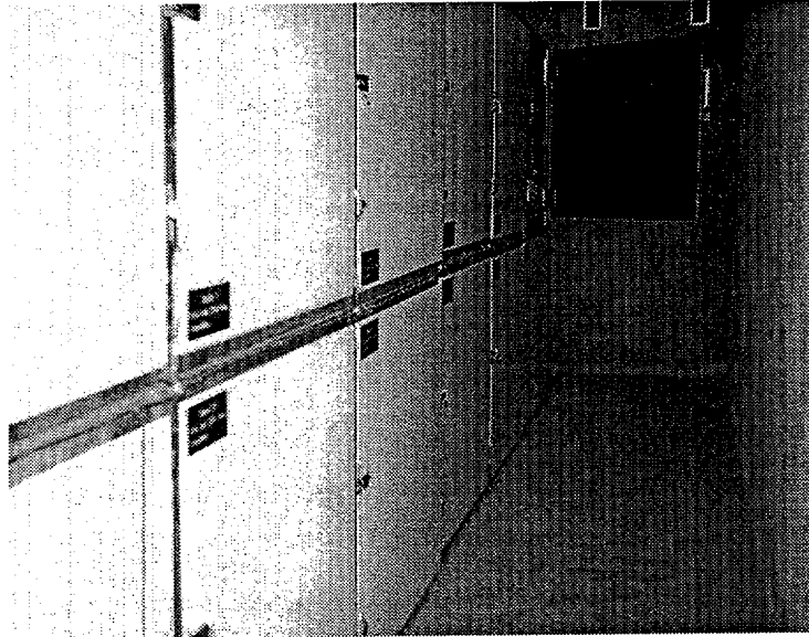
SIFCON CABINETS INSIDE A STORAGE MAGAZINE
