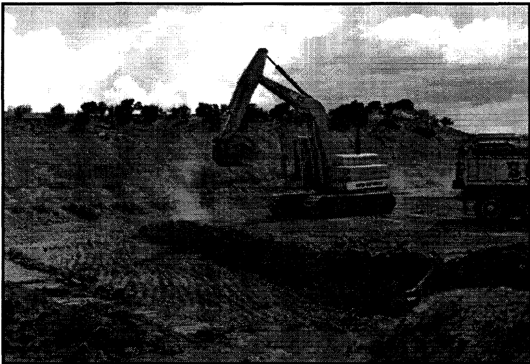
Figure 23. Construction of Sand Pit (Area 4) Showing Excavator in Action
