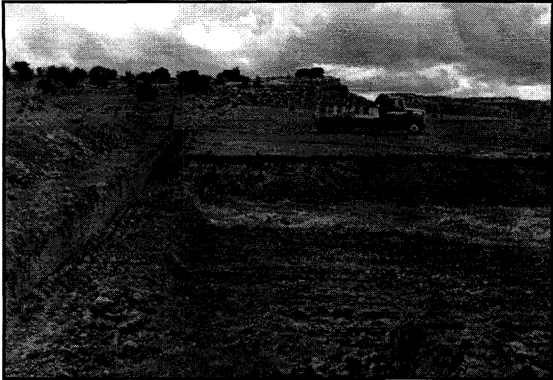
Figure 22. Construction of Clay Pit (Area 5) Showing Pit Boundary
