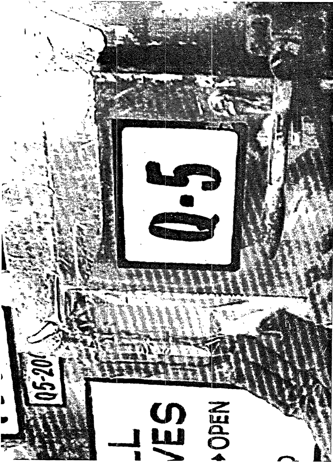
Figure 15. Q-Cell Samplers Being Sealed Shut With Silicon Rubber and Tape During Deactivation Project.
