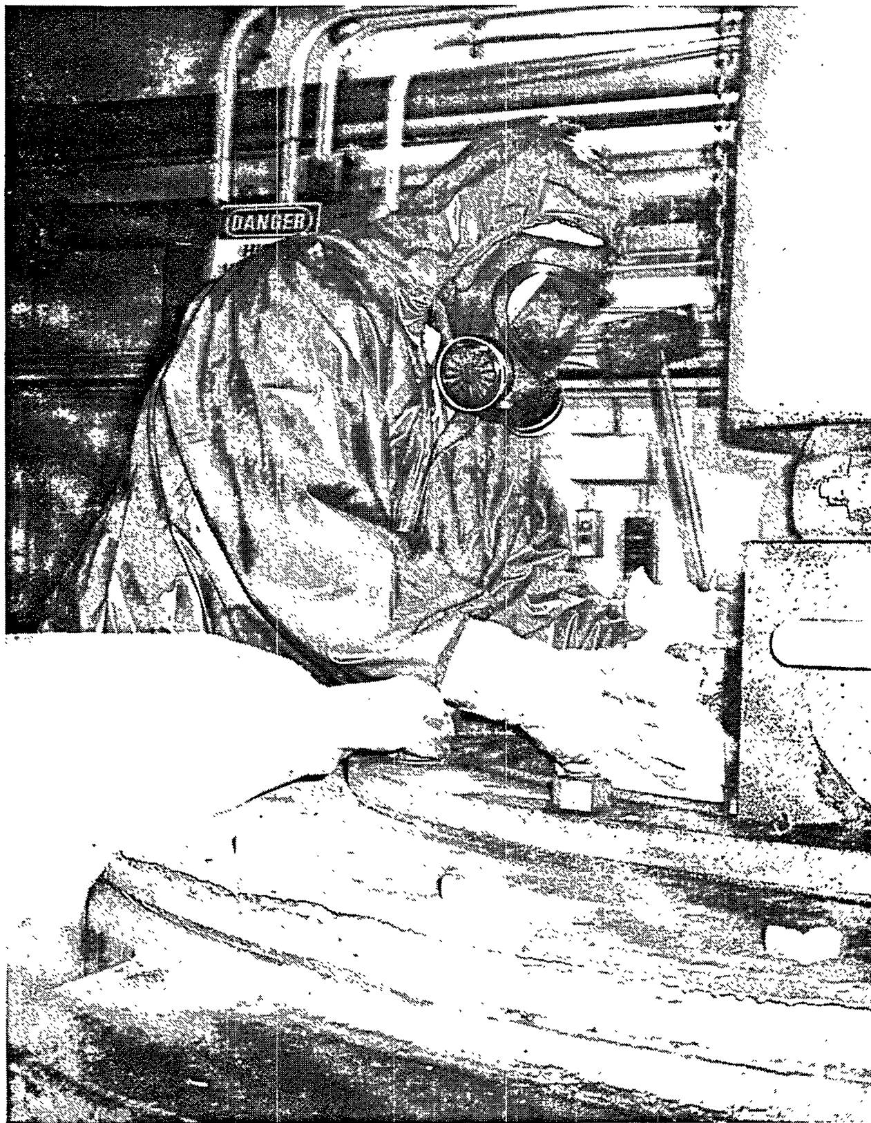
Figure 27. Workers Remove Contaminated Hydraulic Oil From \text{UO}_3 Calciner (1994).
