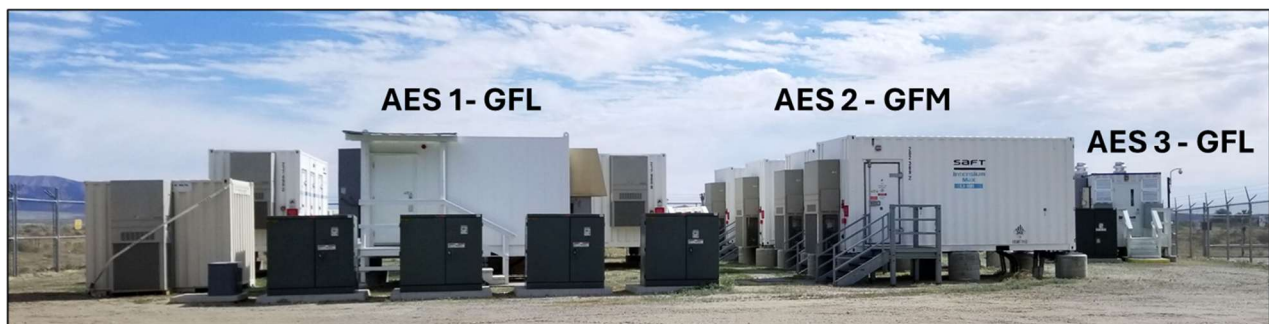
Figure 35: Borrego Springs Microgrid upgraded energy storage IBRs.
