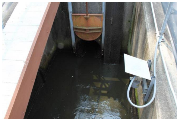
Exhibit 4-4. Flow Sensor and Discharge Valve
