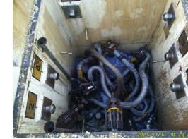
Image of a typical SST pit (with shield blocks removed)
