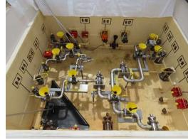
Image of a typical DST pit (with shield blocks removed)
