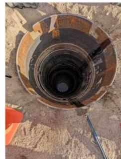
Caissons Installed and Concrete Core Removed
