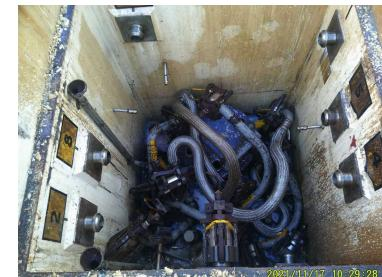
*Photo of a typical SST pit with shield blocks removed*
