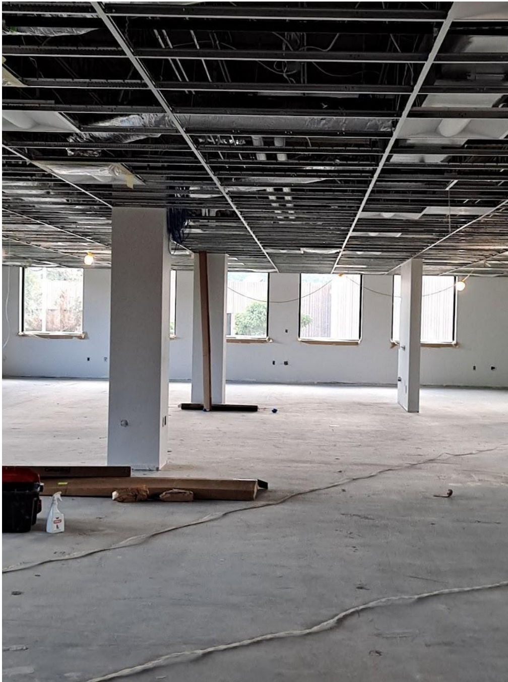
Figure 4. Denver Federal Center Building 40's west wing second floor.
