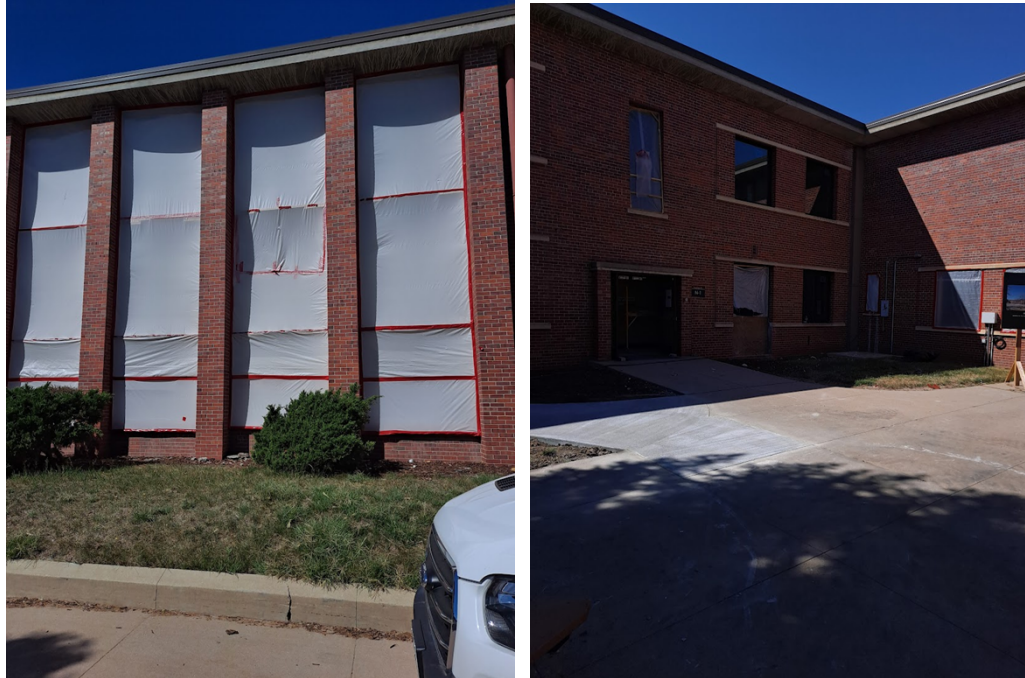
Figure 2. Denver Federal Center Building 40.
