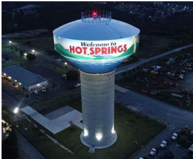
Figure 5-25 11,300 m 3 (3,000,000 gallon) Elevated Water Storage Tank
