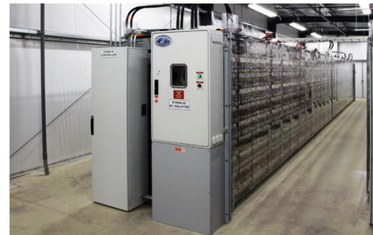
Installed 2012, Lead-based Ultra-battery used for frequency regulation at Lyon Station, Pennsylvania 3.6 MW power capability
