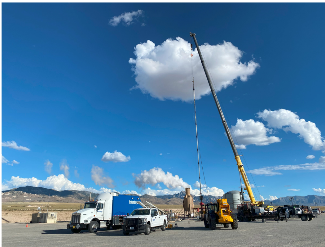
Figure 4-9: Utah FORGE Well 16B test site with lubricator stacks for chemical tool.
