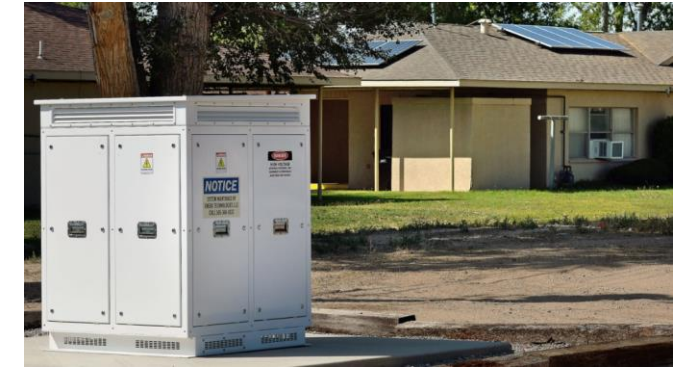
BlockEnergy Nanogrid Serving Residential Housing Loads
