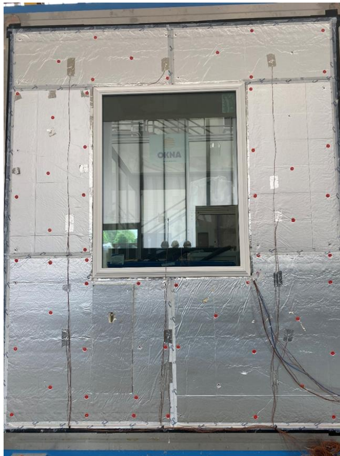
Figure 5. Wall after installation of hydrobox and insulation layer
