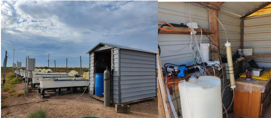
Figure G3-15. The installed DIC feeding system in 900-L raceway ponds at the Qualitas Health facility.
