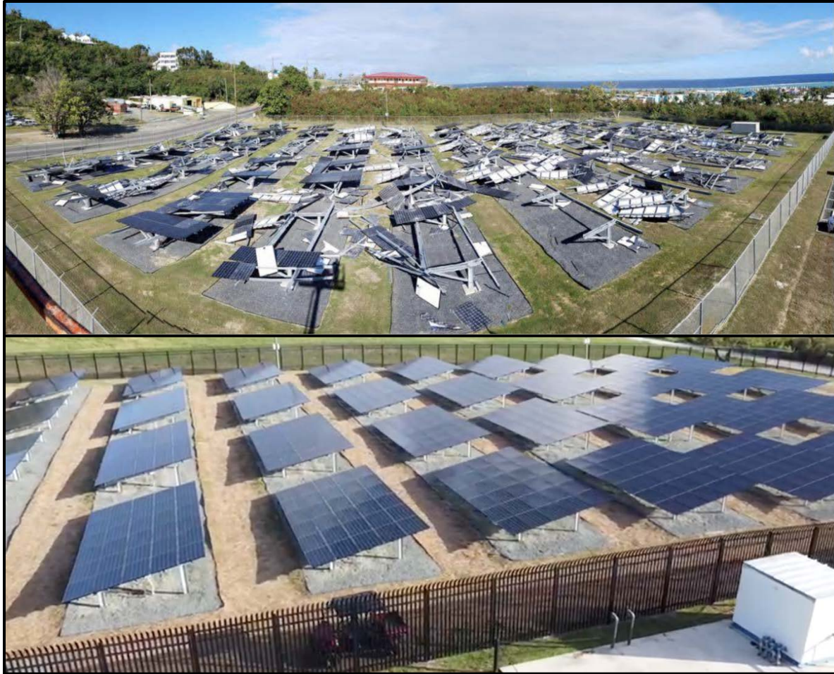
Figure 1. Storm damage at St. Croix after Hurricane Maria (top) and after Hurricane Fiona (bottom).
