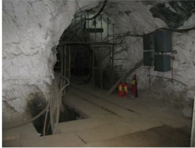
Figure 5.1: The Jaduguda UCIL mine site. The experiment is proposed to happen inside this cavern.
