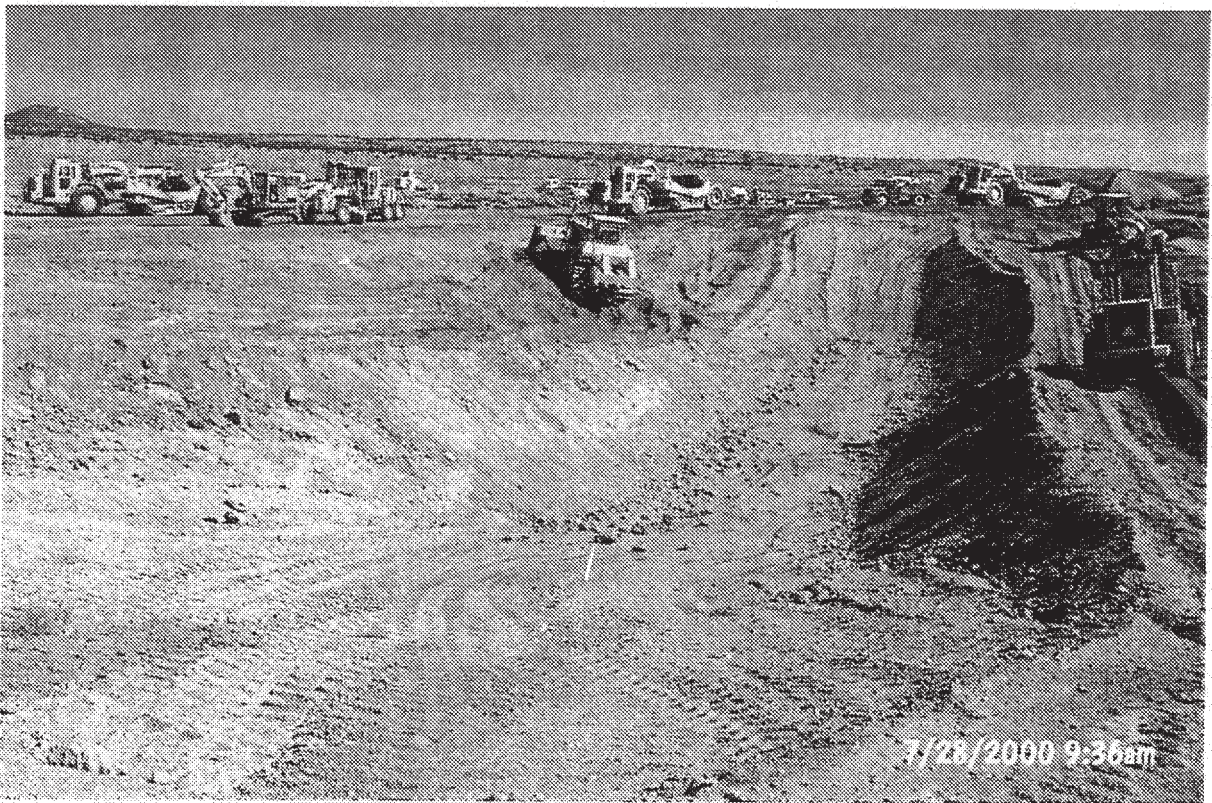
PHOTOGRAPH 6 - Excavation of the CMP Mud Relocation Trench
