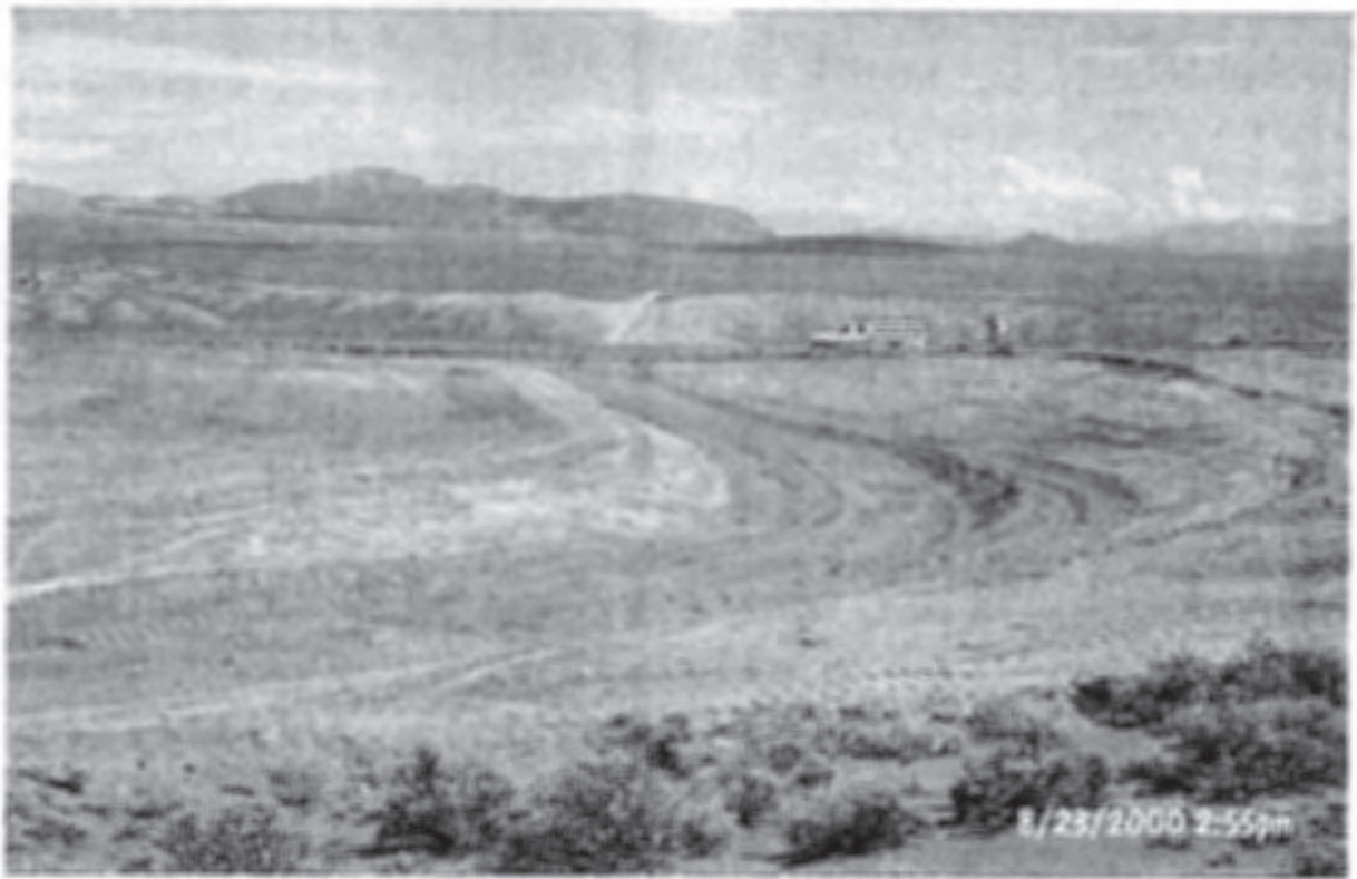
PHOTOGRAPH 15 - South portion of the West Diversion Channel
