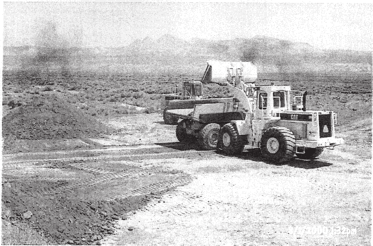
PHOTOGRAPH 25 - Clean closure by excavation of UC-1 Area S, CAS 58-10-03
