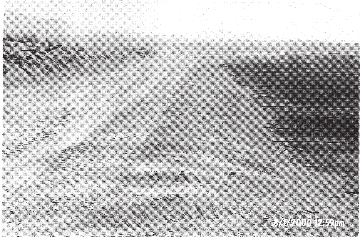
PHOTOGRAPH 3 - Geogrid anchored in place on CMP
