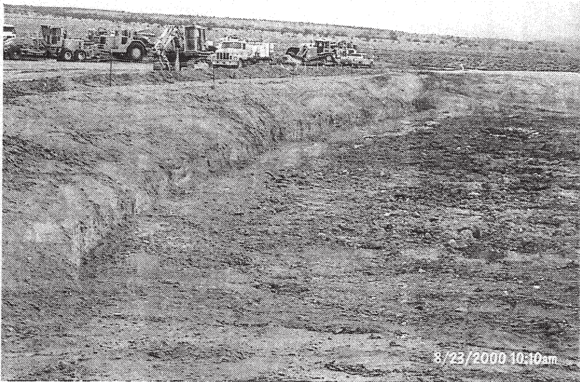
PHOTOGRAPH 12 - Geogrid anchor bench, west side of Mud Relocation Trench
