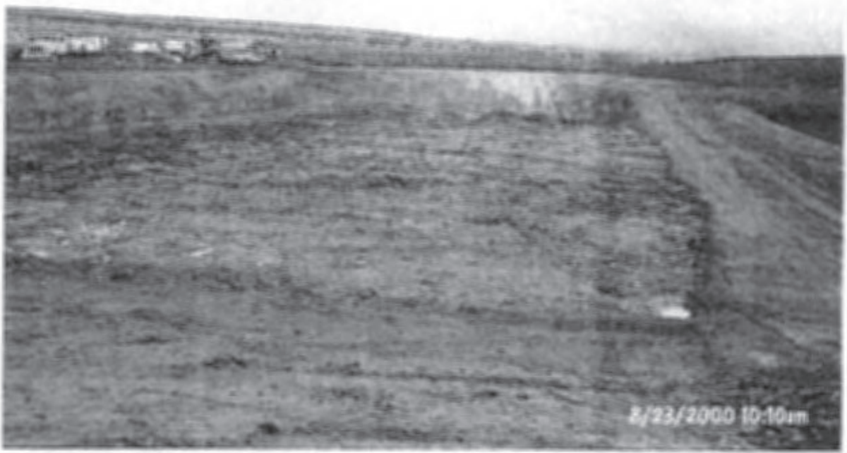
PHOTOGRAPH 11 - Filled CMP Mud Relocation Trench
