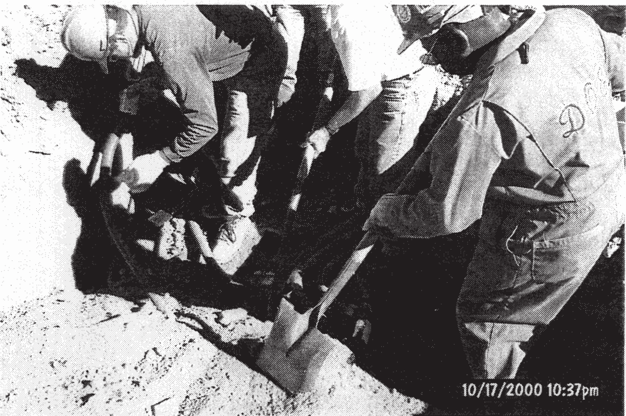
PHOTOGRAPH 22 - Placing and burying TDR sensors in CMP cover
