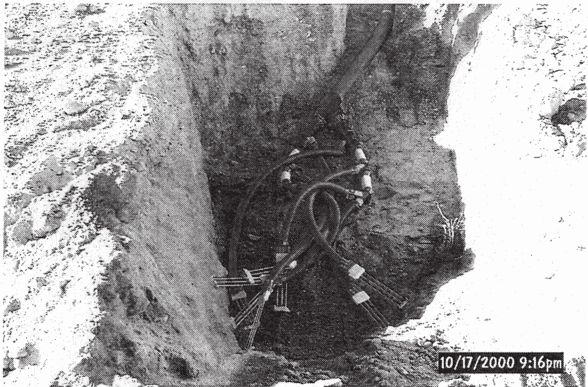
PHOTOGRAPH 21 - Installing TDR sensors in CMP cover
