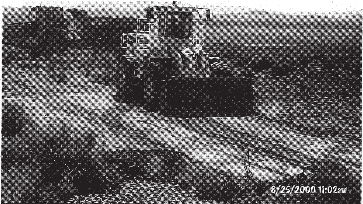
PHOTOGRAPH 26 - Clean closure by excavation of UC-1 Area Y, CAS 58-44-06
