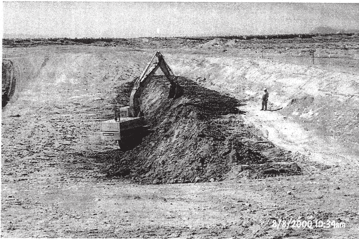
PHOTOGRAPH 10 - Leveling drilling material surface with Track Hoe
