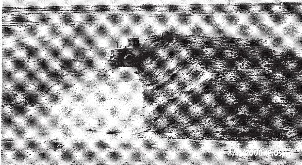
PHOTOGRAPH 9 - Stacking drilling material in the Mud Relocation Trench
