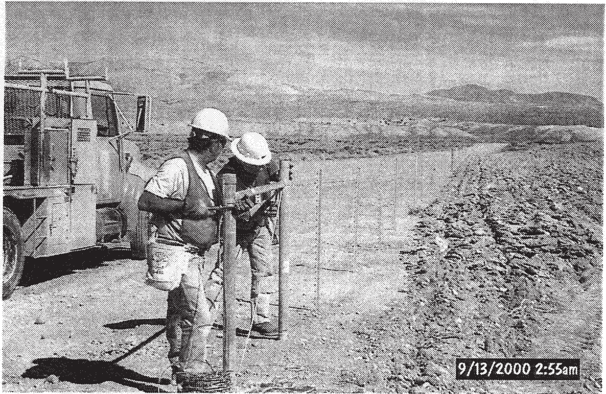
PHOTOGRAPH 17 - Erecting the CMP cover fence
