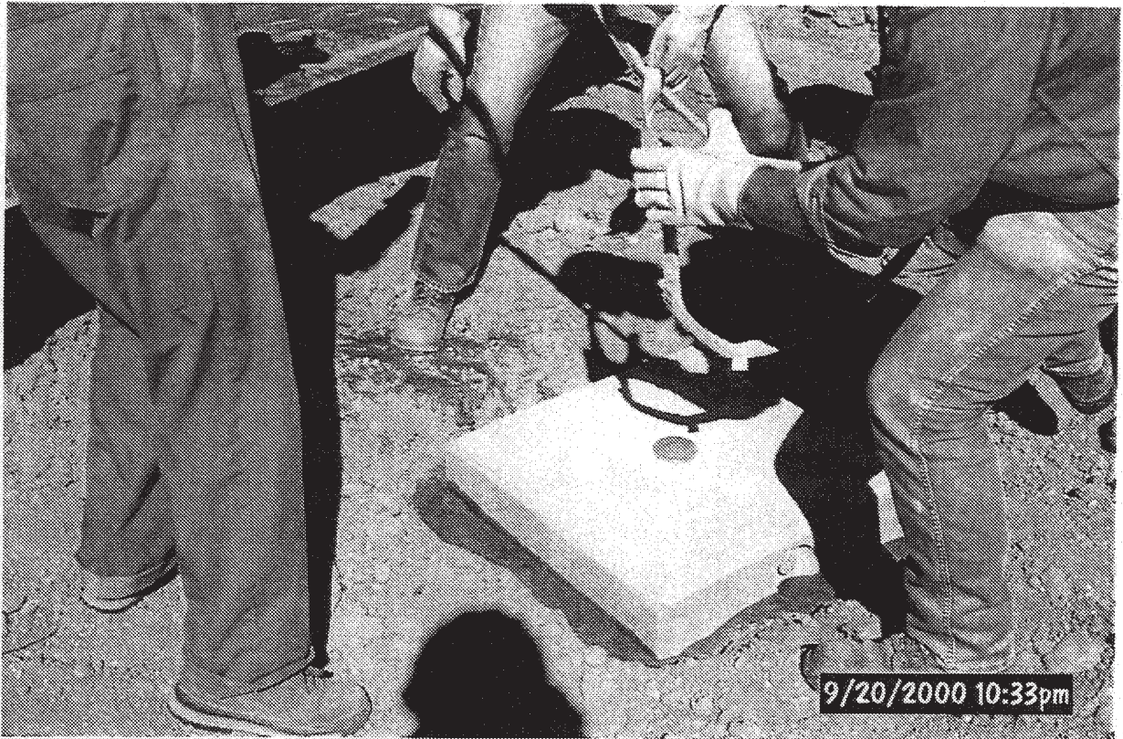
PHOTOGRAPH 20 - Placing subsidence monuments on the CMP cover
