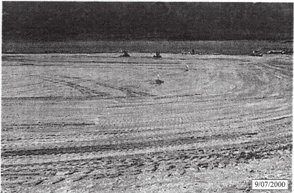
PHOTOGRAPH 14 - Completed 4 foot earthen mono-layer CMP cover
