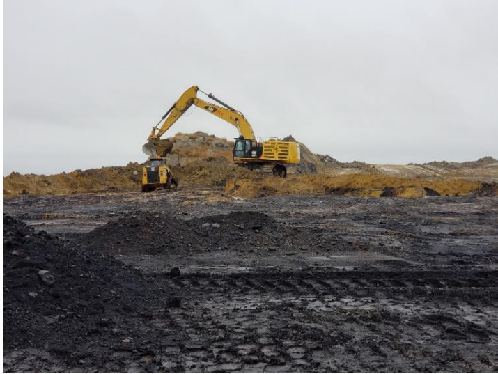
Figure 3. Removal of Overburden and Cleaning of the Top Mine Waste Layer.
