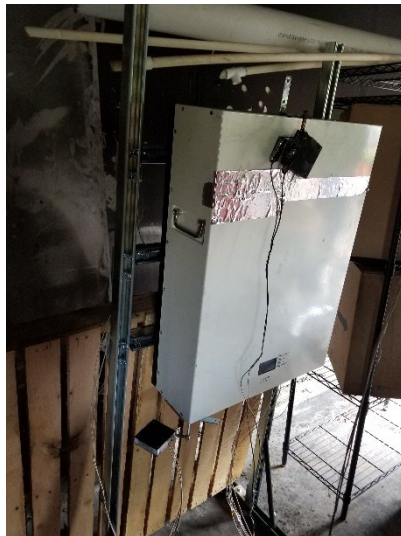
Figure 4 (ESS Mounted in Garage)
