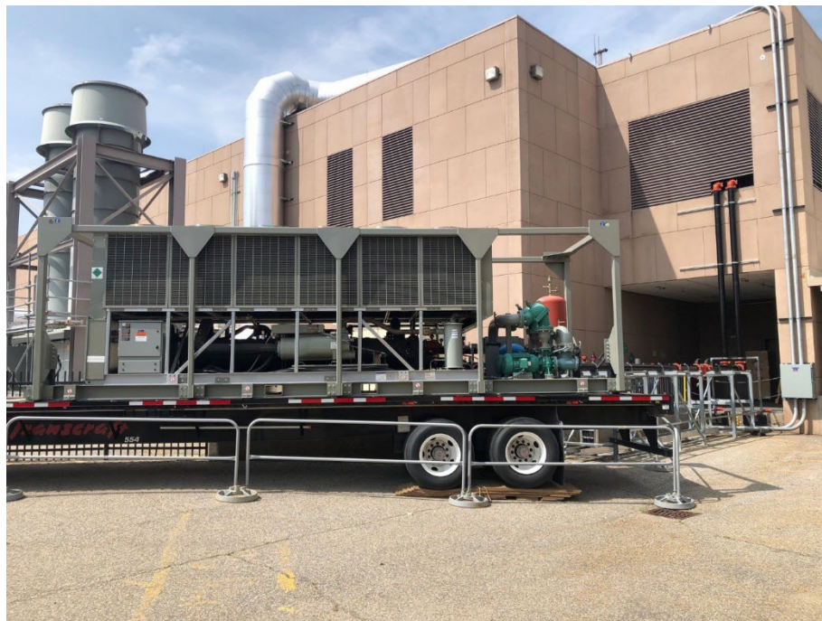
Figure V.I-3: MST Chiller (McEahern, 2021)
