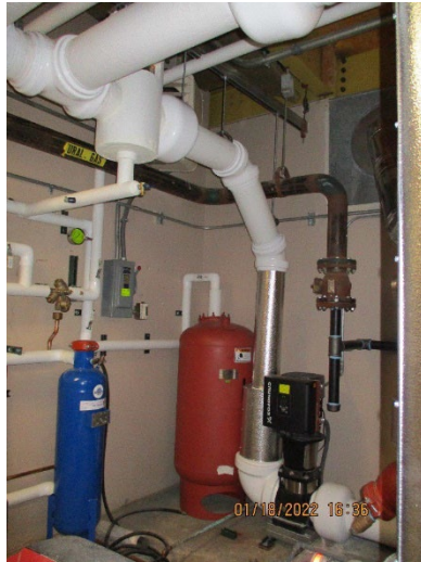
Figure V.I-7: Primary Pump 2022 (McEahern, 2022)
