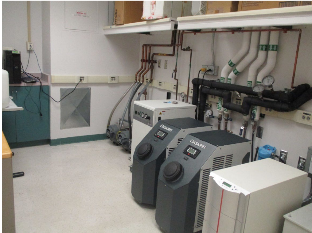
Figure V.III-4: MST Small Chillers
