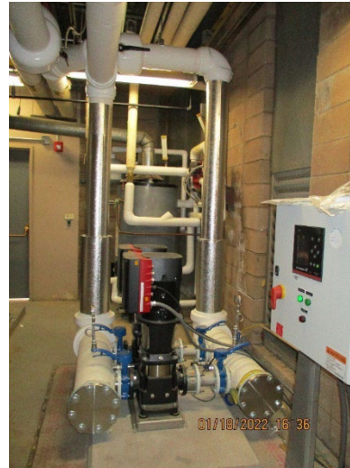
Figure V.I-7: Primary Pump 2022 (McEahern, 2022)
