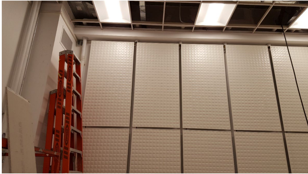
Figure V.III-5: MST Radiant Cooling
