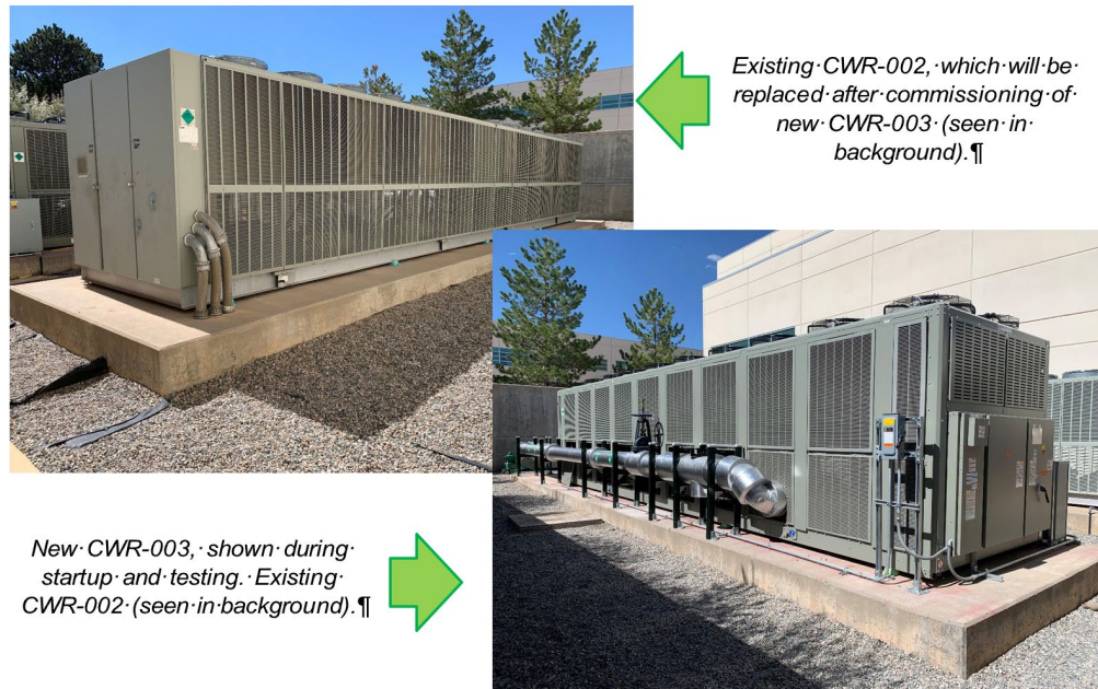
Figure V.I-4: Global Security Chillers (McEahern, 2021)
