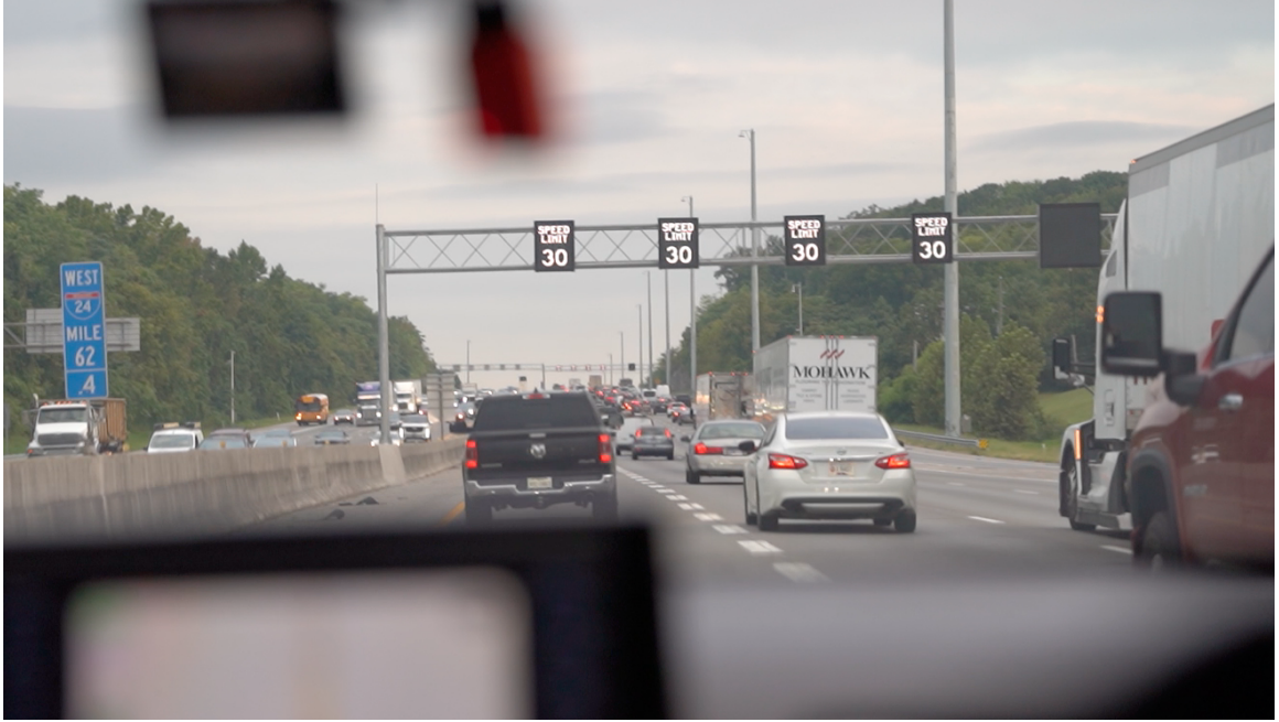
Figure 6.1: Movie 1: Variable speed limit (VSL) system activated and posting 30 mph speed limit during congested traffic. Photo taken from the ego vehicle which automatically adjusts its velocity to 30 mph in response to the VSL system. View a video associated with this work at: https://youtu.be/gFwJfEvnogI?si=BC_smYujNFJ2Adj .
