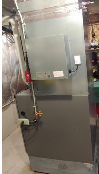
Figure 13 - Furnace and blower cabinet with new heat pump coil installed above. The available vertical space to install this coil in place of the old cooling coil was assessed as part of the system selection.
