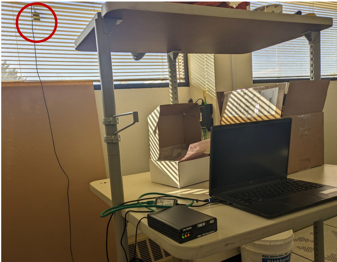
Figure 19. New GPS Timer Hardware where the antenna is located within the red circle.
