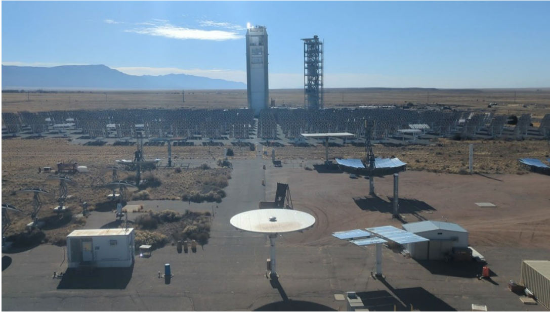
Figure 67. Heliostat Field on Calibration Panel.
