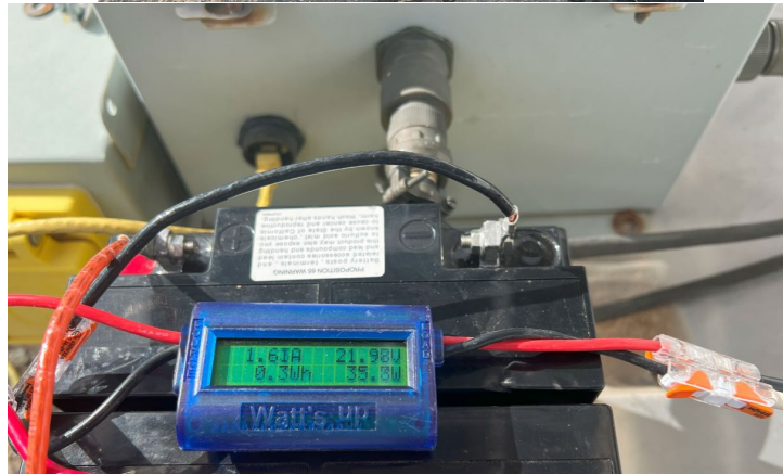
Figure 53. NSTTF heliostat on-board power setup and demonstration.
