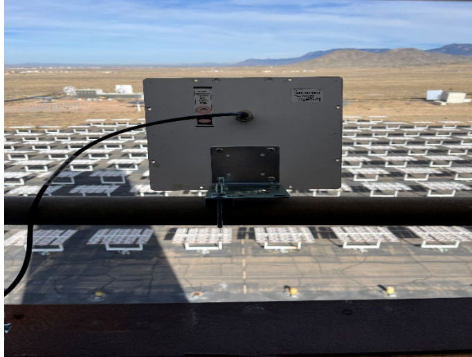
Figure 45. Gateway Antenna Installed at NSTTF 220 Level.
