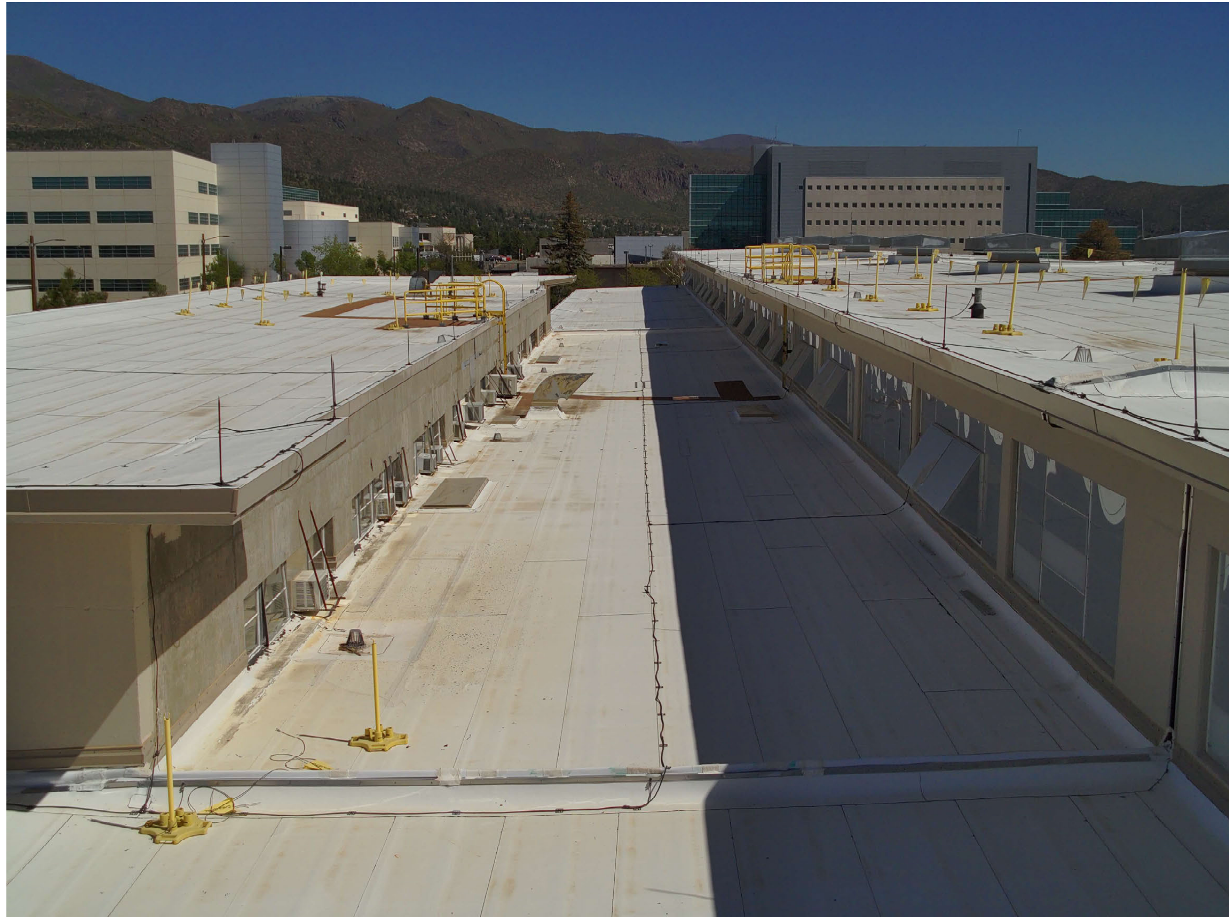
TA-03-0039 admin wing on left, spine on right facing north
