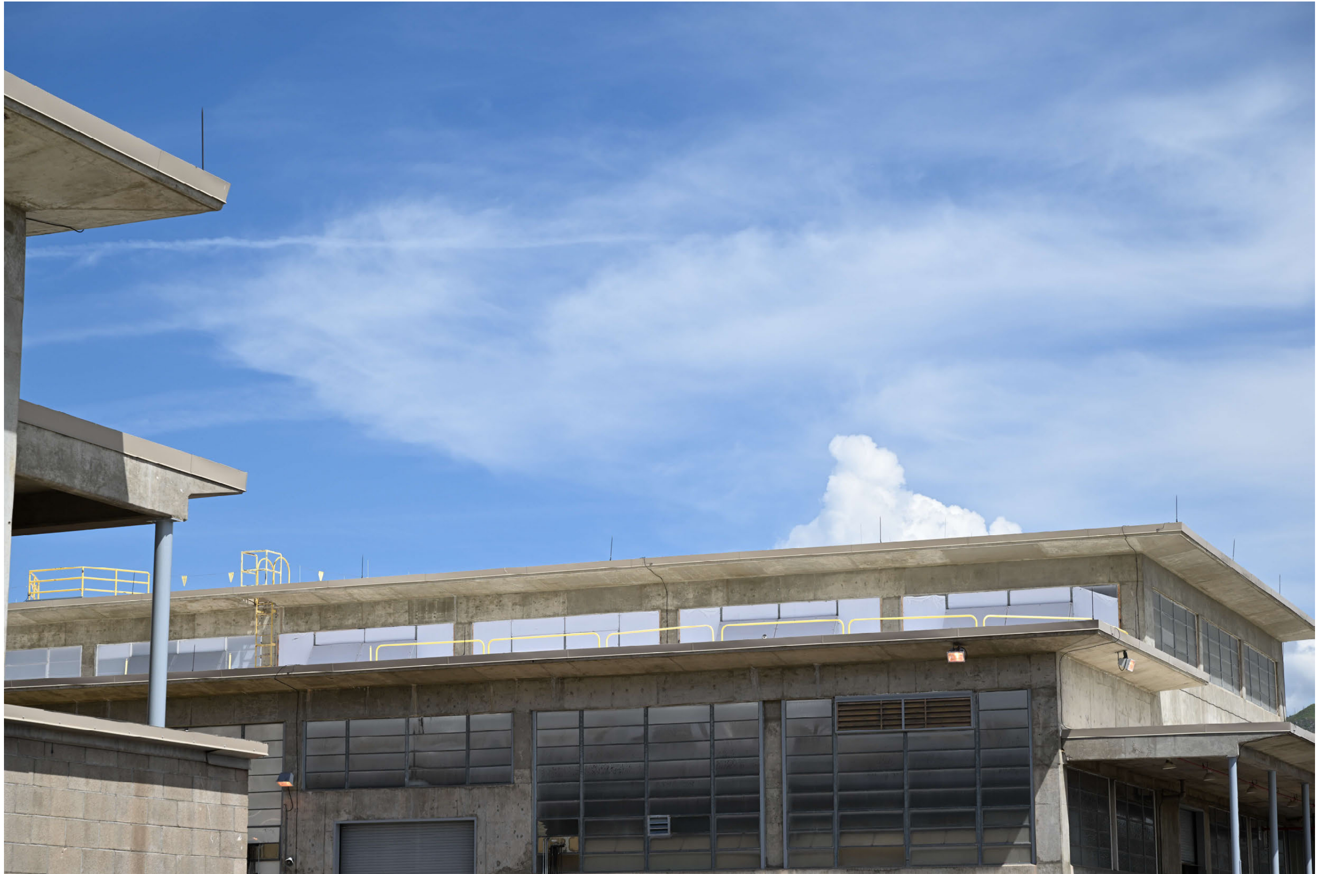
TA-03-0039 center wing, south facade
