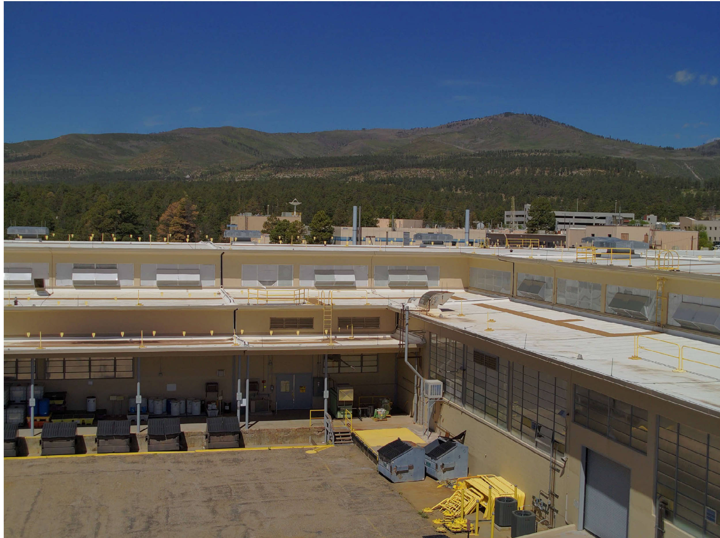
TA-03-0039 south portion of spine (left), center wing (right), east and south facades
