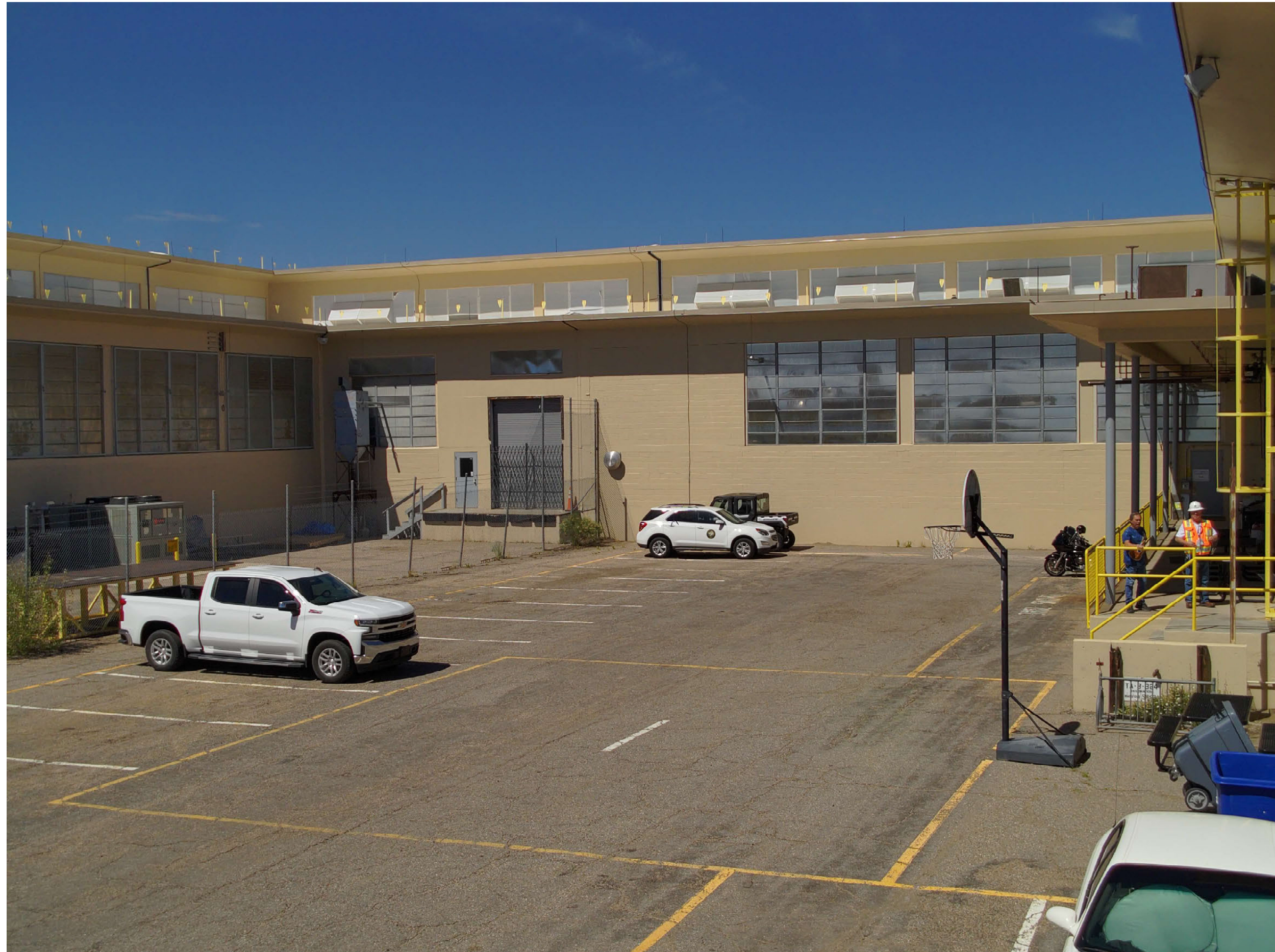
TA-03-0039 north portion of spine, east facade
