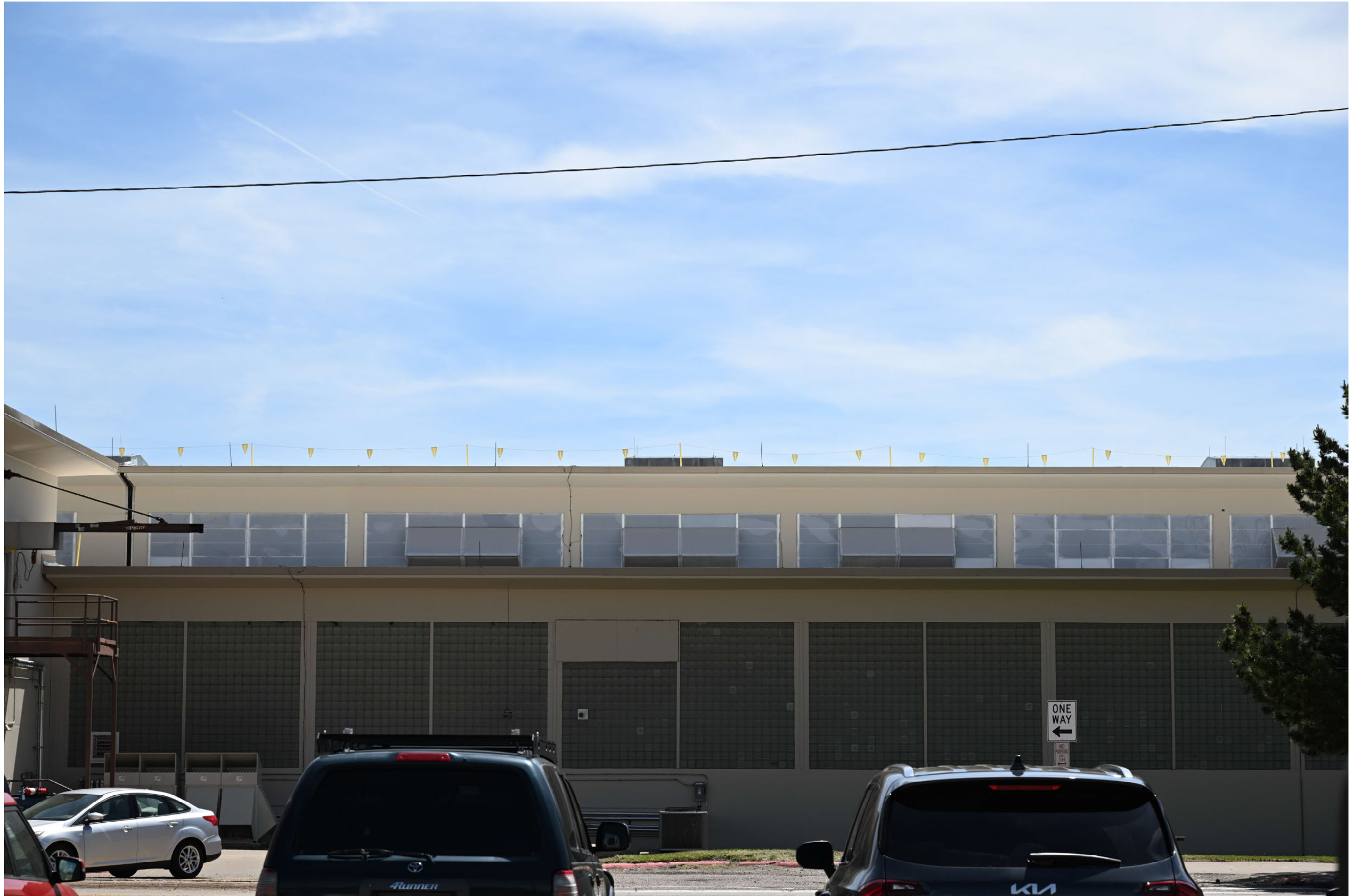
TA-03-0039 south portion of spine, west facade
