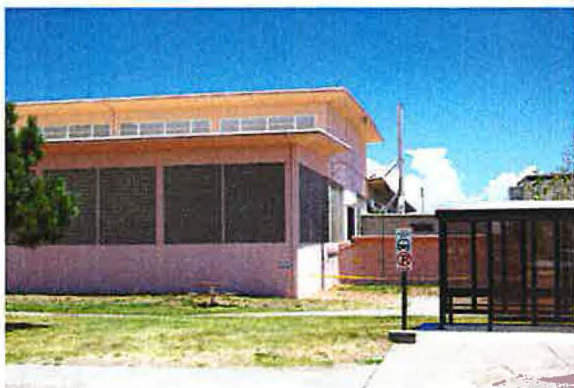
Figure 3: Oblique view of west and south elevations with corridor connecting TA-3-39 to TA-3-102.
