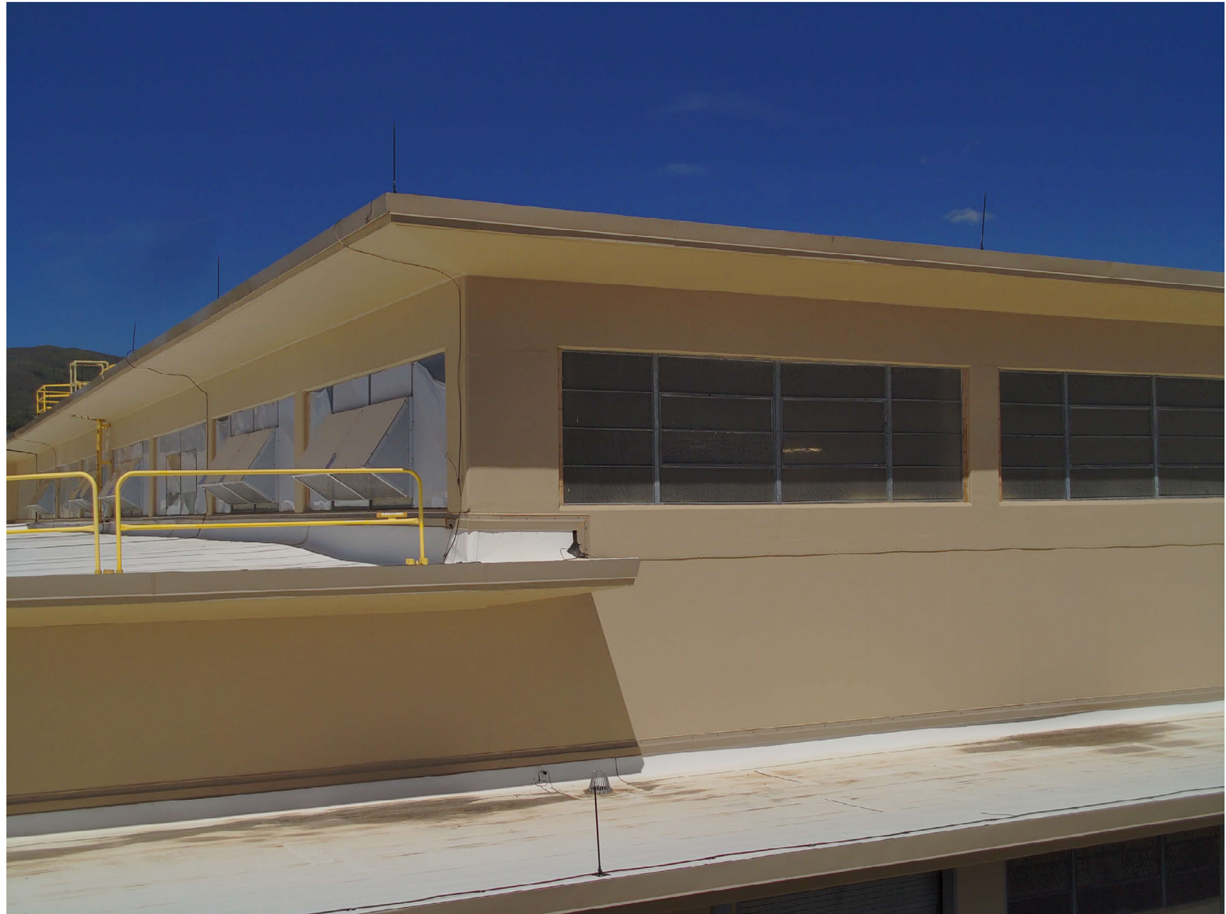
TA-03-0039 center wing, south and east facades
