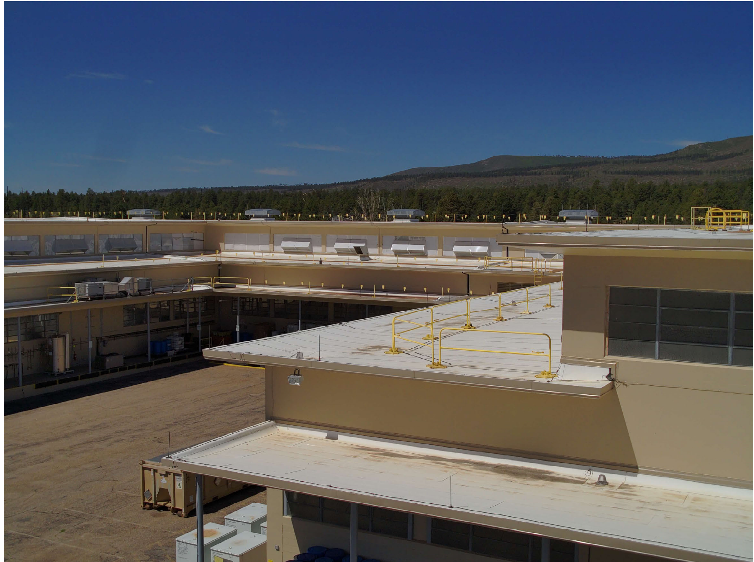
TA-03-0039 south wing (left), south portion of spine (center), center wing (right), north and east facades
