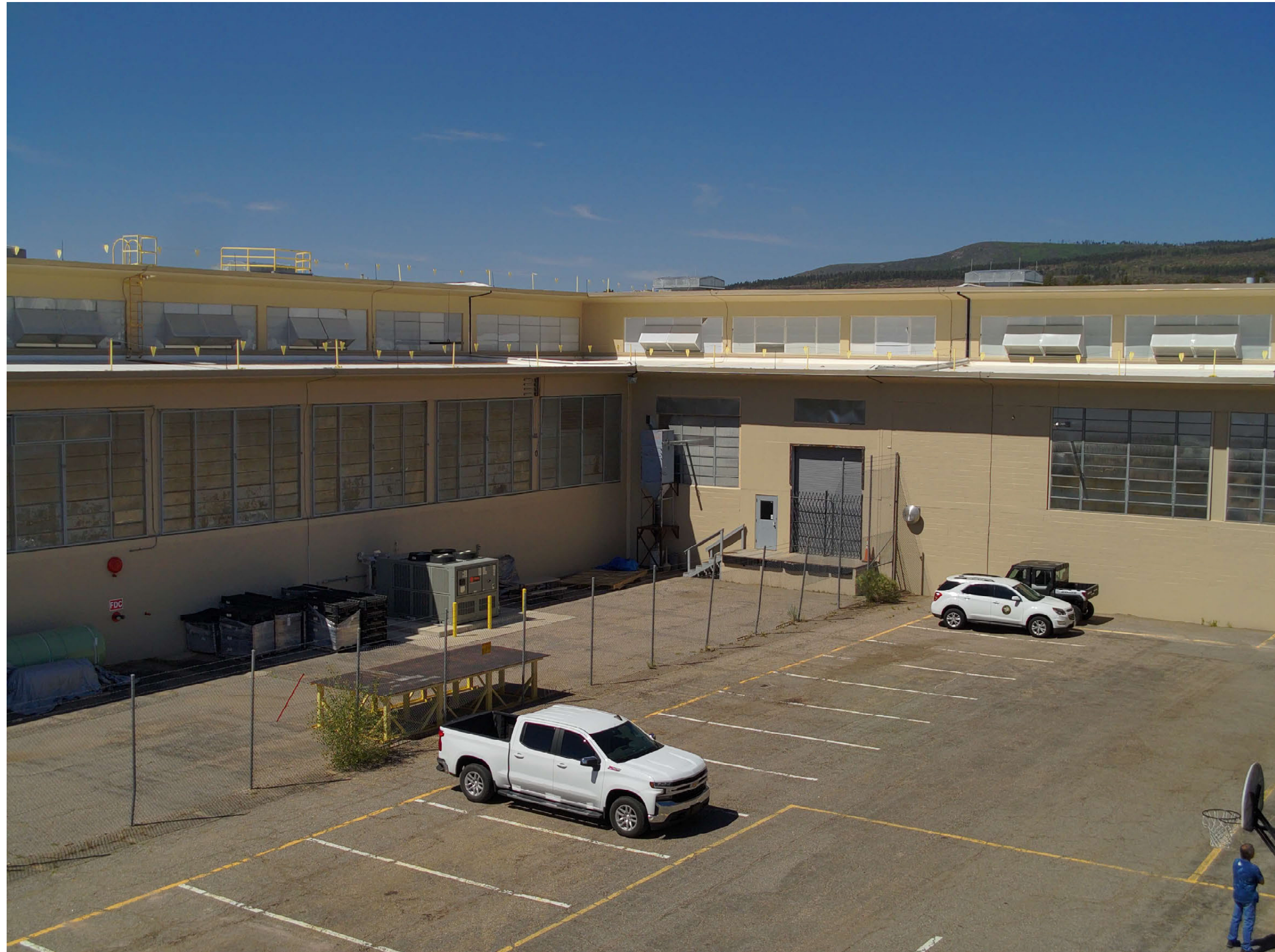
TA-03-0039 center wing and north portion of spine, north and east facades
