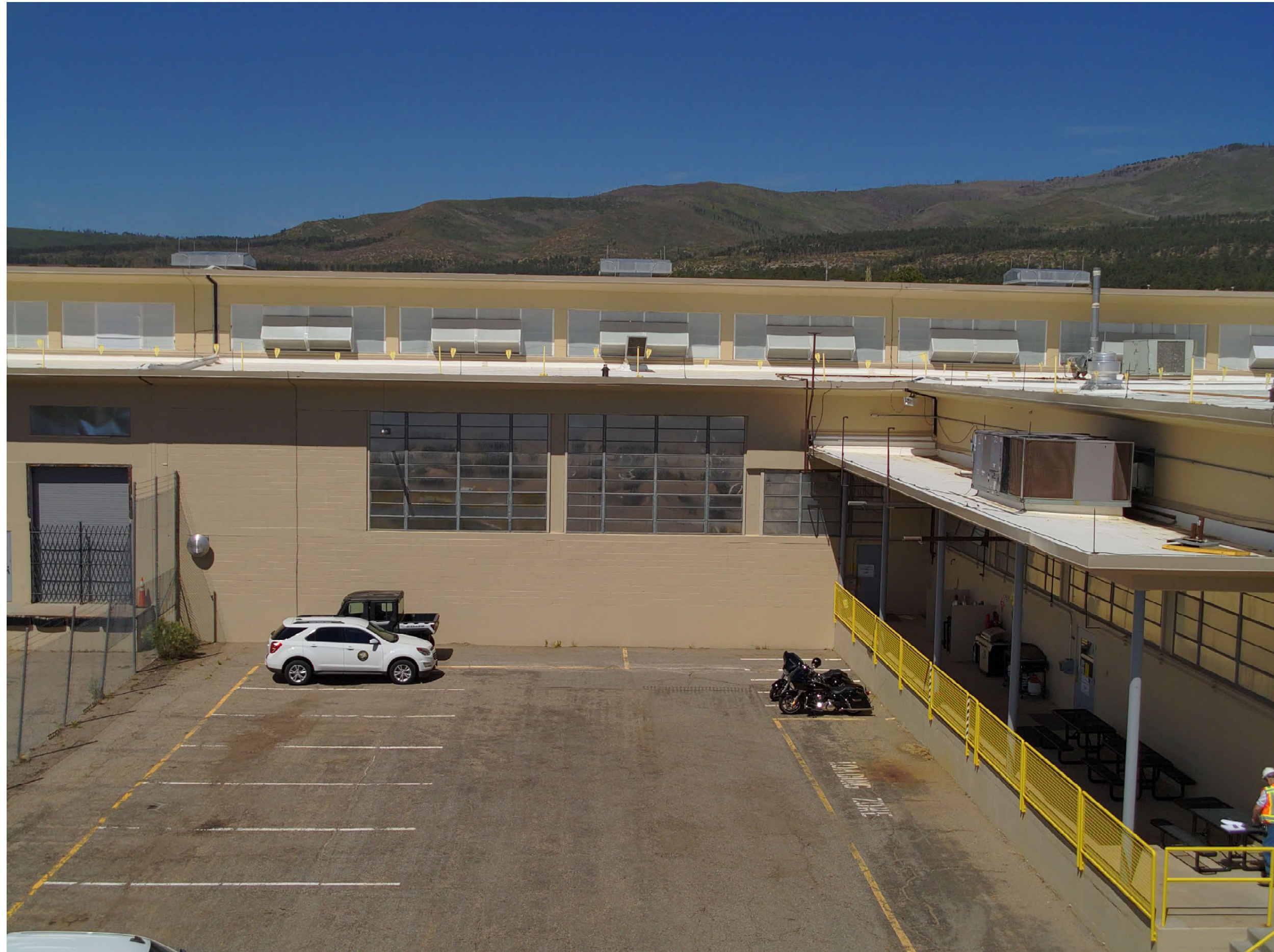
TA-03-0039 north portion of spine (left, center), north wing (right), east and south facades
