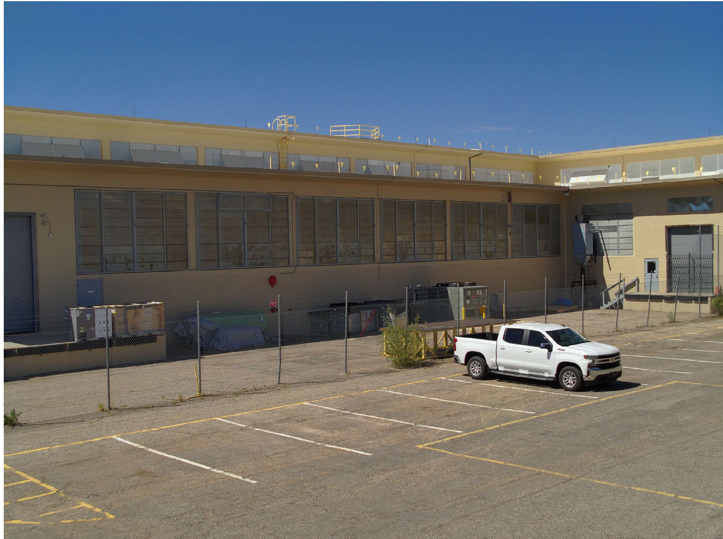
TA-03-0039 center wing, north and east facades
