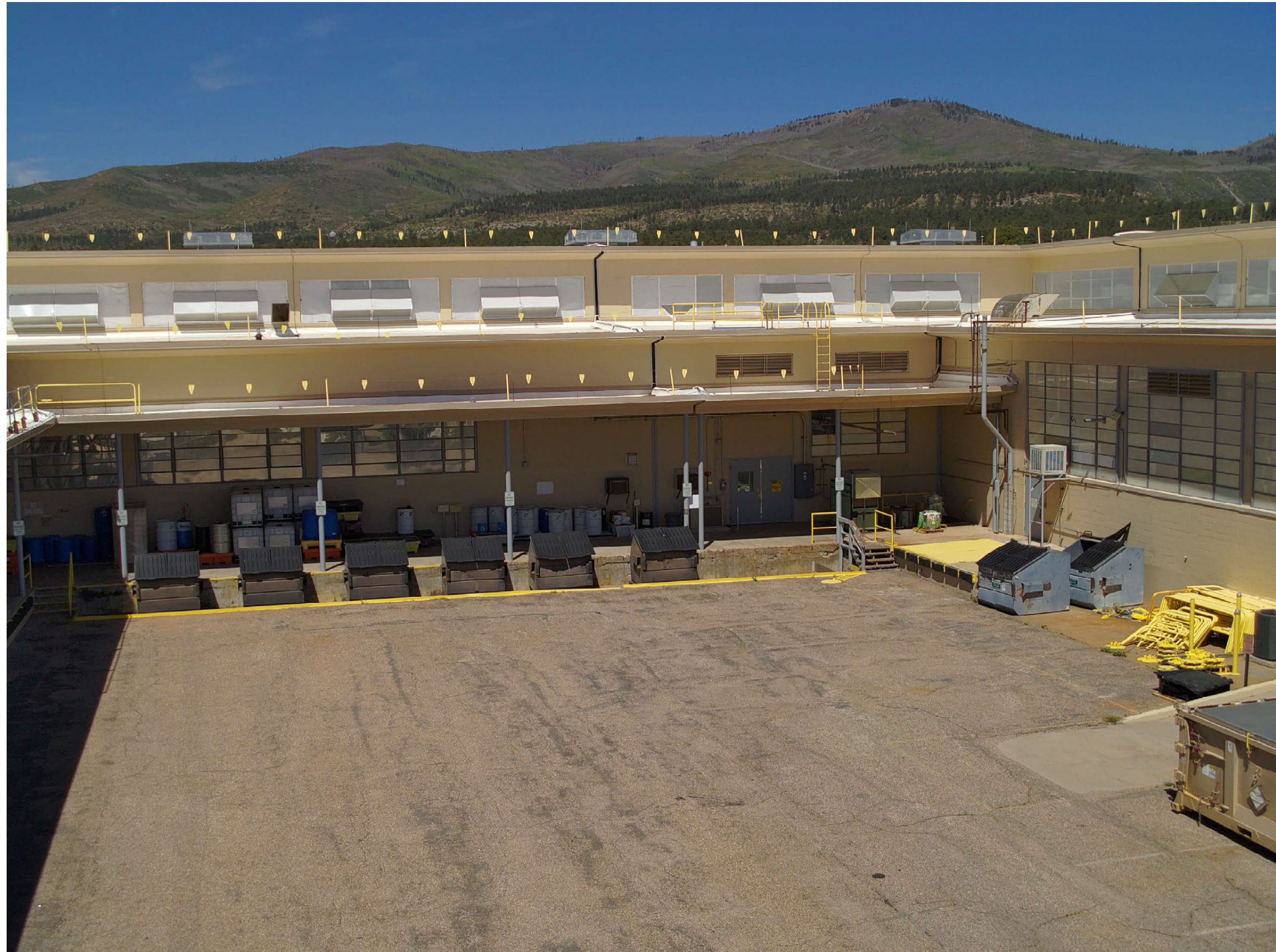
TA-03-0039 south portion of spine, east facade
