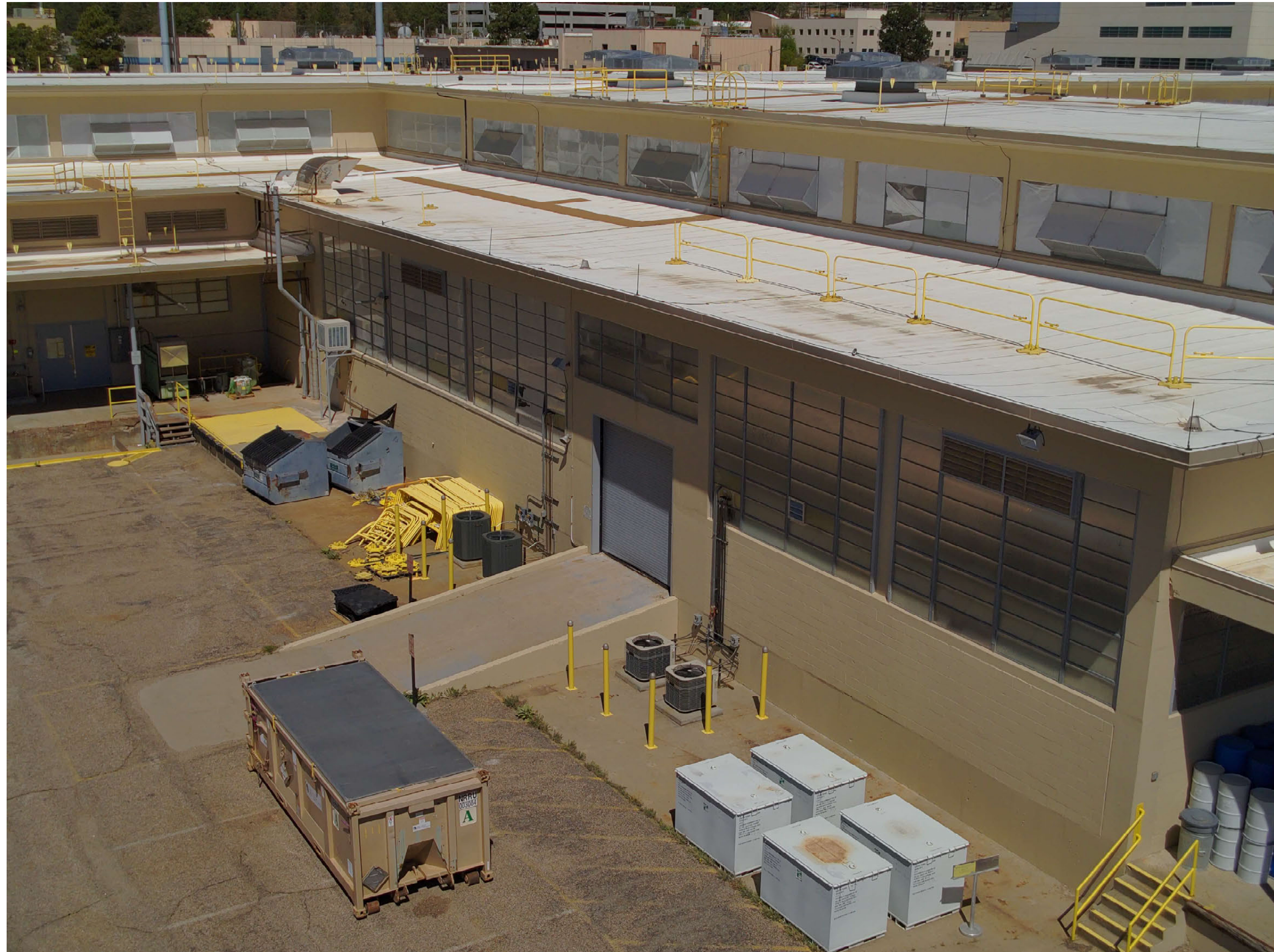
TA-03-0039 center wing, south facade
