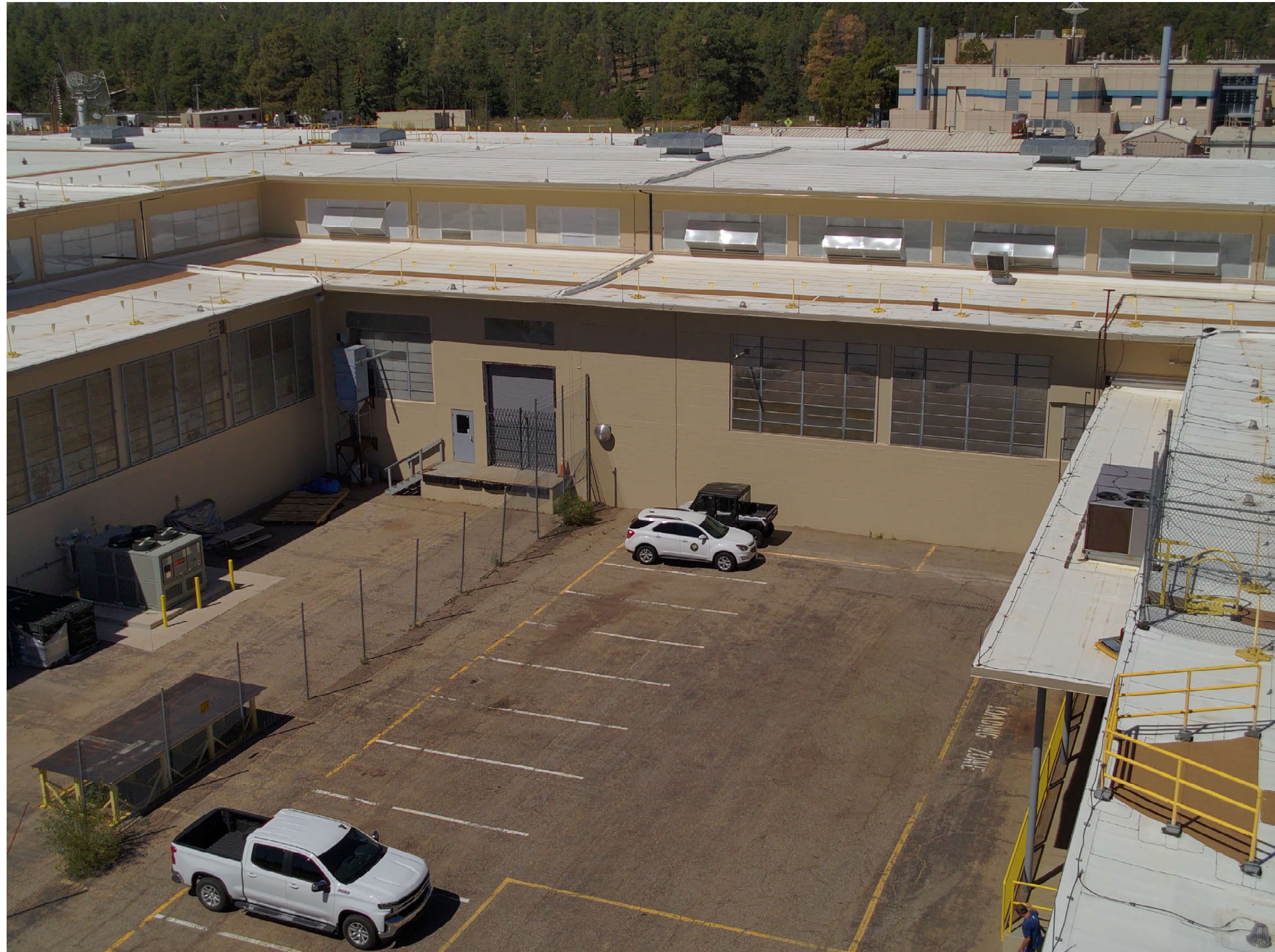
TA-03-0039 north portion of spine, east facade
