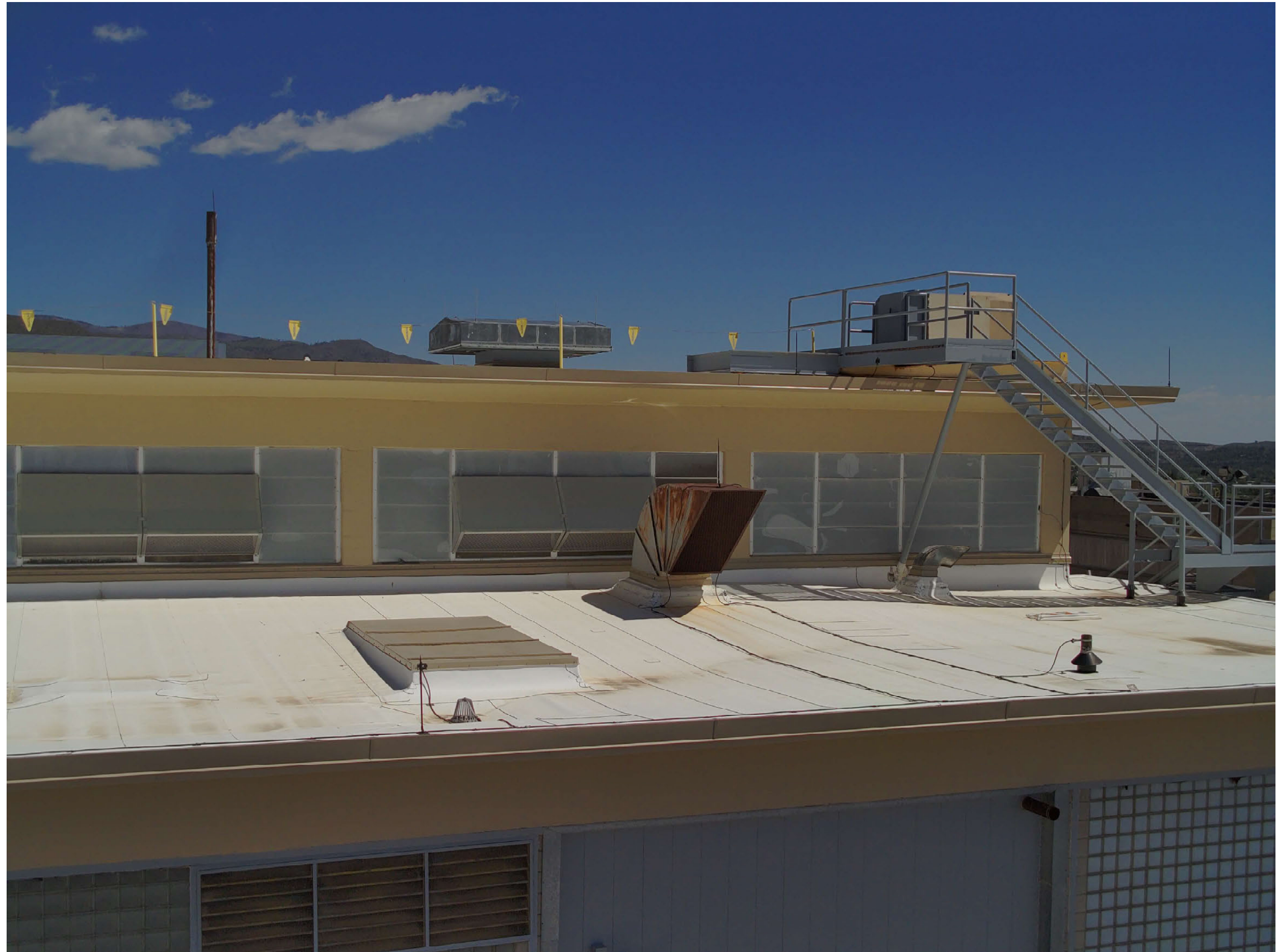
TA-03-0039 south wing, south facade
