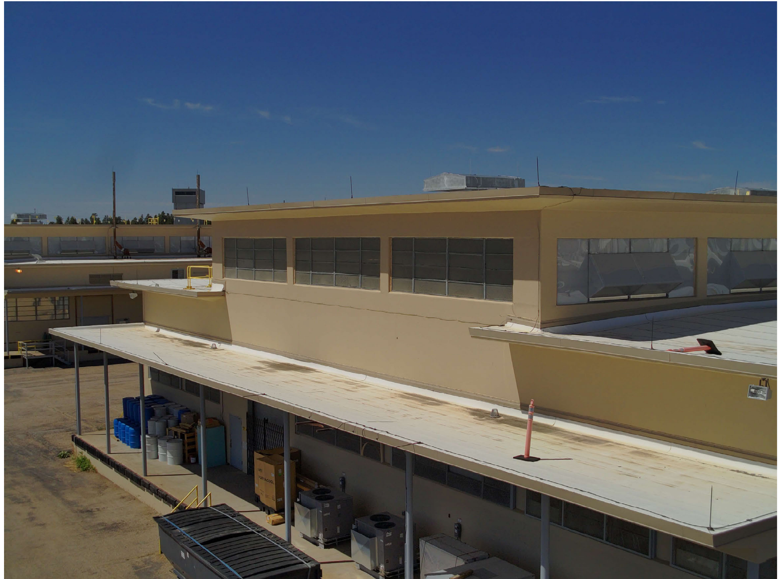
TA-03-0039 center wing (foreground), south wing (background), east facade
