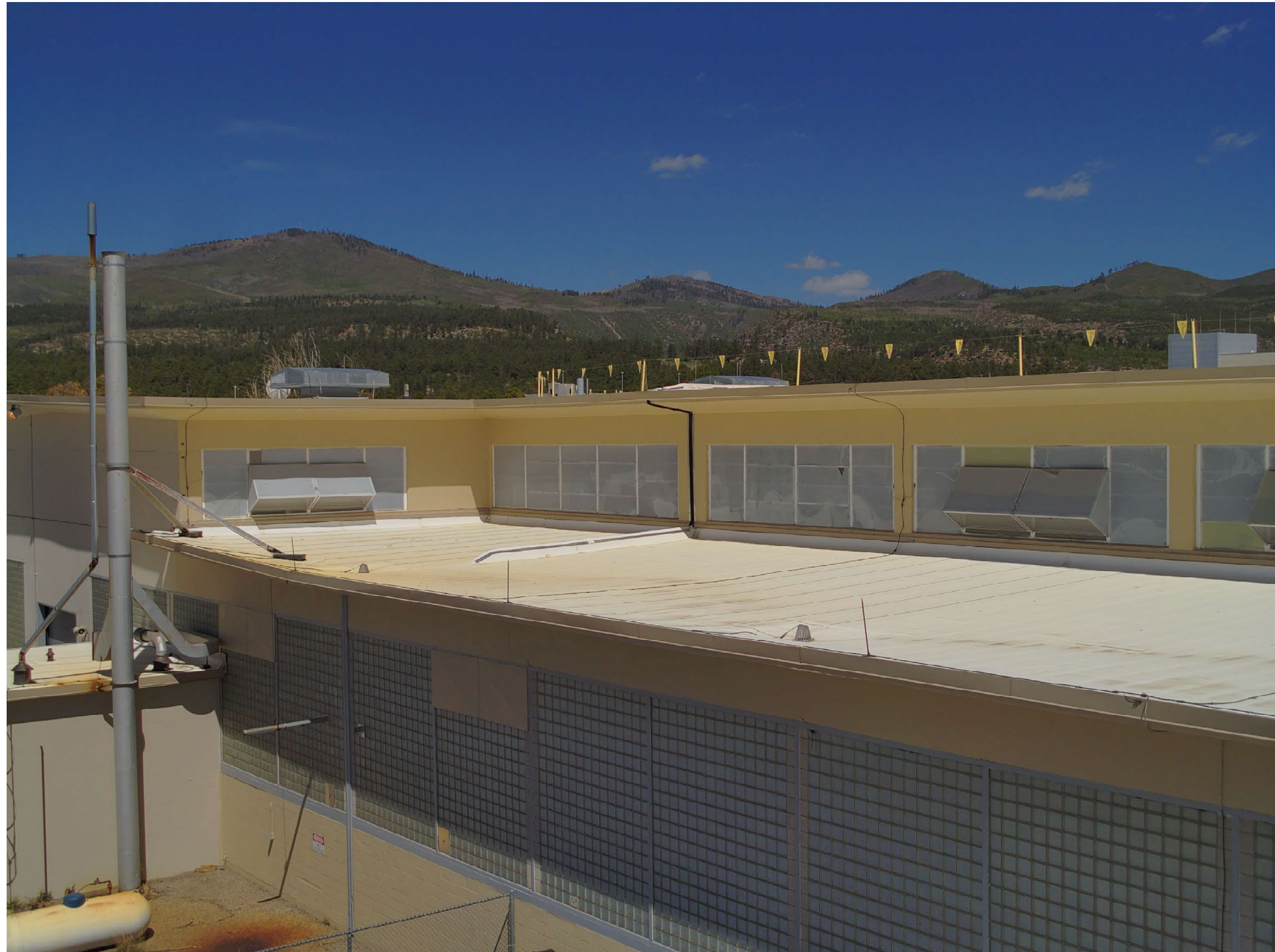
TA-03-0039 south wing, south facade
