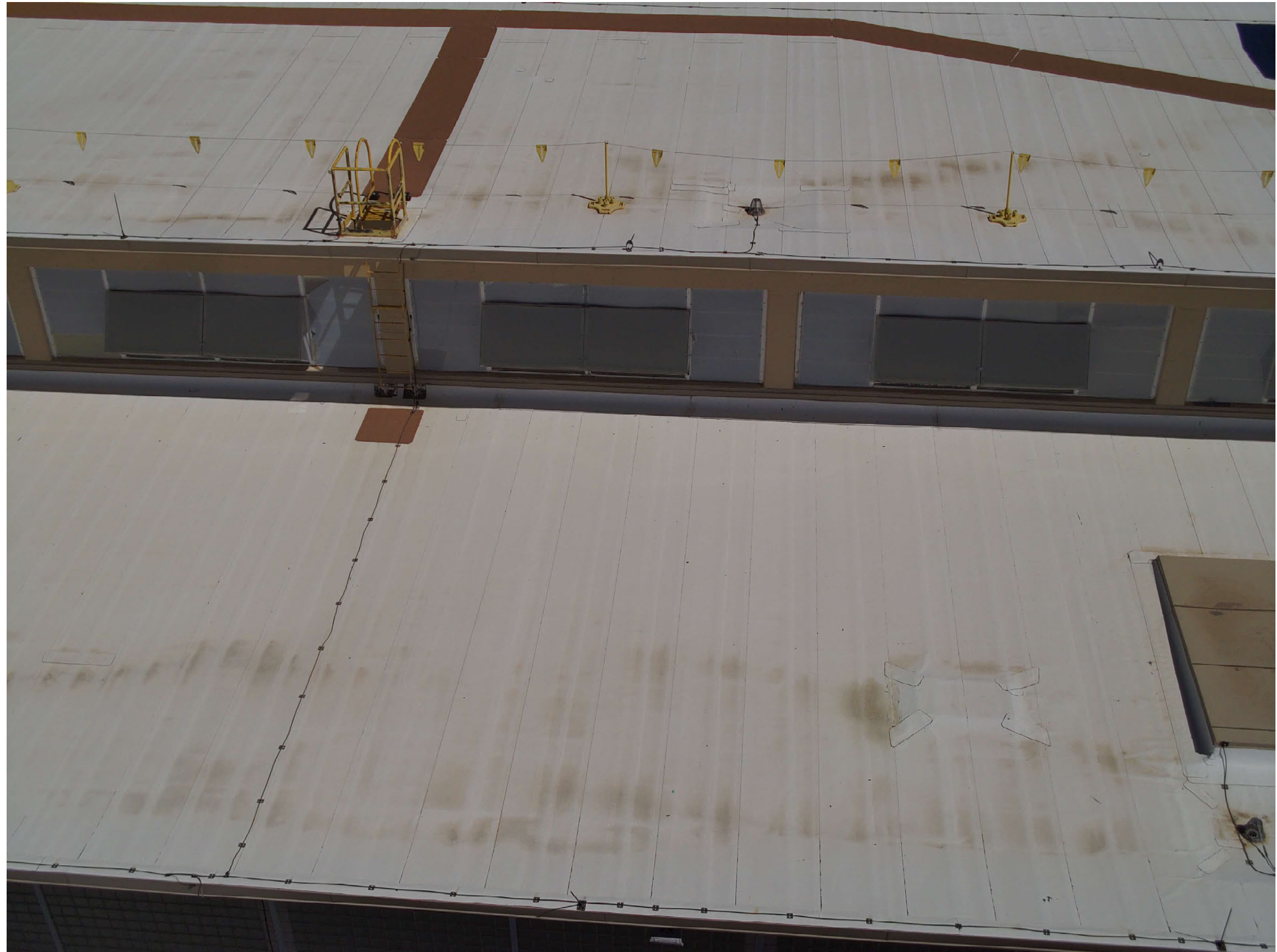
TA-03-0039 south wing clerestory, south facade
