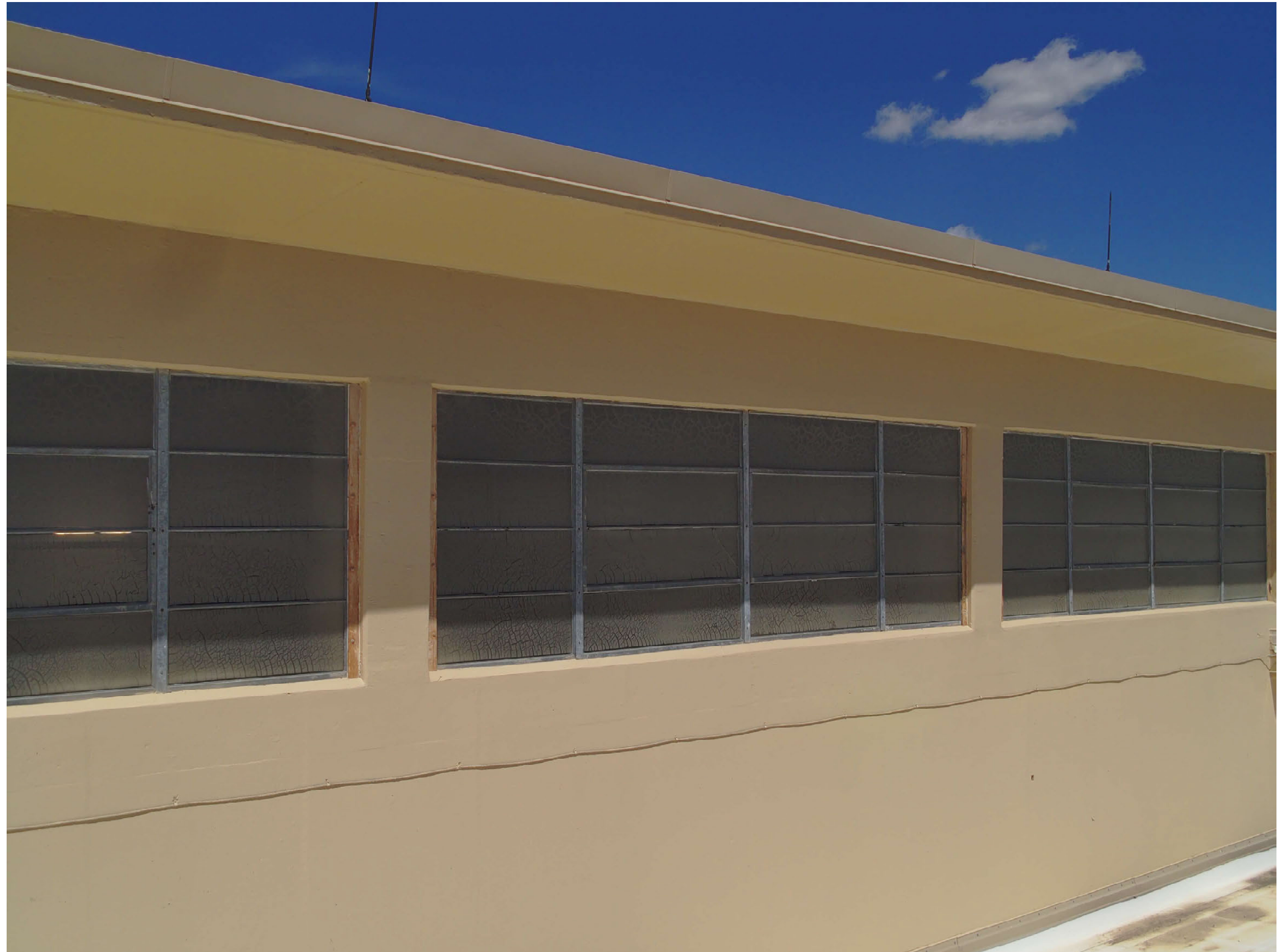
TA-03-0039 center wing, east facade
