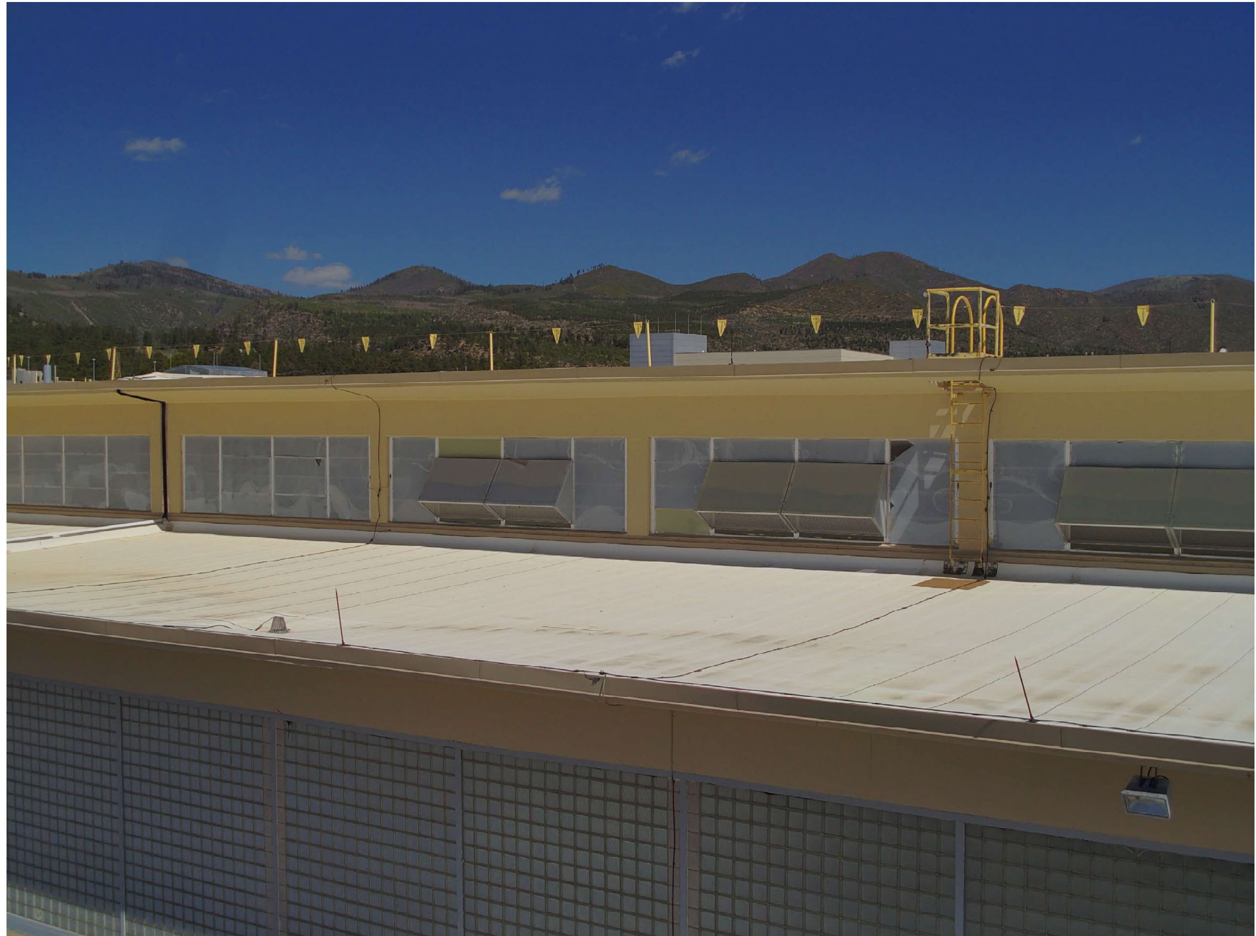
TA-03-0039 south wing, south facade
