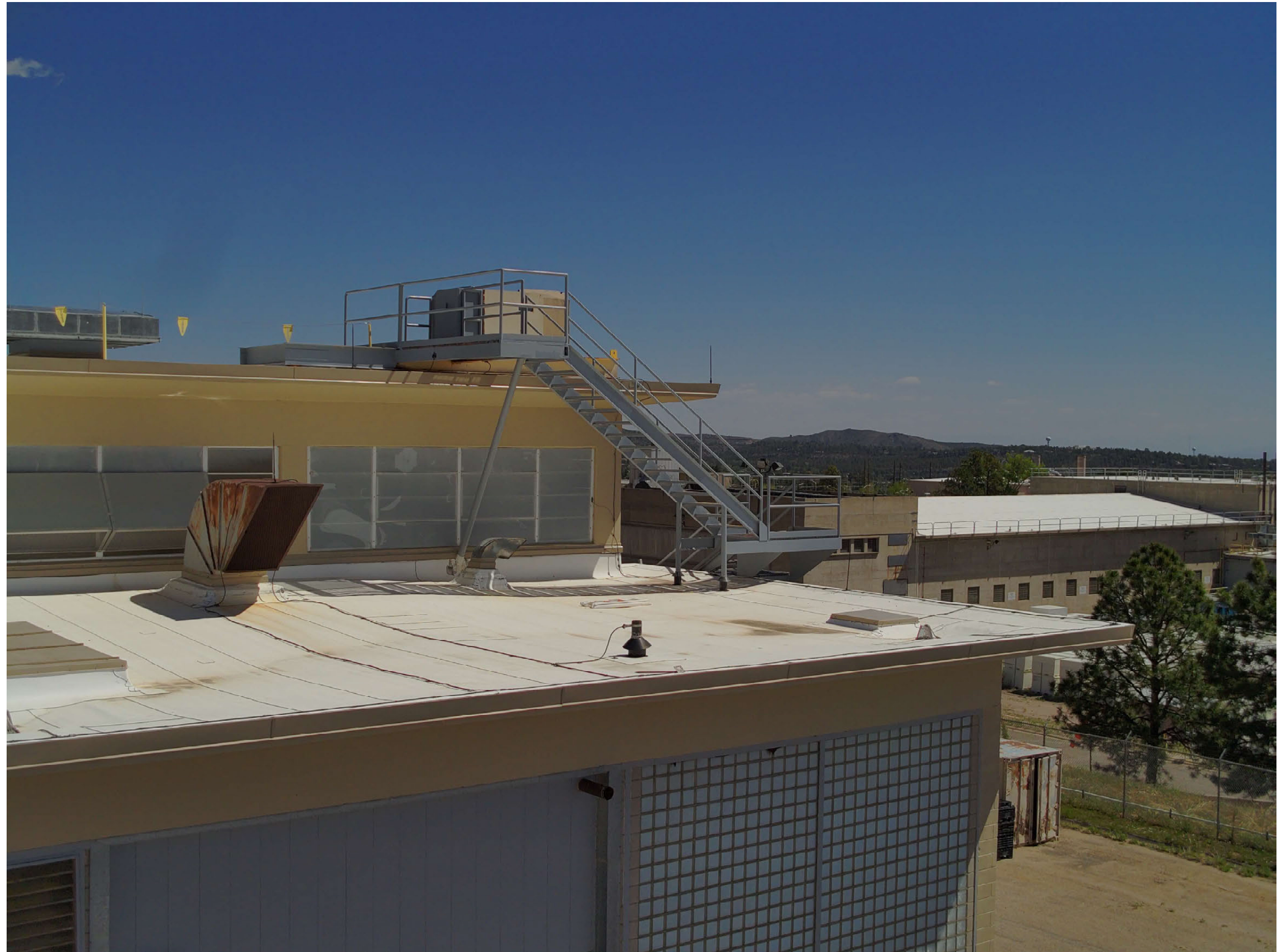
TA-03-0039 south wing, south facade
