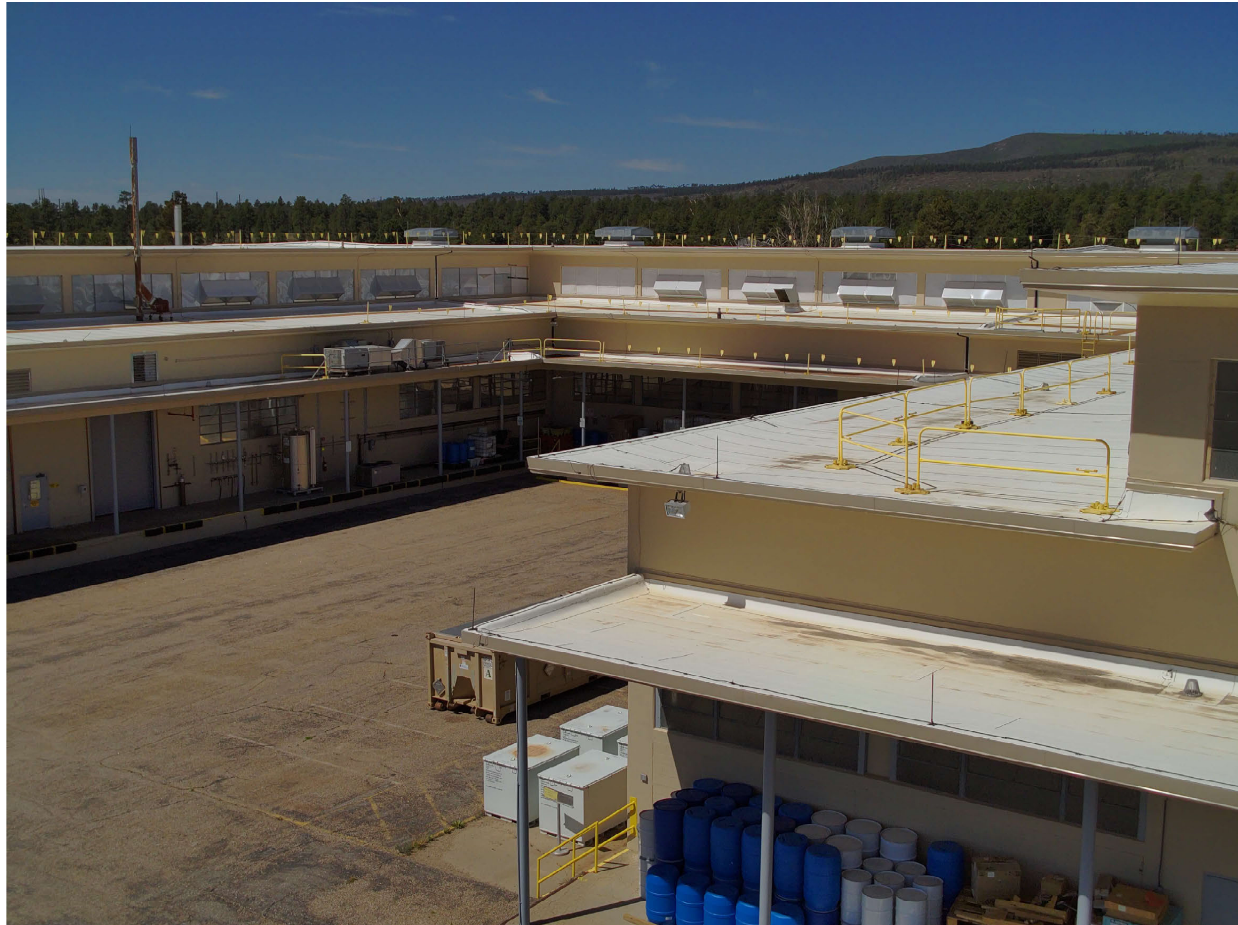
TA-03-0039 south wing (left), south portion of spine (right), north and east facades
