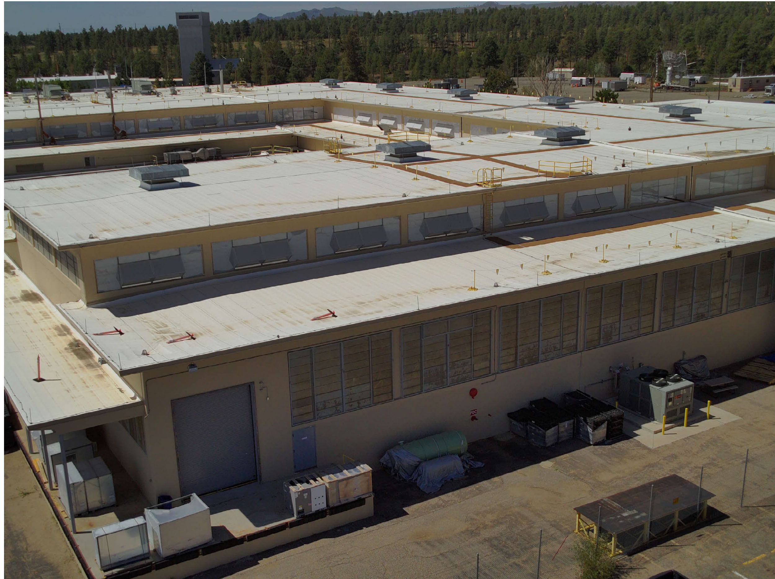
TA-03-0039 center and south wings, north facades
