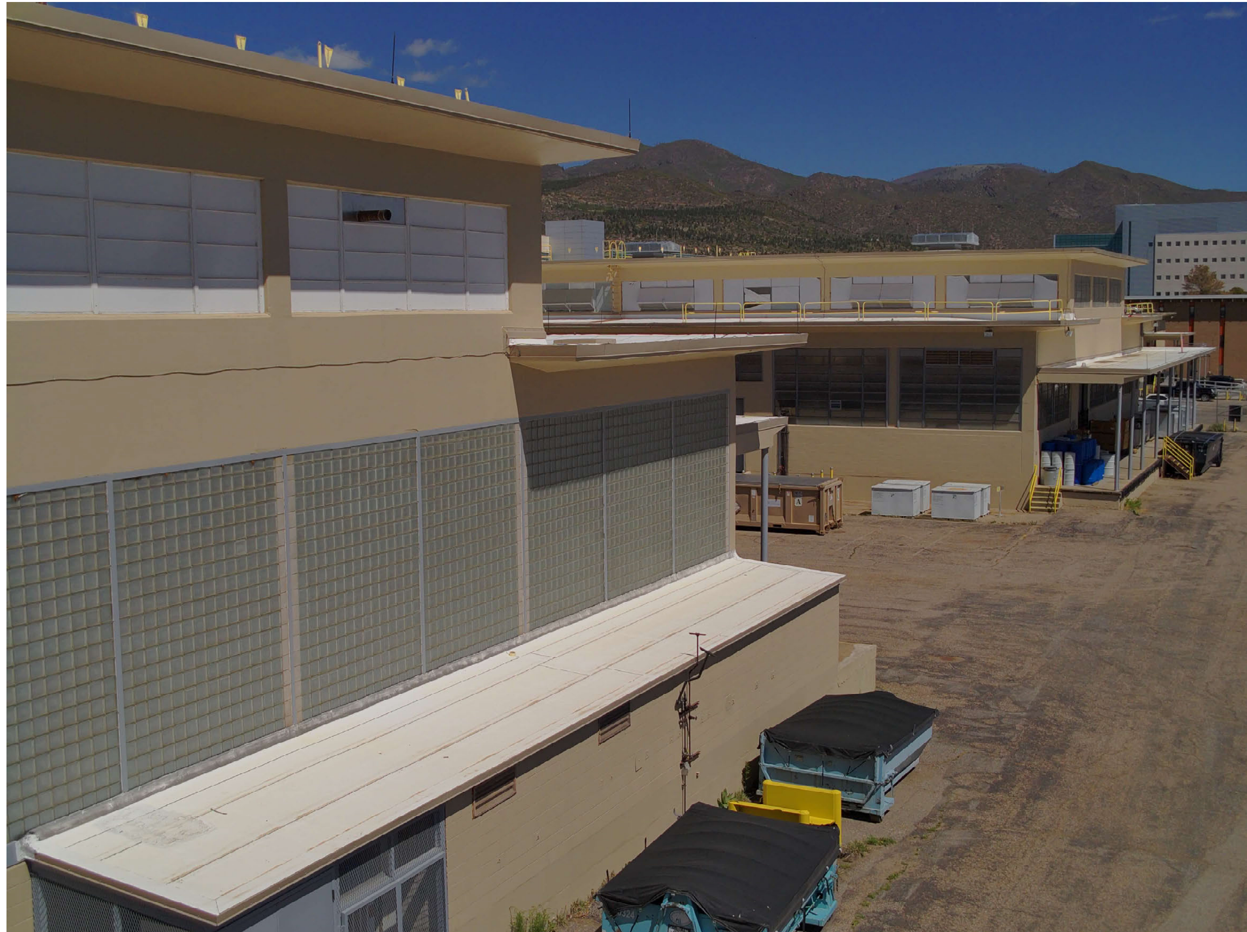
TA-03-0039 south wing (foreground), center wing (background), south and east facades
