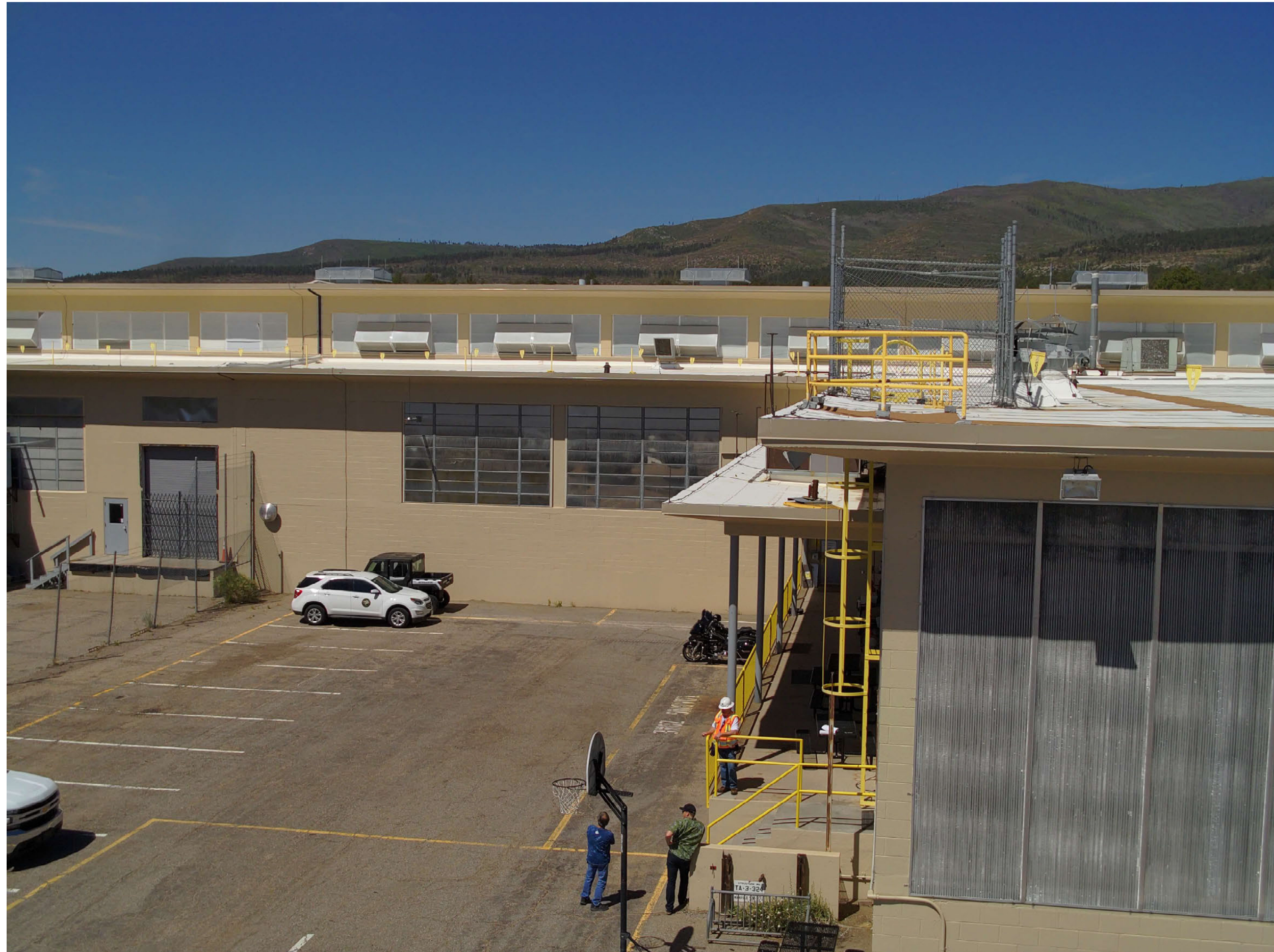
TA-03-0039 north portion of spine, east facade
