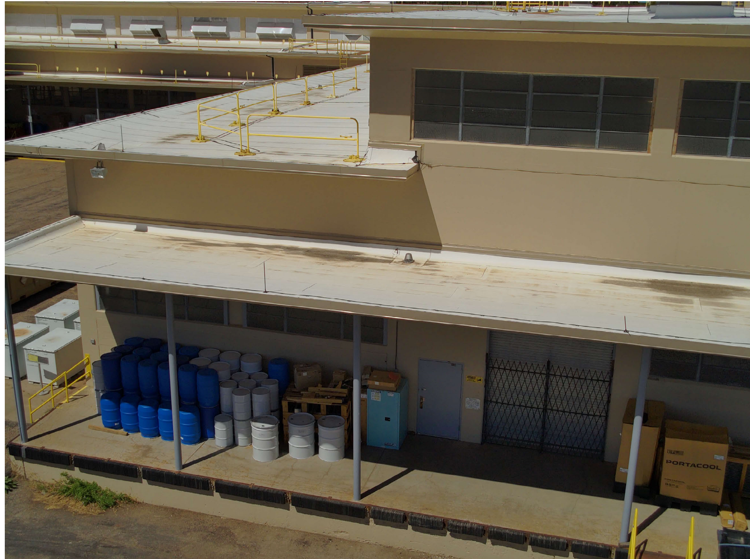
TA-03-0039 south portion of spine (left), center wing (right), east facades
