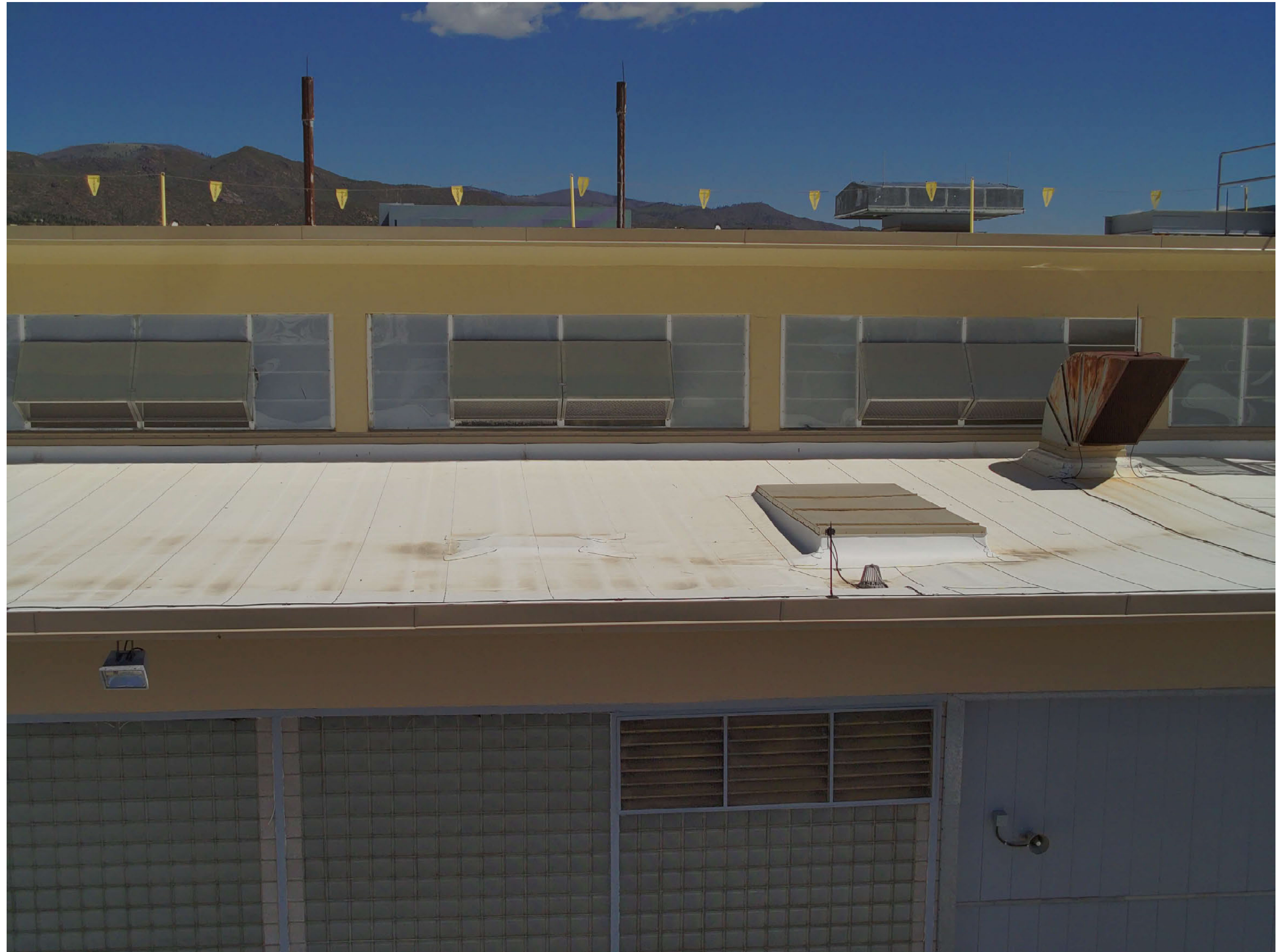
TA-03-0039 south wing, south facade
