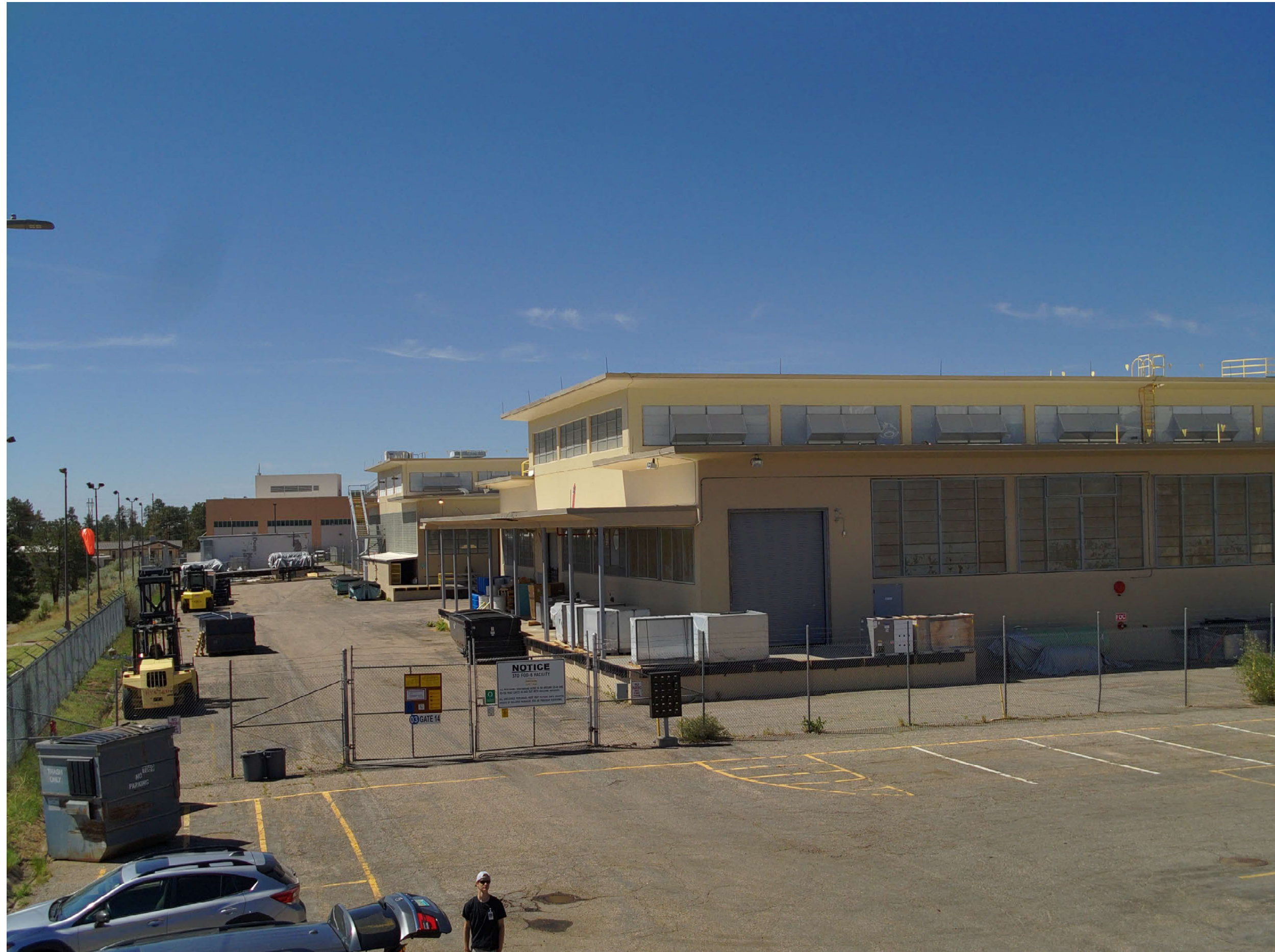
TA-03-0039 center wing (foreground) and south wing (background), north facades
