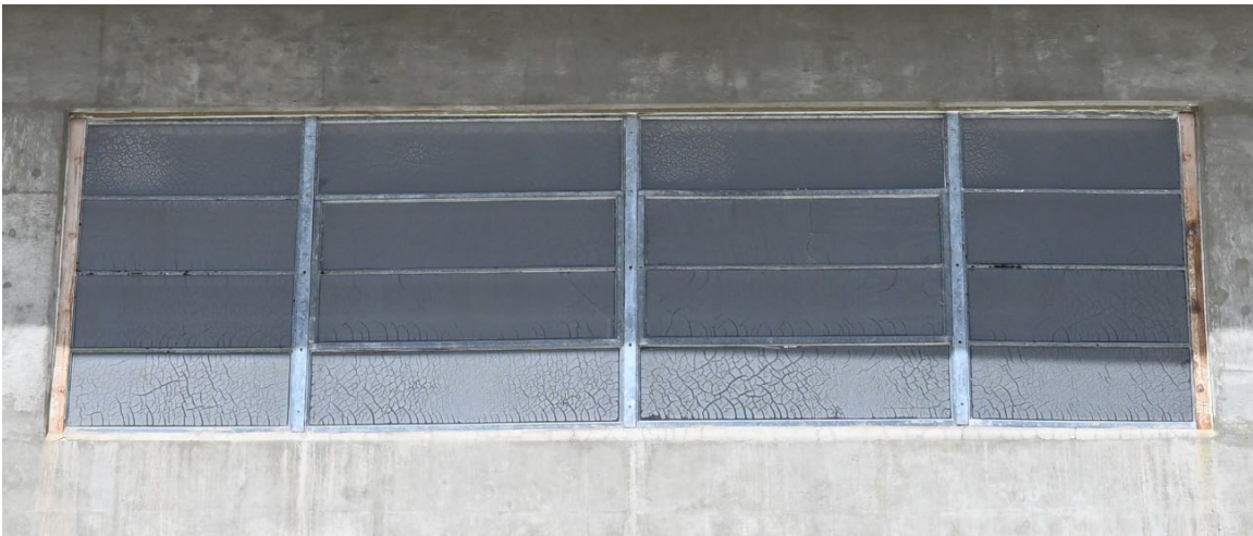
Figure 5-5. Example deteriorated window film coating (center) June 6, 2023 (LANL image, image no. DSC_0112).
