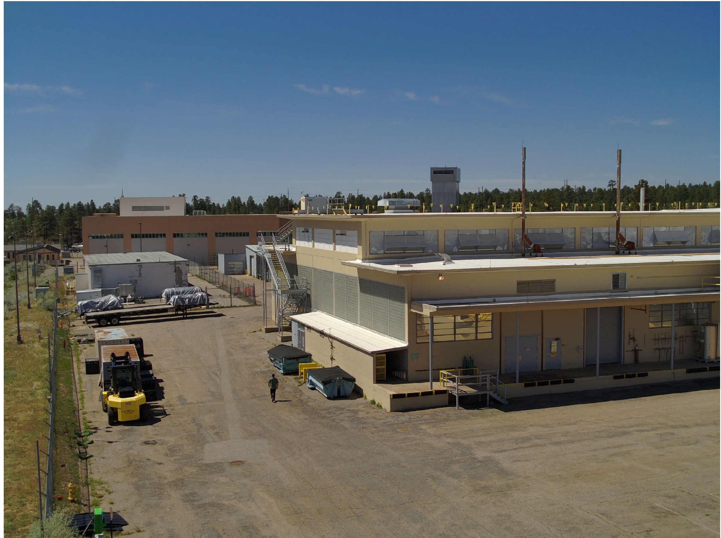
TA-03-0039 south wing, north facade
