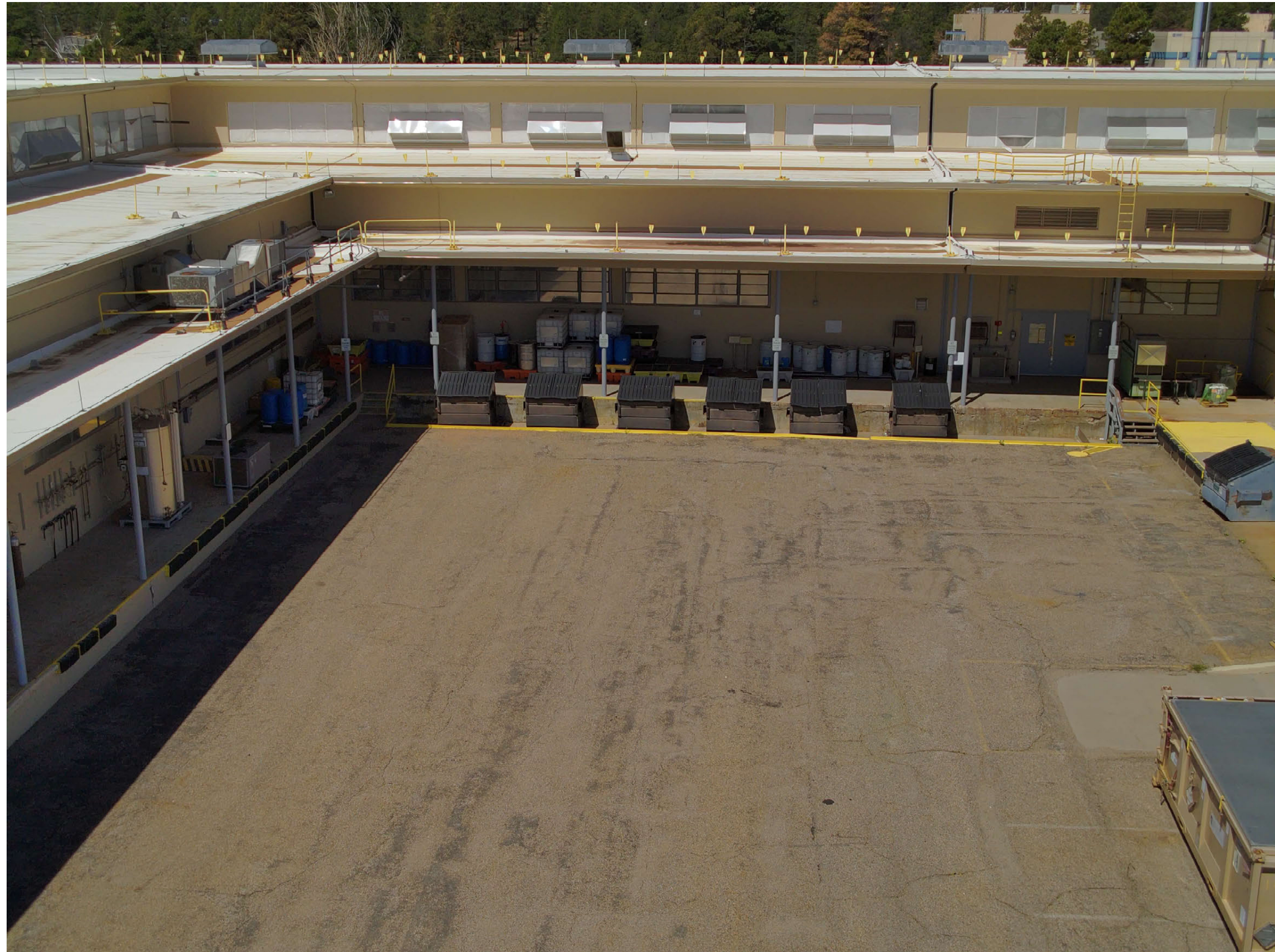
TA-03-0039 south portion of spine, east facade
