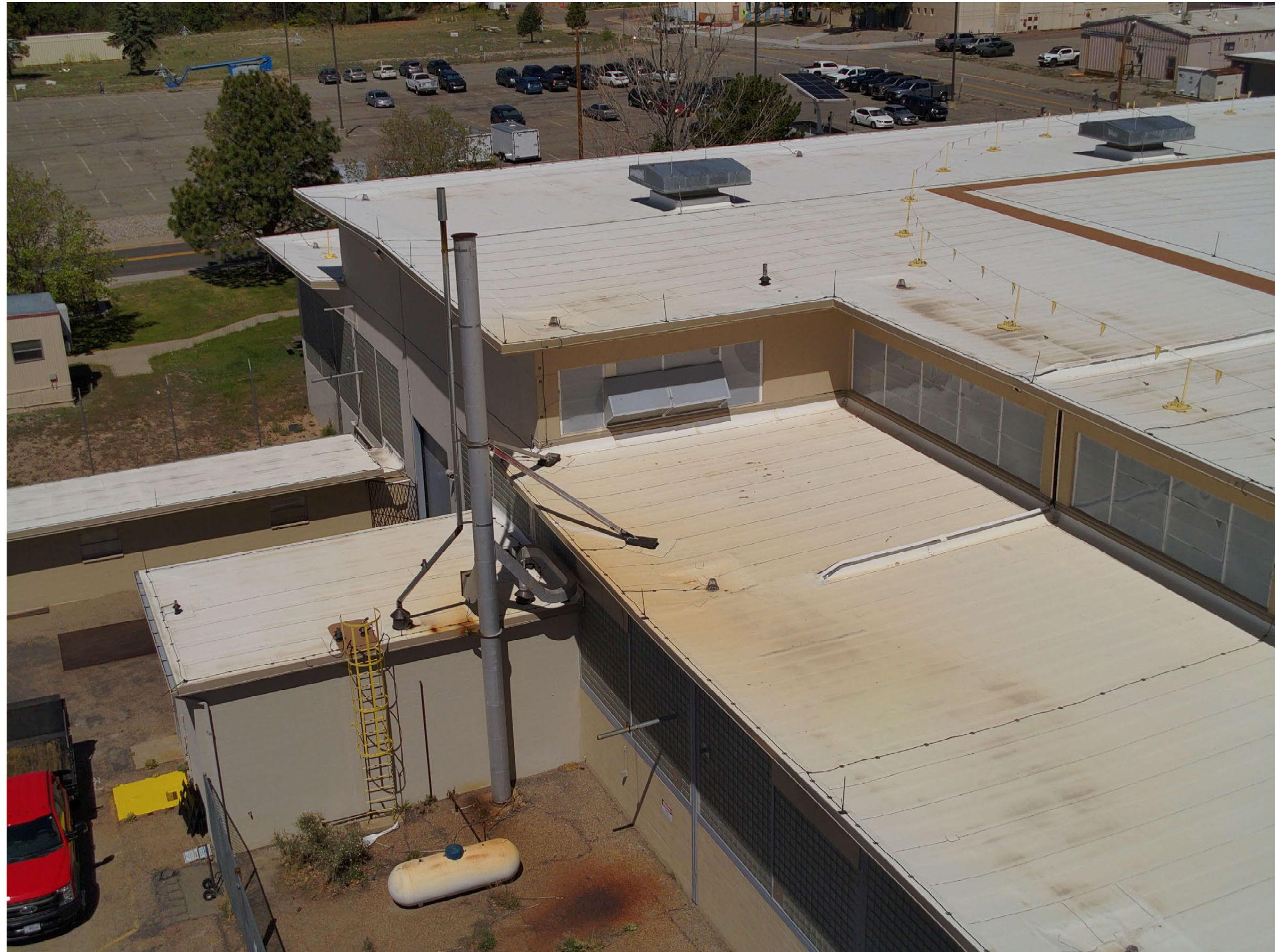
TA-03-0039 south wing, south and east facades
