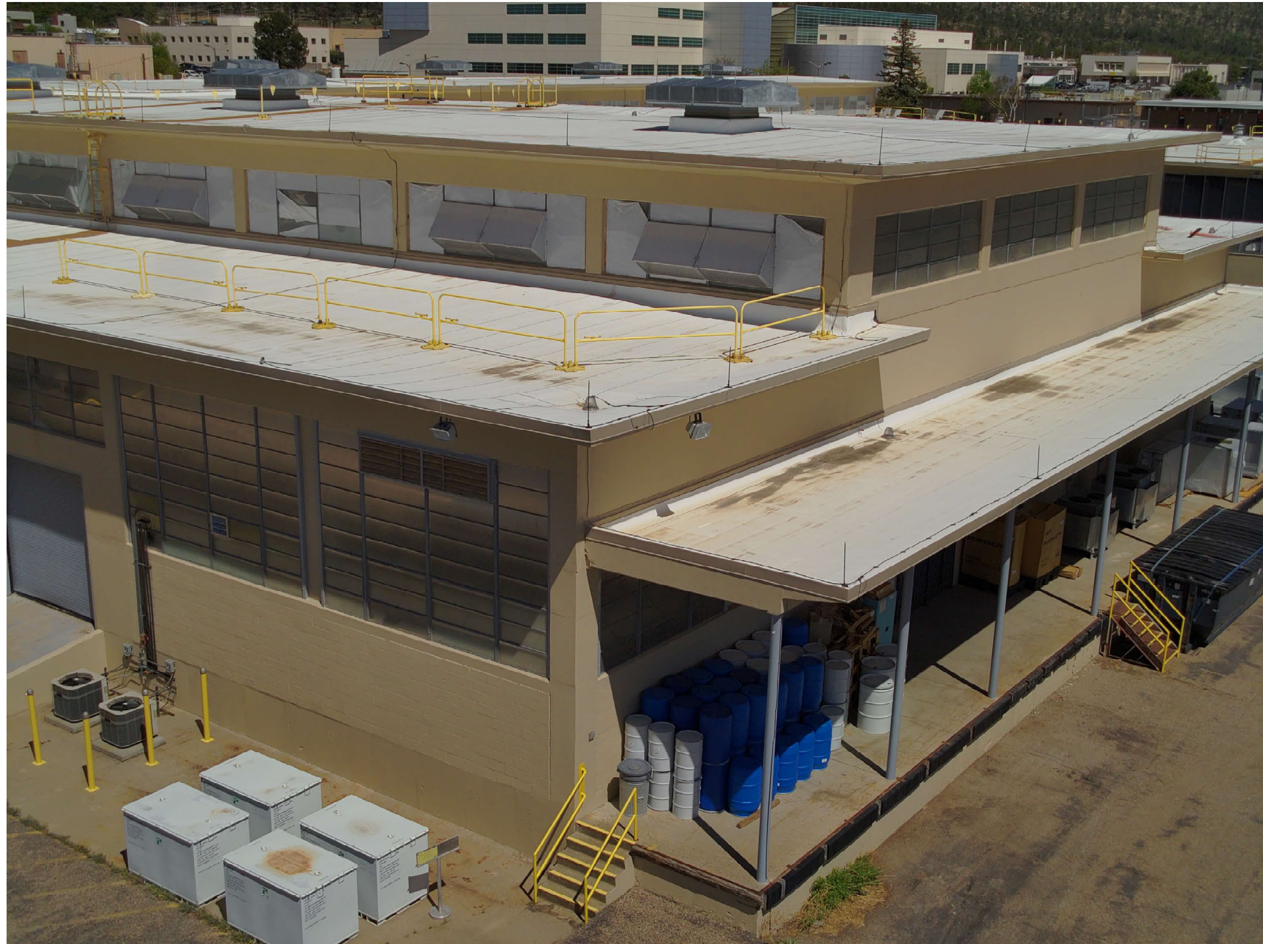
TA-03-0039 center wing, south and east facades
