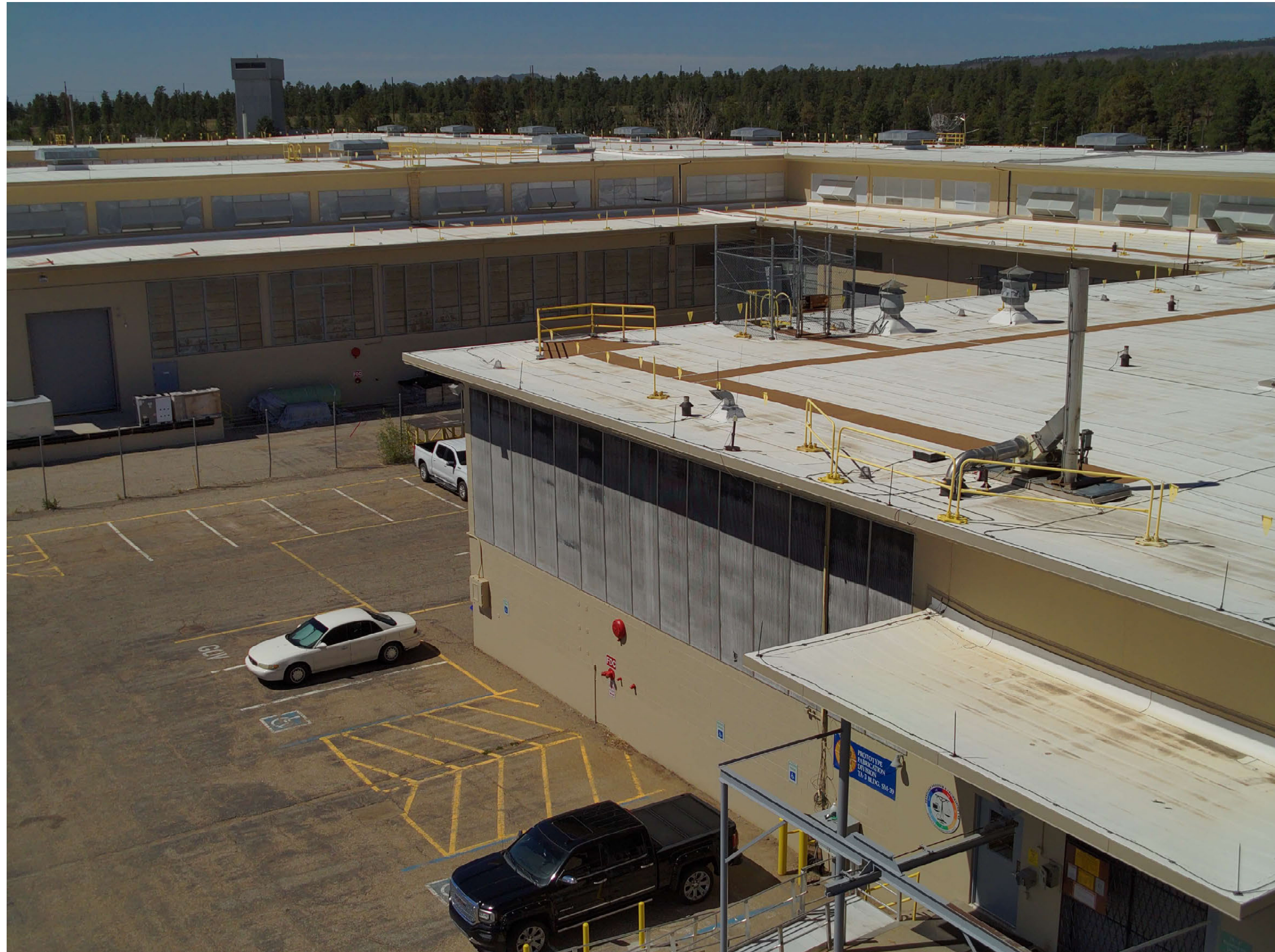
TA-03-0039 north wing (foreground) and center wing (background), north and east facades
