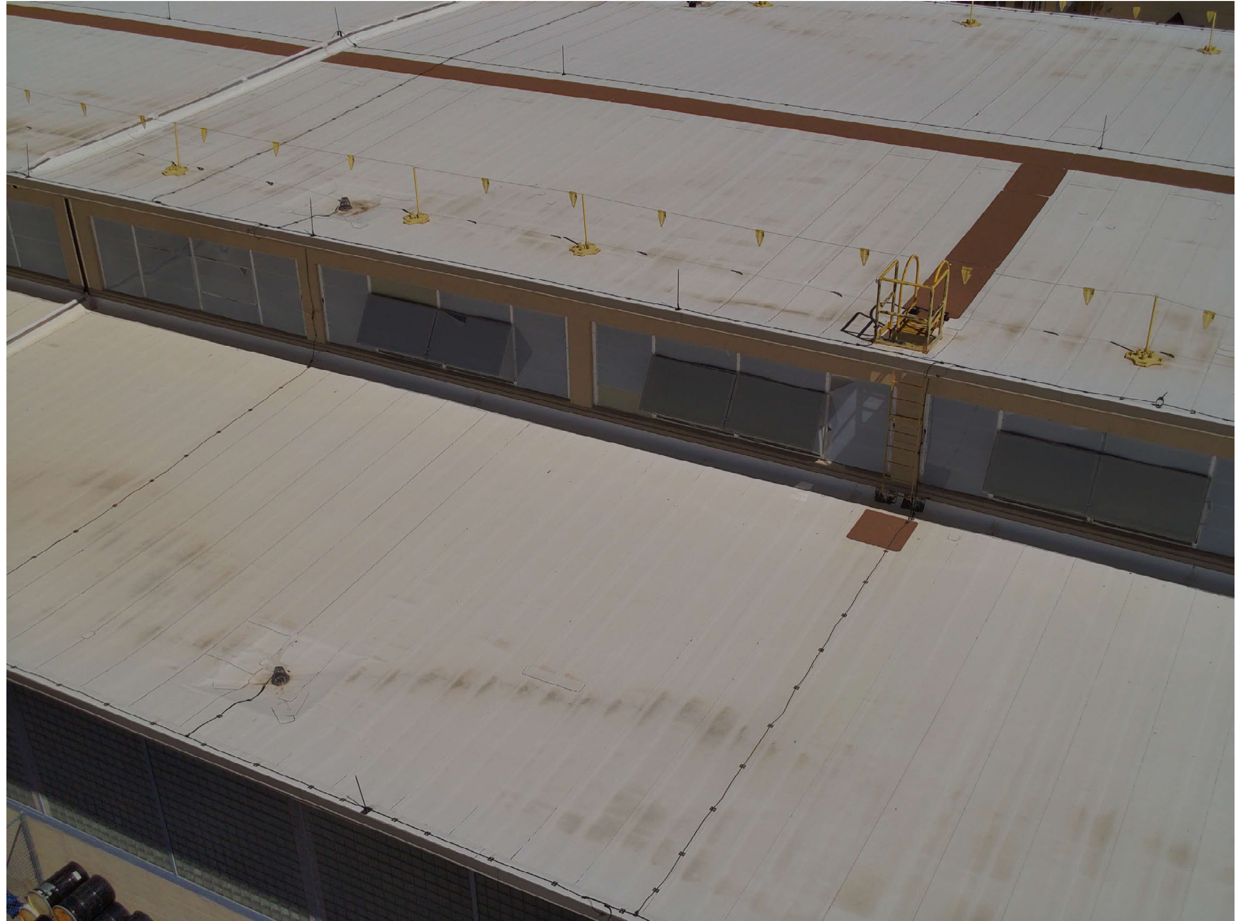
TA-03-0039 south wing clerestory, south facade
