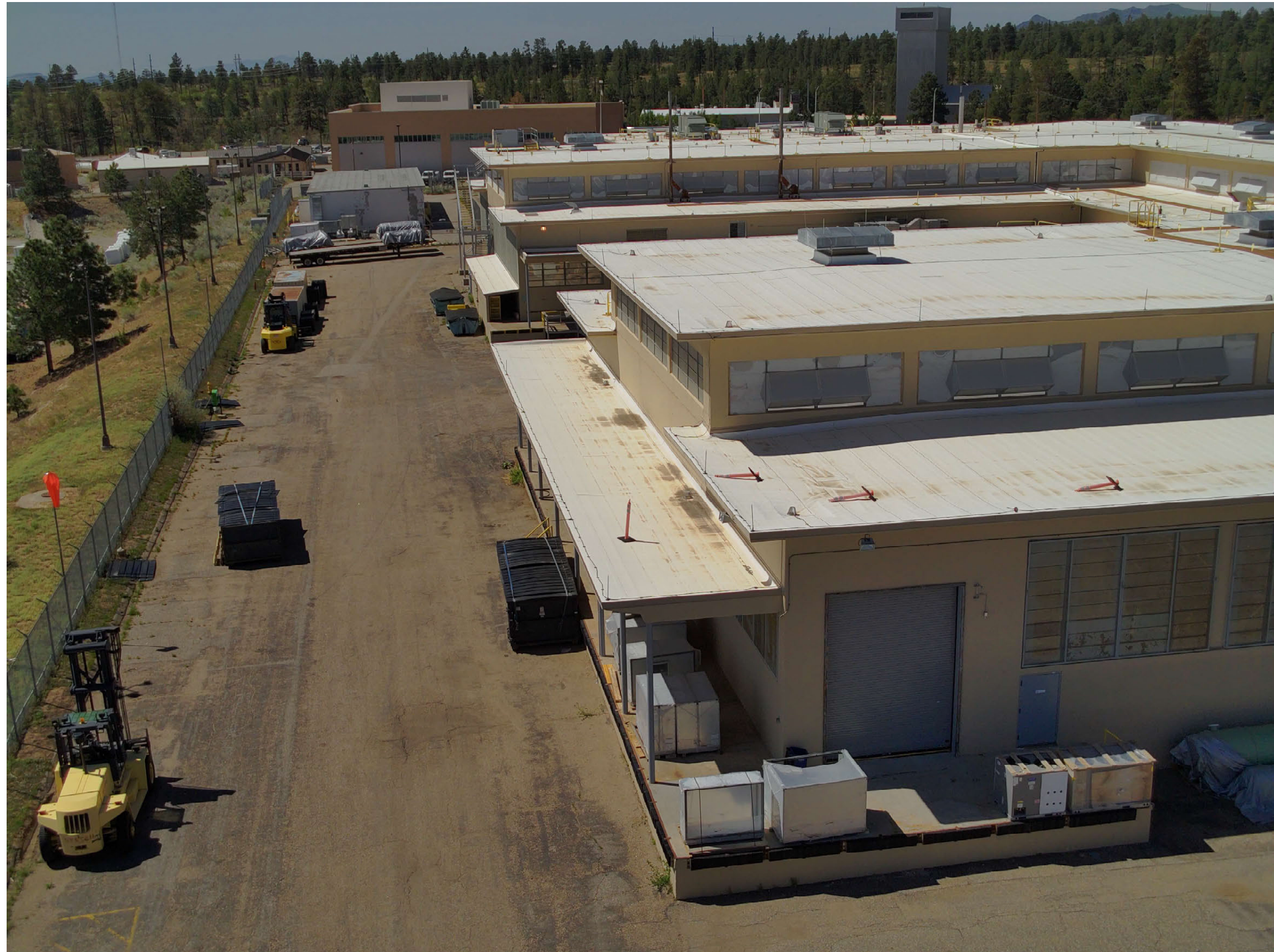
TA-03-0039 center and south wings, north facades
