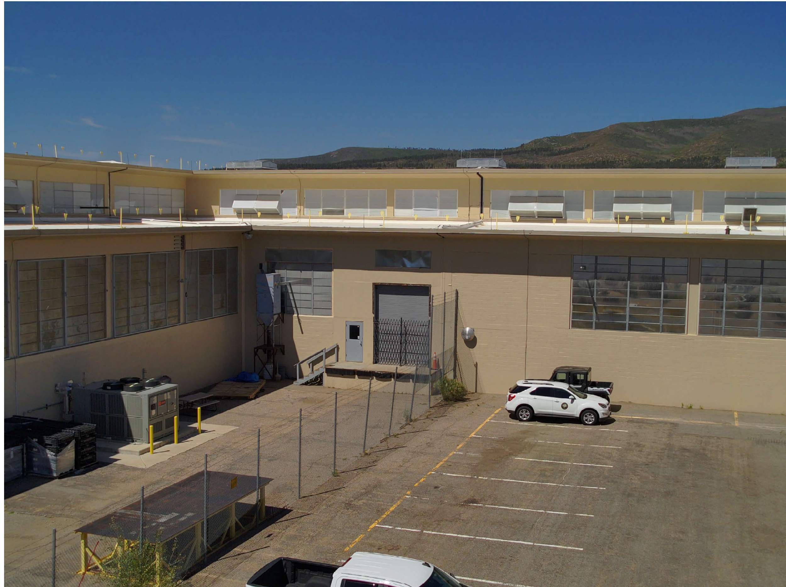
TA-03-0039 center wing (left), north portion of spine (right), north east facades
