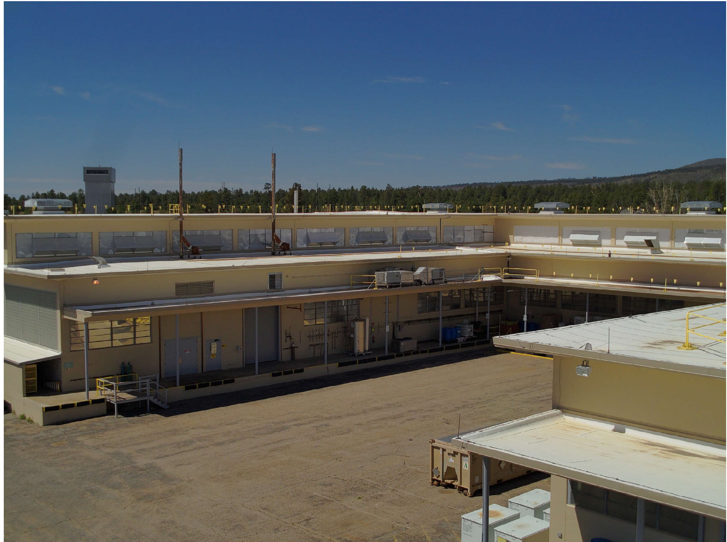
TA-03-0039 south wing, north facade
