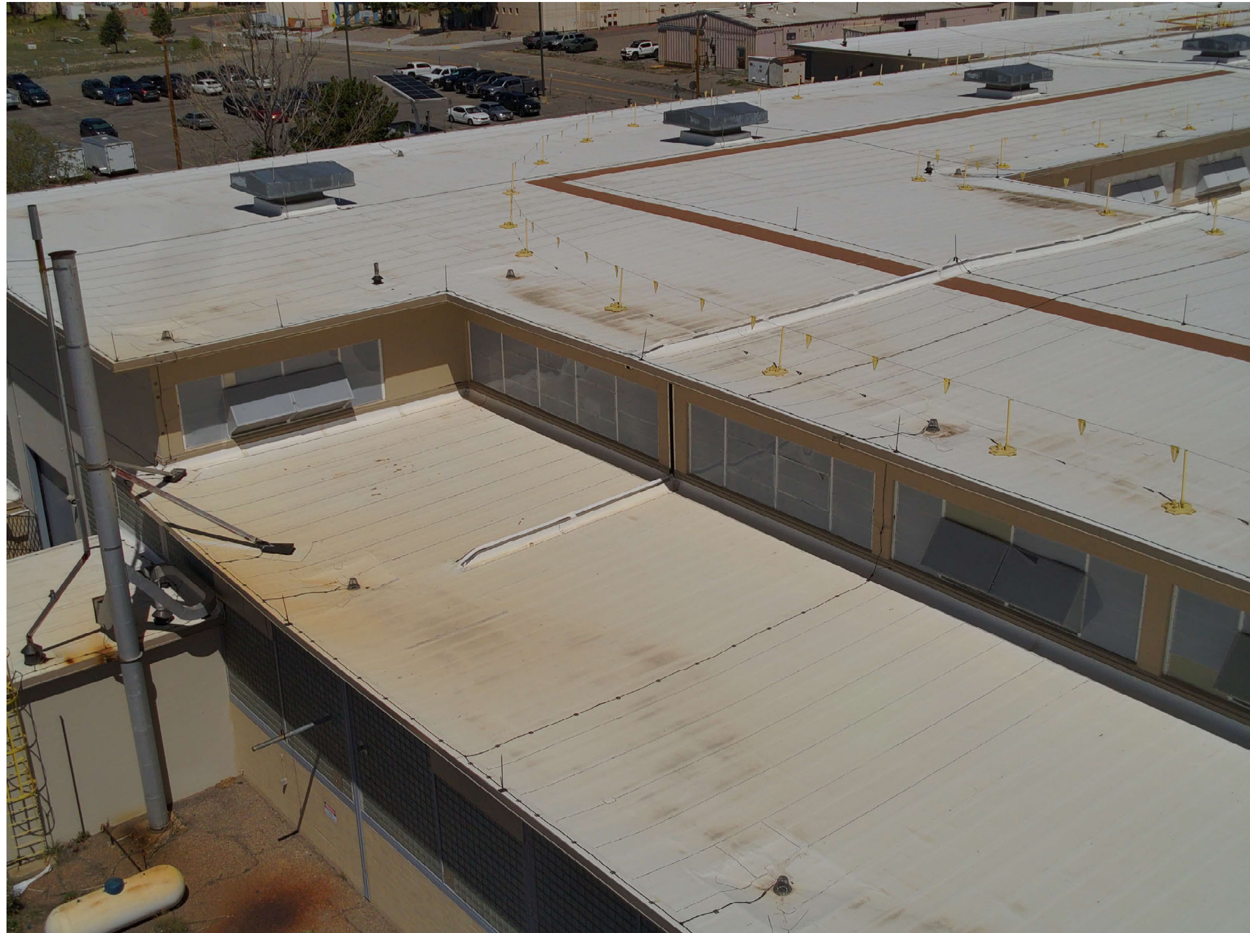
TA-03-0039 south wing clerestory, south and east facades
