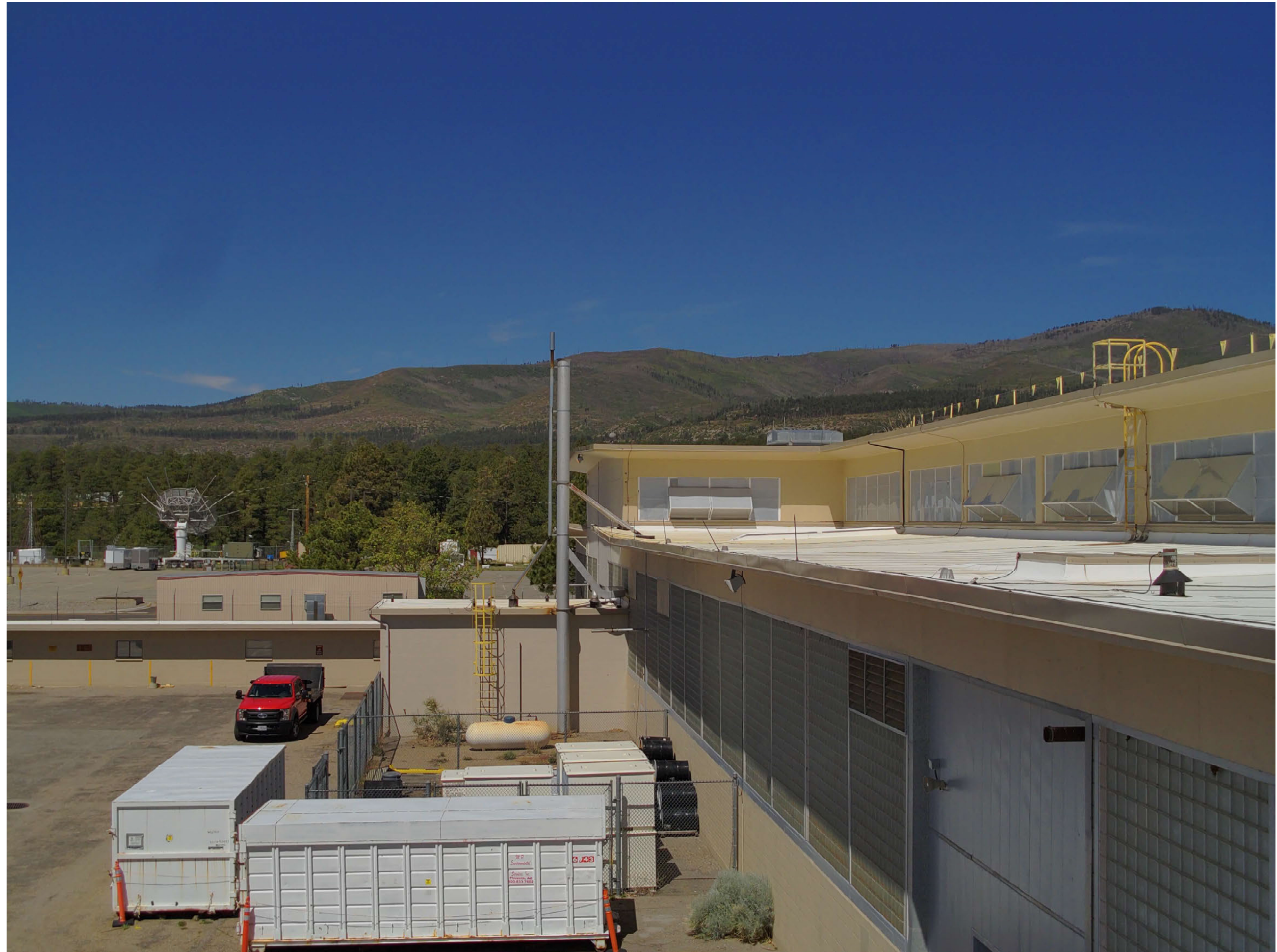
TA-03-0039 south wing, south facade
