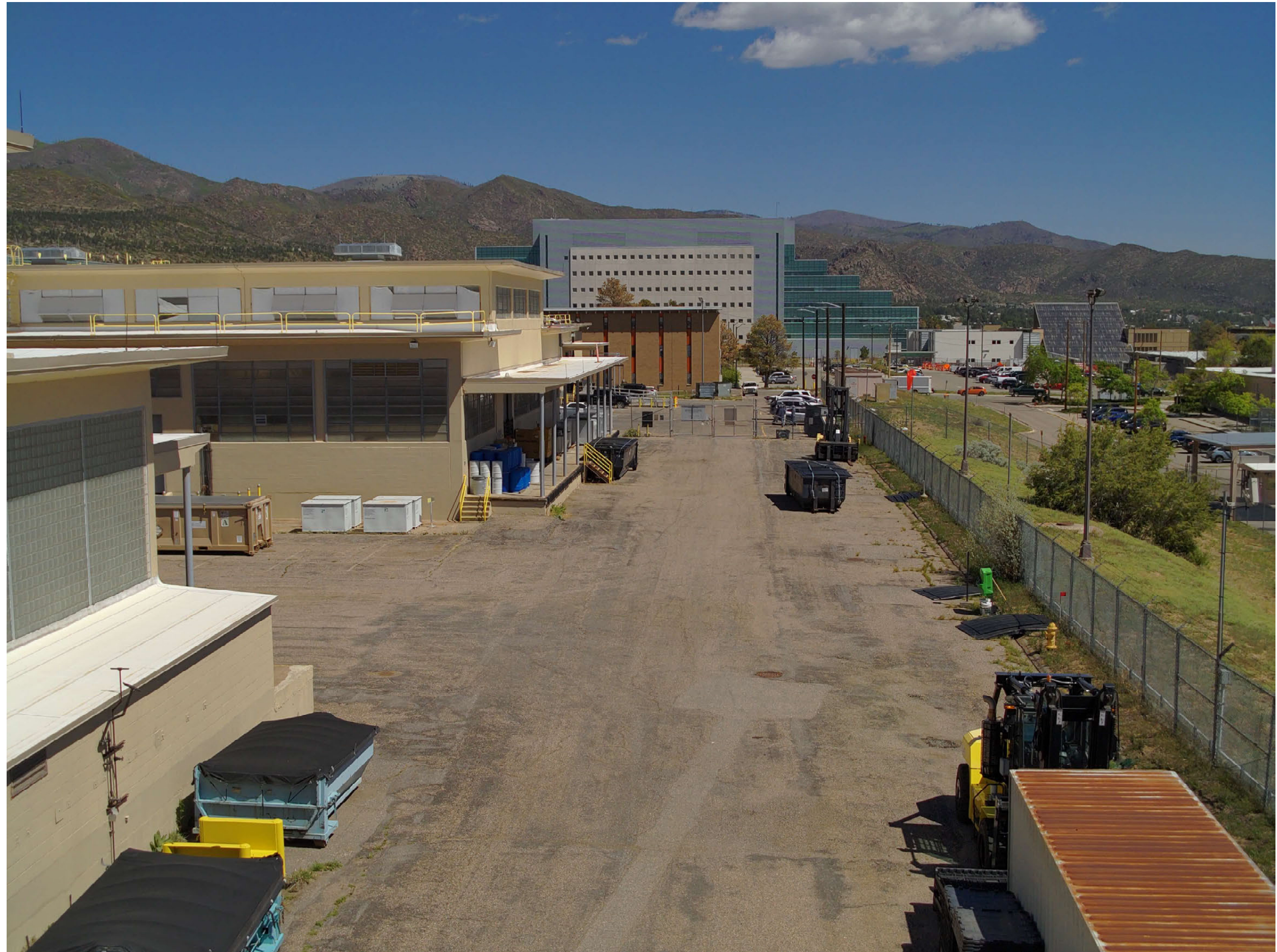
TA-03-0039 center wing, south facade
