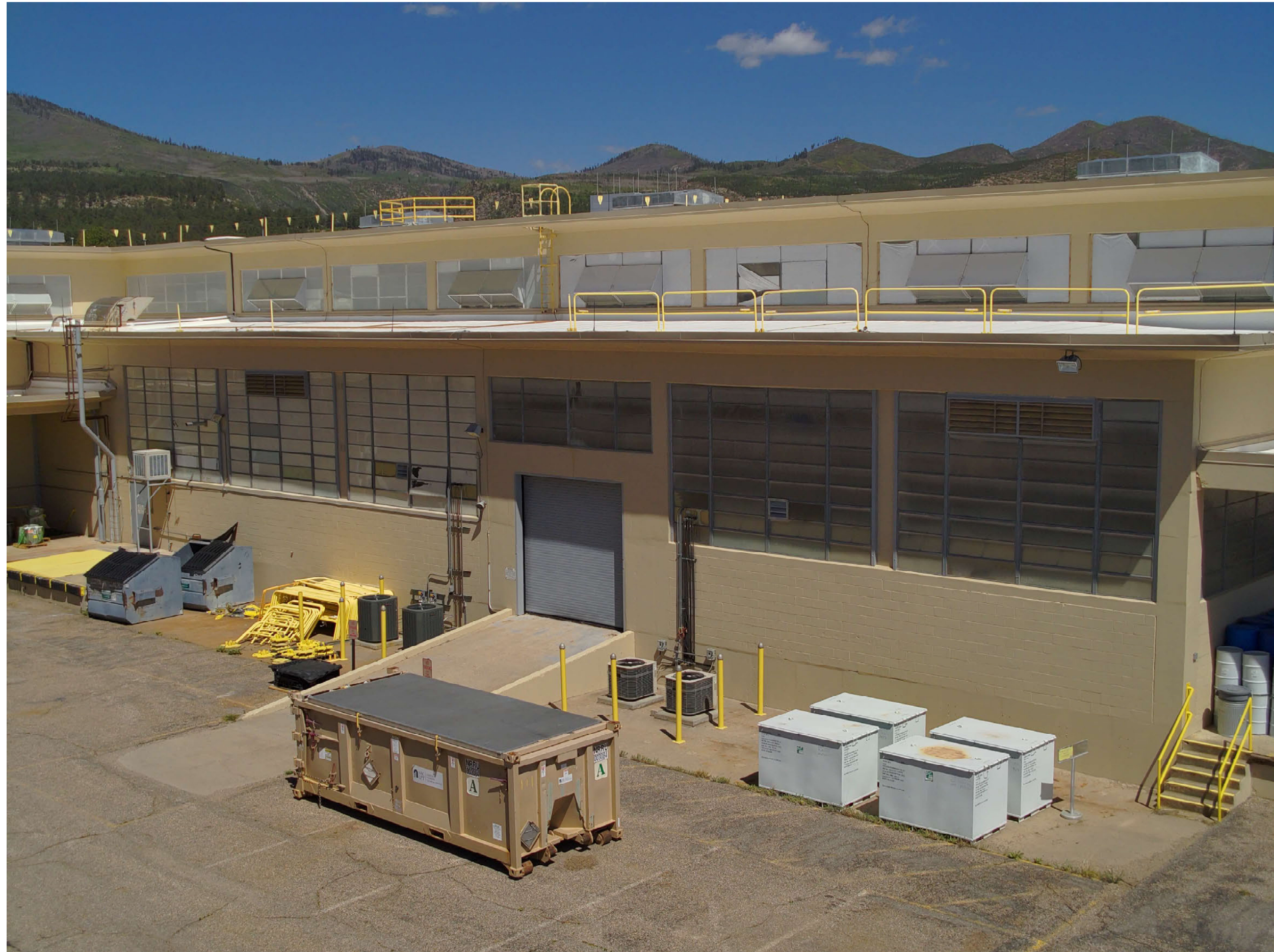
TA-03-0039 center wing, south facade
