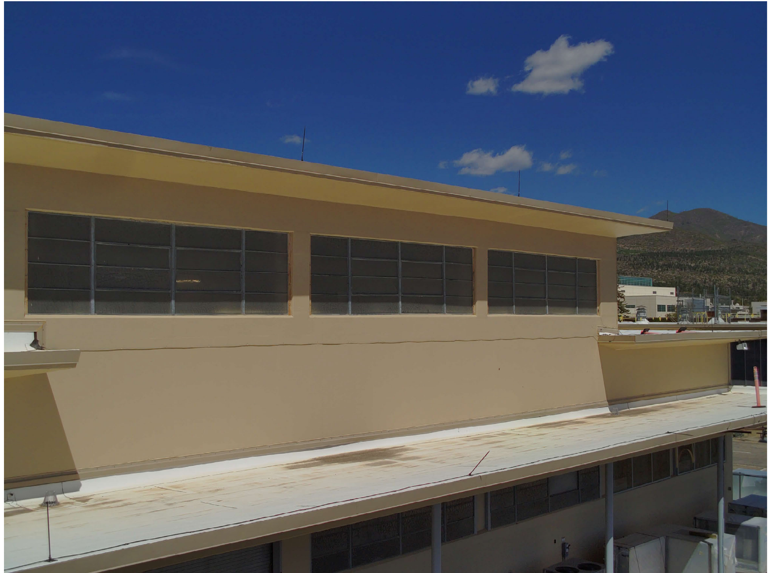
TA-03-0039 center wing, east facade
