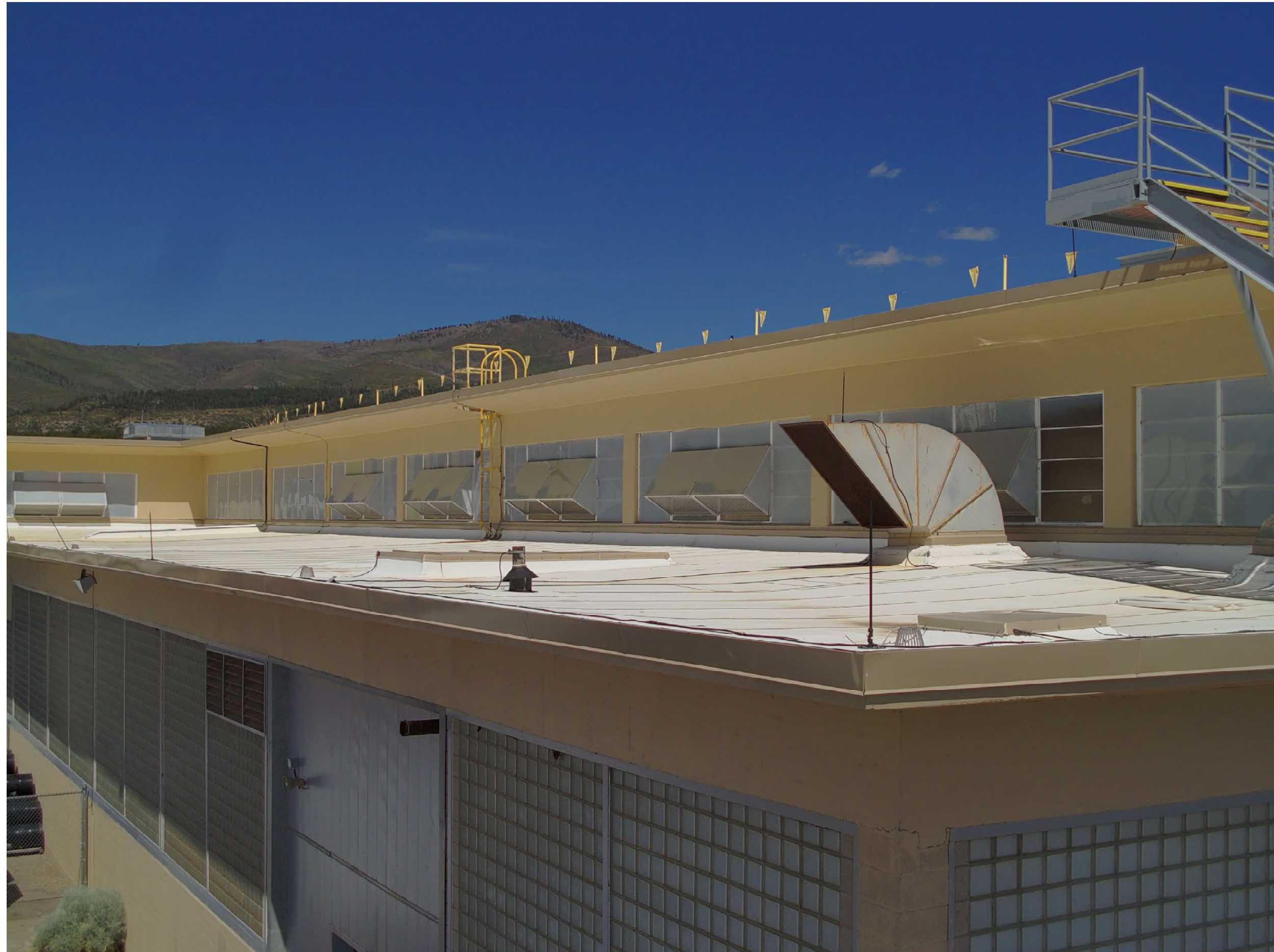
TA-03-0039 south wing, south facade
