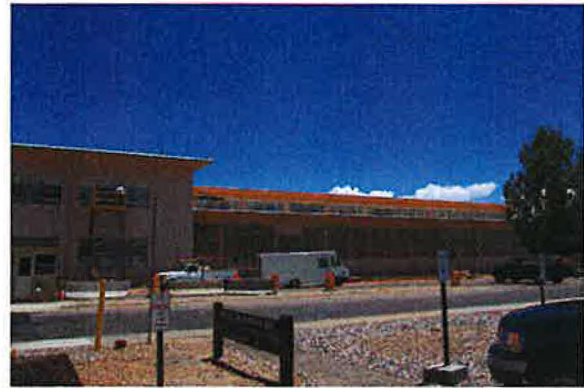
Figure 2: South end of west elevation.
