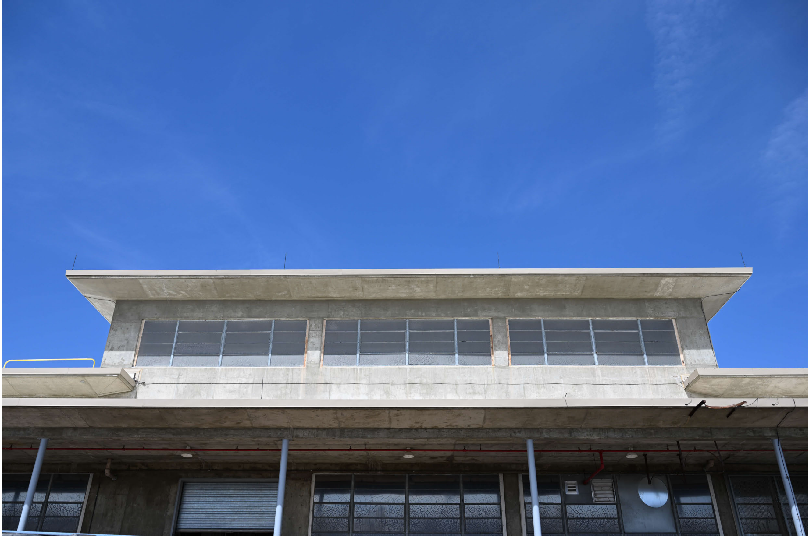
TA-03-0039 center wing, east facade
