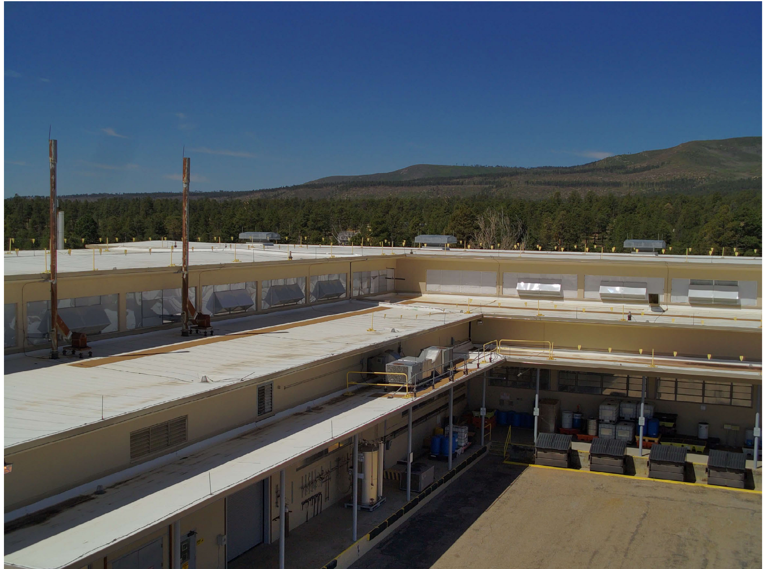
TA-03-0039 south wing (left), south portion of spine (right), north and east facades
