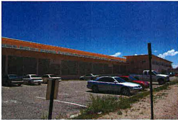
Figure 1: North end of west elevation.
