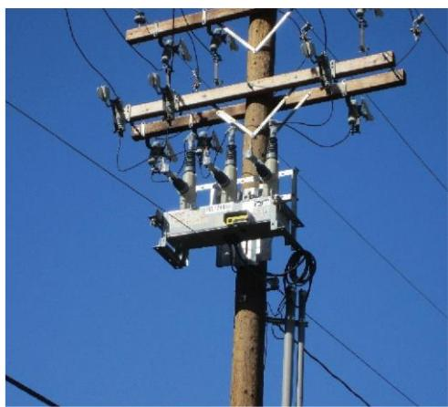
**Figure 3.4:** Recloser on the primary distribution level with remote control capabilities.
