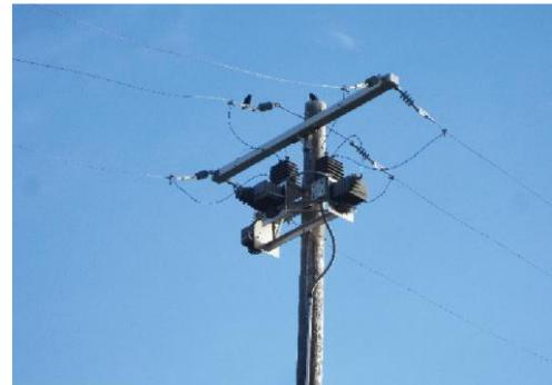
**Figure 3.3:** Primary distribution line with three phase voltage measurement.
