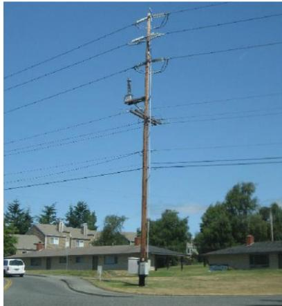
**Figure 3.2:** Sub-transmission line with voltage measurement on a single phase.
