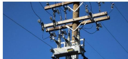
**Figure A.9:** Three-phase recloser on primary distribution system.
