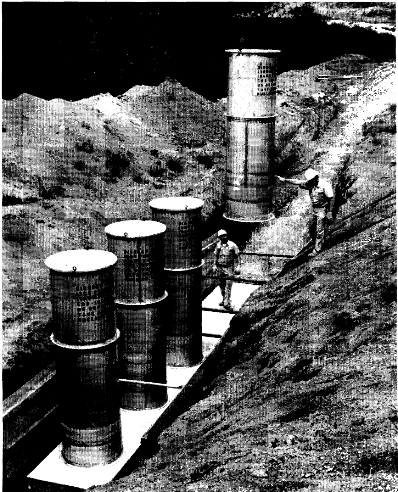
Figure 6. Unfilled lysimeter vessel being lowered into position at ORNL.
