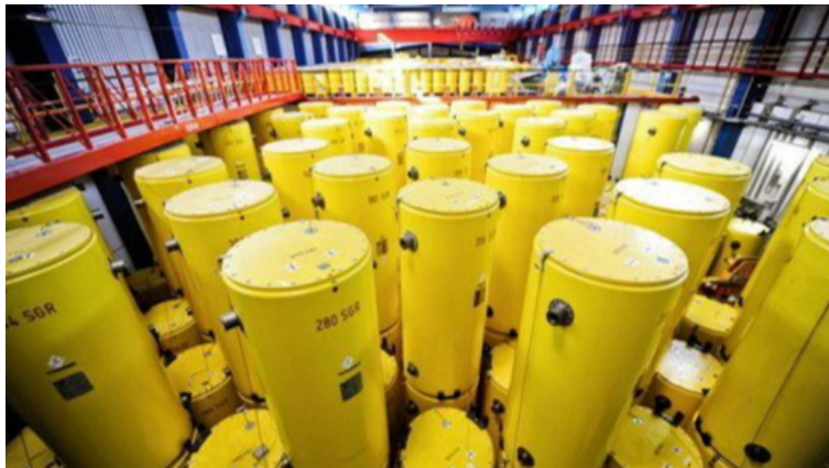
Figure 5: Some facilities have tightly packed casks, and access to seals at the top of casks is achieved via crane or bridge. Image from [8].
