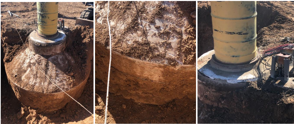
Figure 16. Heliostat base extraction depicting (left to right), concrete support, a more detailed view, and electrical cables.
