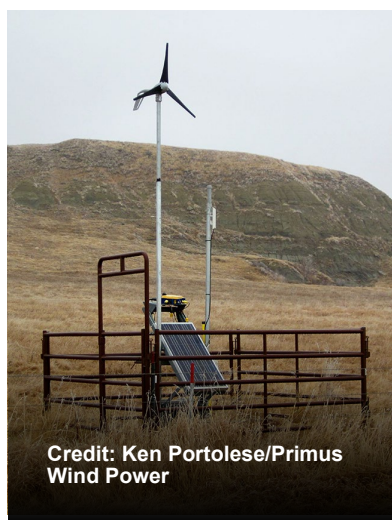
Figure 4. Distributed wind energy hybrid system powering a remote monitoring station.
