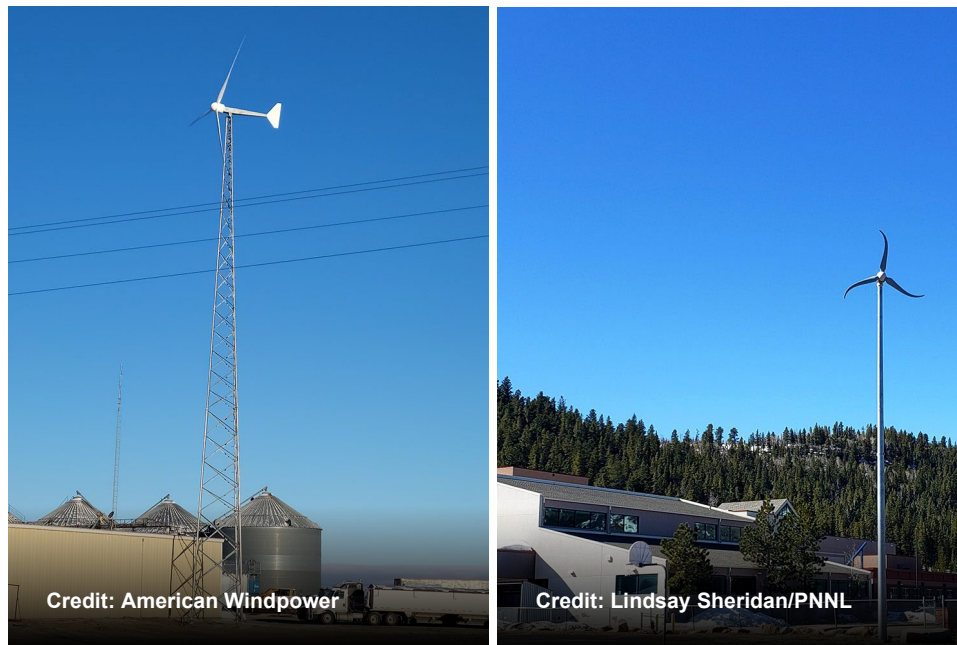
Figure 7. Comparison of lattice (left) and monopole (right) turbine towers.
