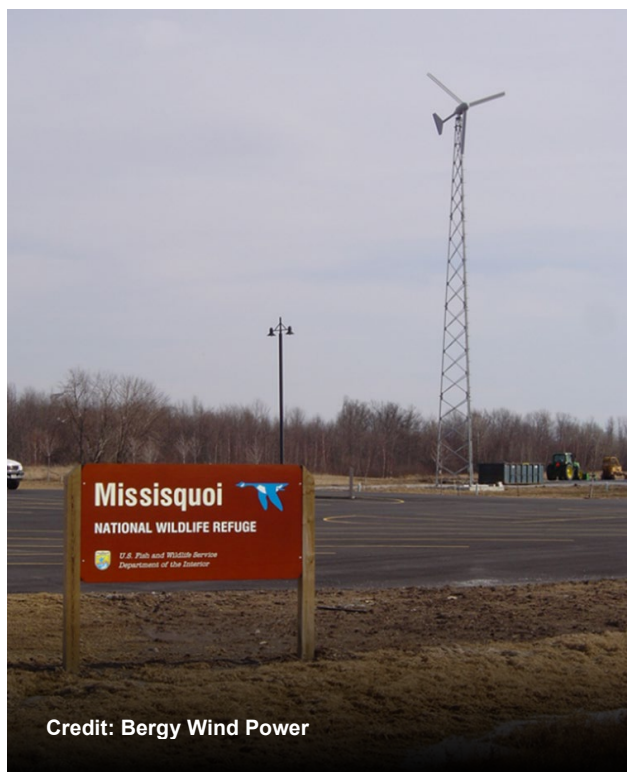
Figure 11. The 10 kW Bergey Excel 10 wind turbine at Missisquoi National Wildlife Refuge in Swanton, Vermont.
