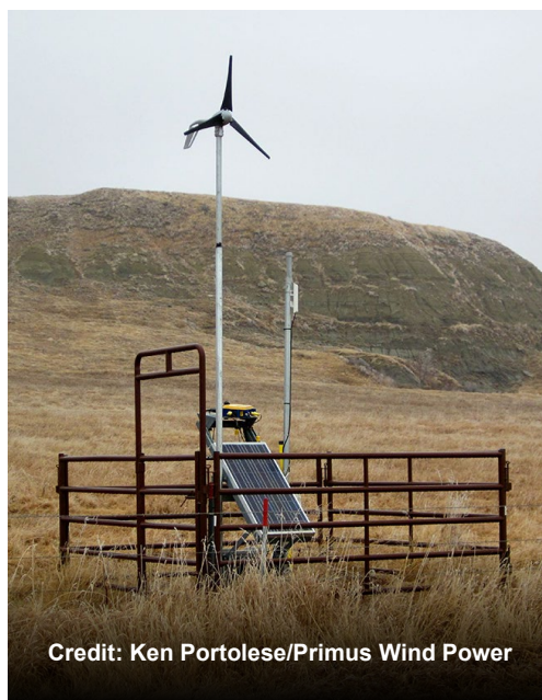
Figure 8. Distributed wind energy hybrid system powering a remote monitoring station.
