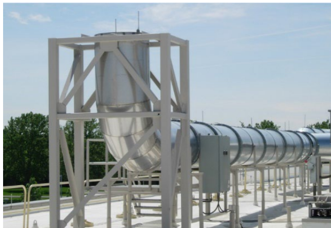
3410 Building Filtered Exhaust Stack
