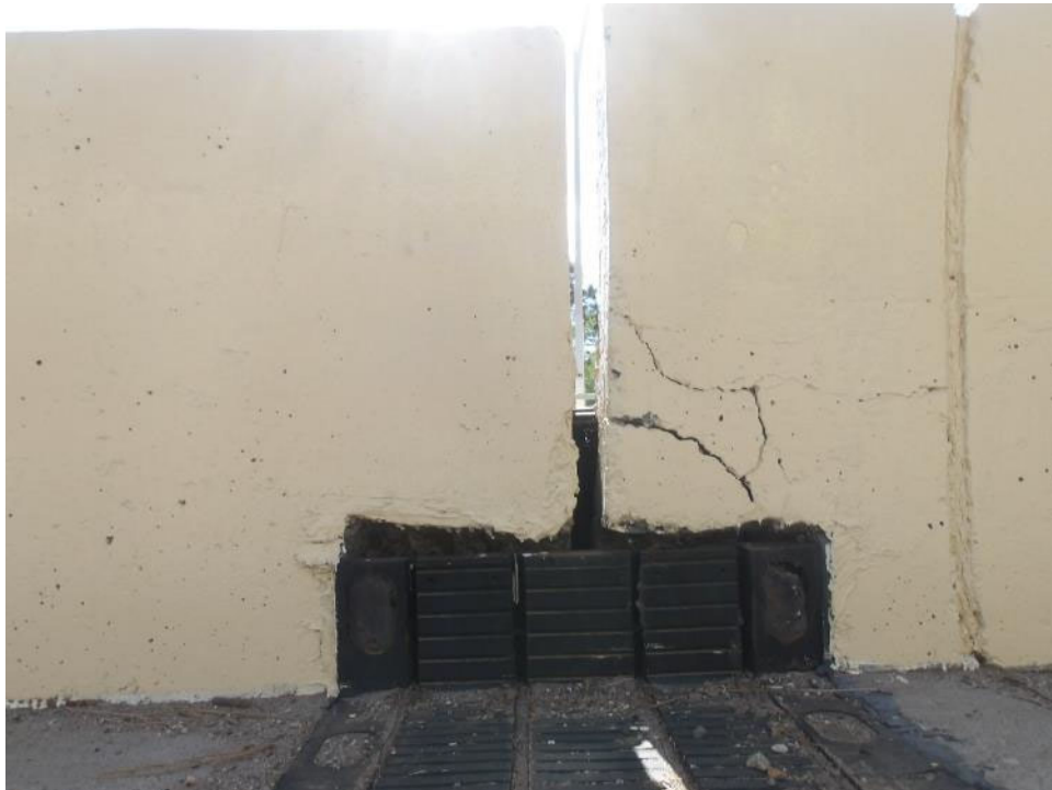
Photo 108- 1/8" crack in the west concrete barrier rail immediately above the southern joint.
