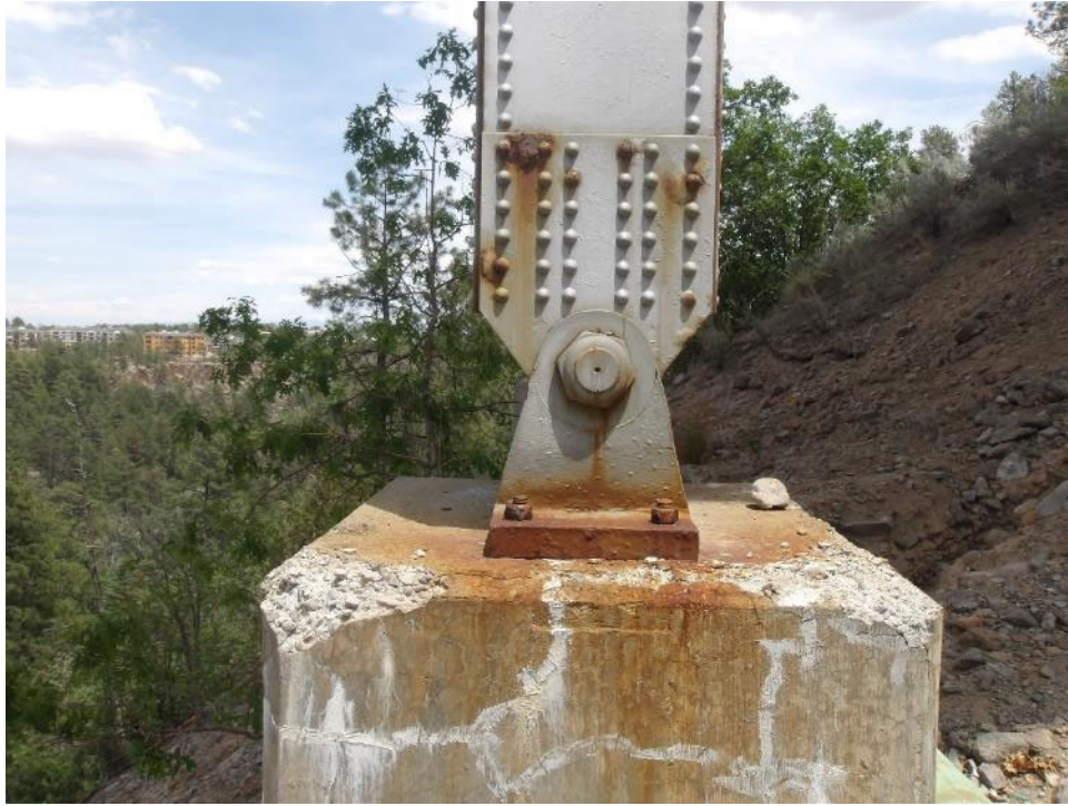
Photo 92- West face of concrete pier column 2, west, with efflorescence and crack repairs. Note 1'x1'x1/2" spall on northwest corner.
