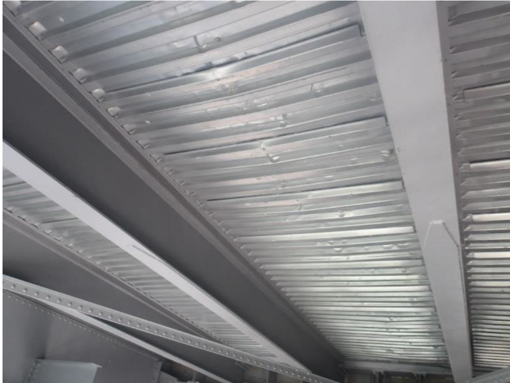
Photo 63- Ends of stringer cover plates in end spans. No defects noted.
