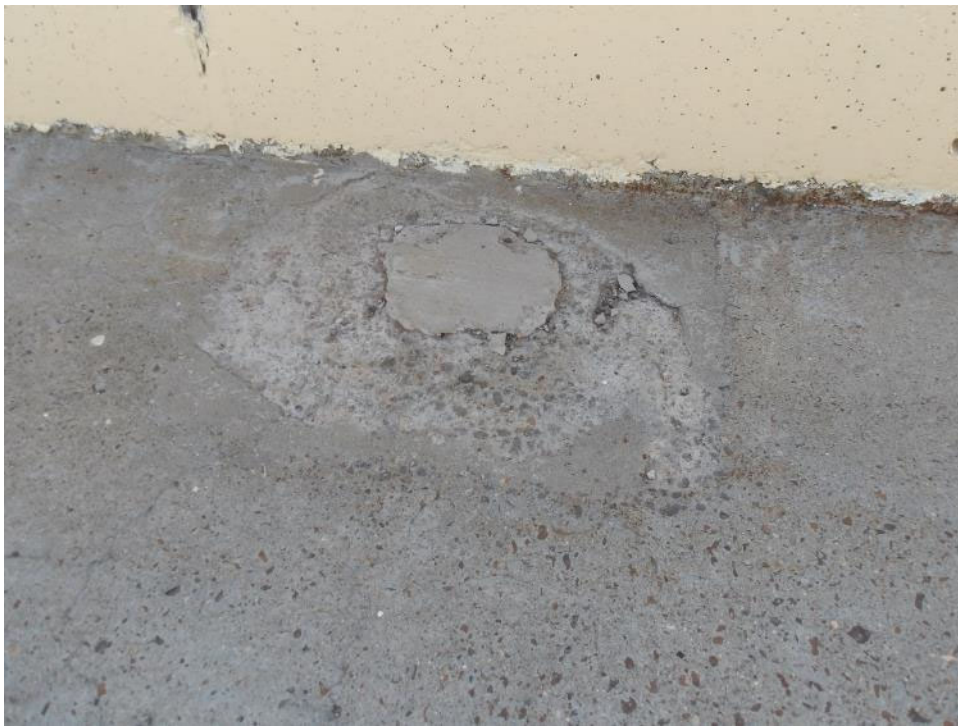
Photo 16- (14"x10"x1/2") spall at failed concrete repair towards north end of the pedestrian walkway.
