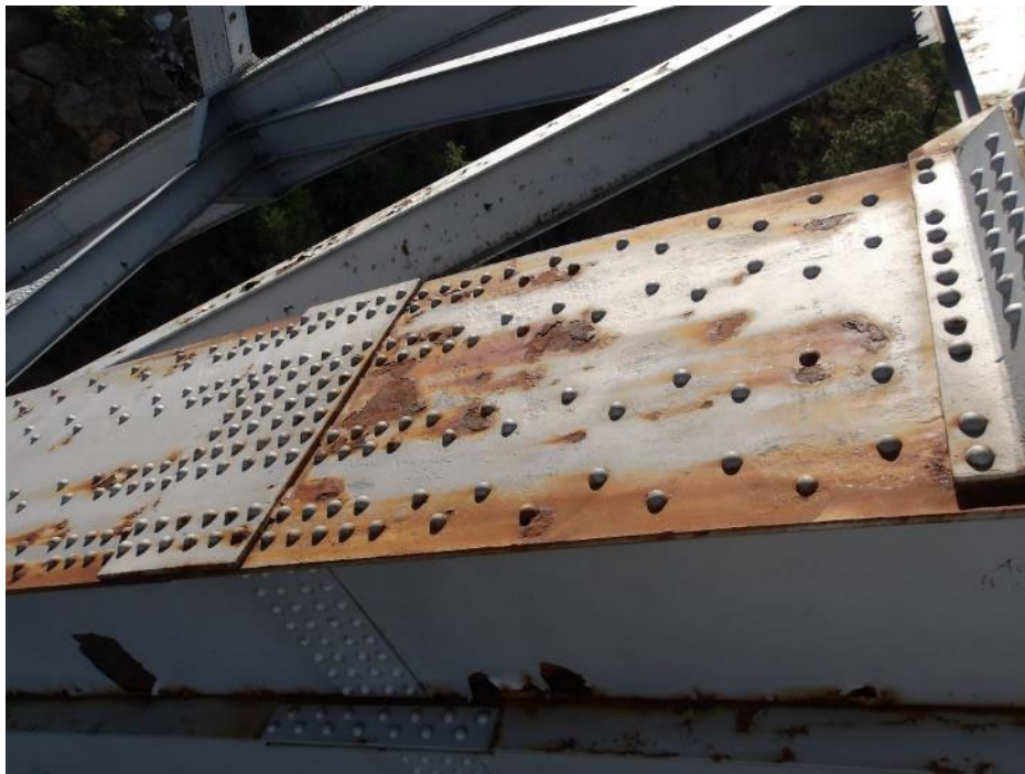
Photo 22- Minor corrosion on top plate of west arch at column 11.
