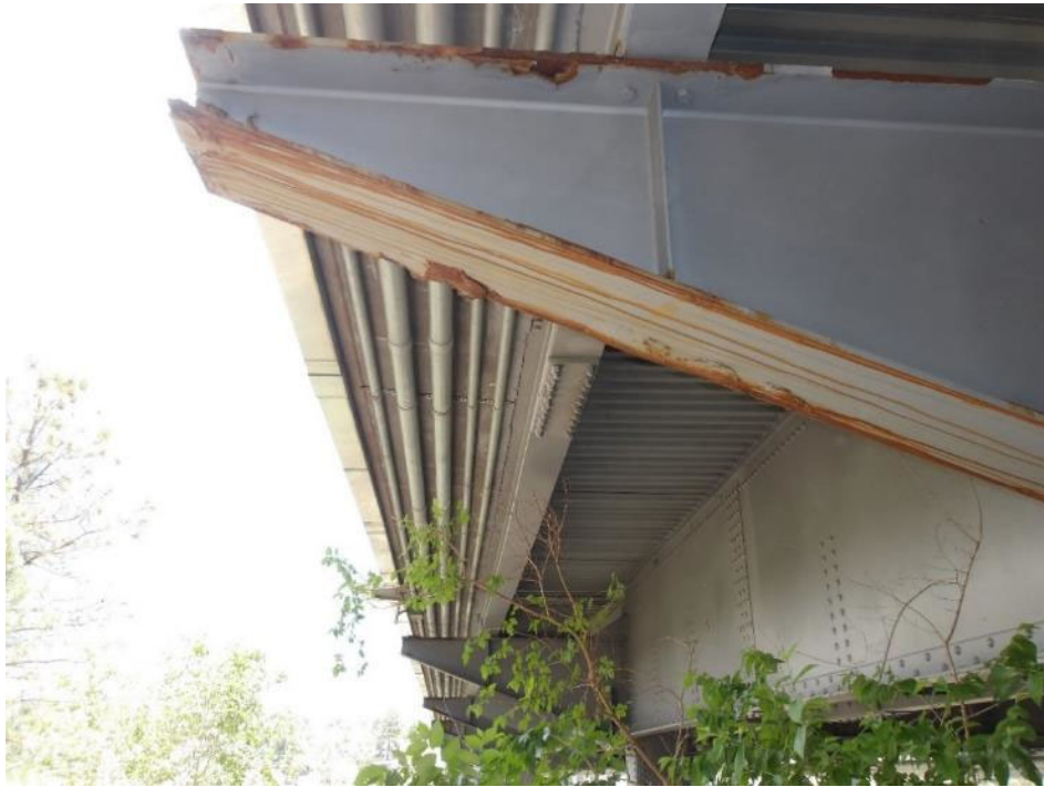
Photo 49- View of outrigger at FB2 on West side, minor surface corrosion.
