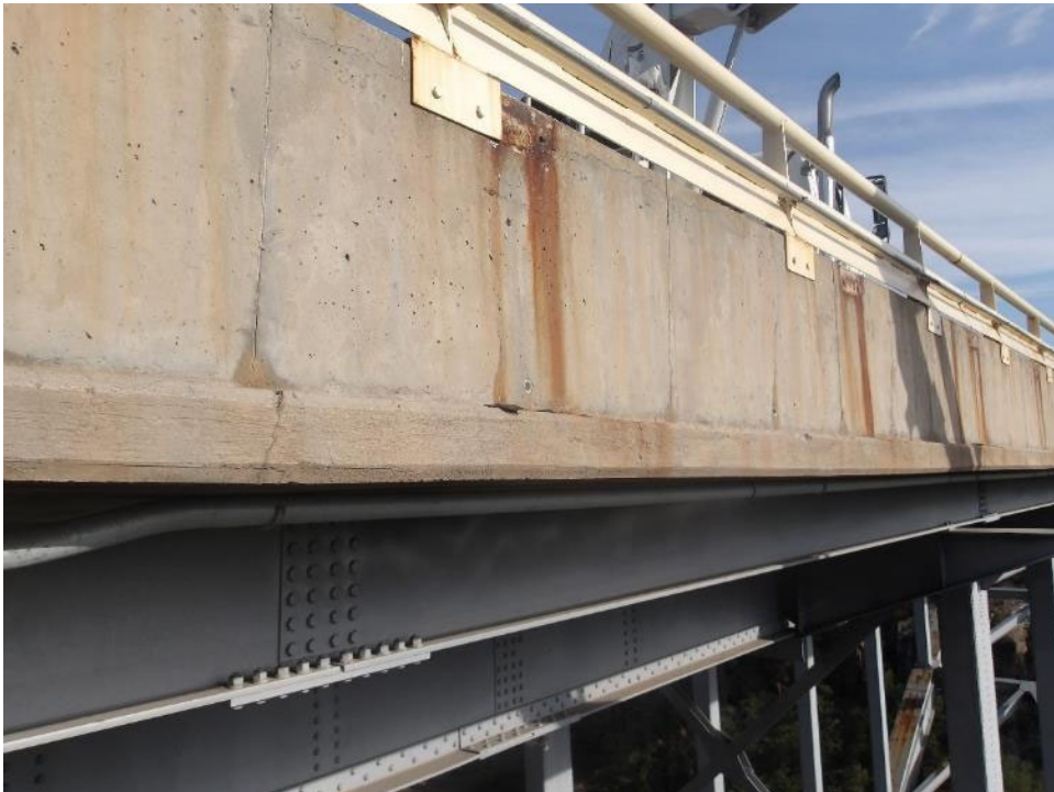
Photo 8– General photo of east fascia. Note rust staining and cracking.
