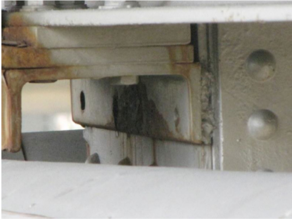
Photo 41- Missing bolts and poorly welded connection at top of arch column. No change since previous inspection.
