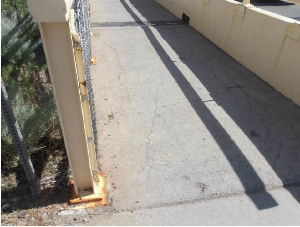
Photo 13- Map cracking at the north end of the pedestrian walkway (TYP).
