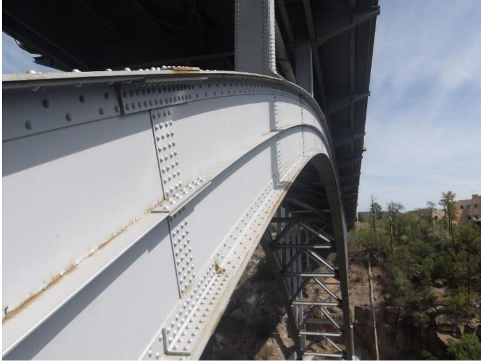
Photo 25- Minor corrosion on east arch at column 5.
