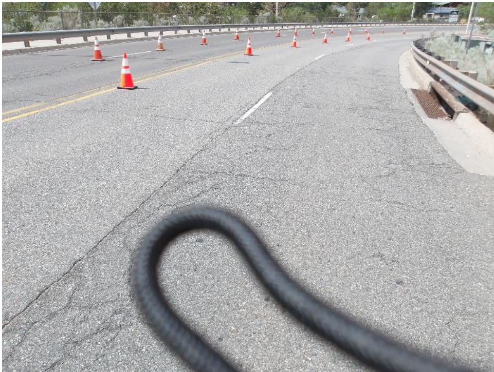
Photo 103- North approach looking north with random cracking.
