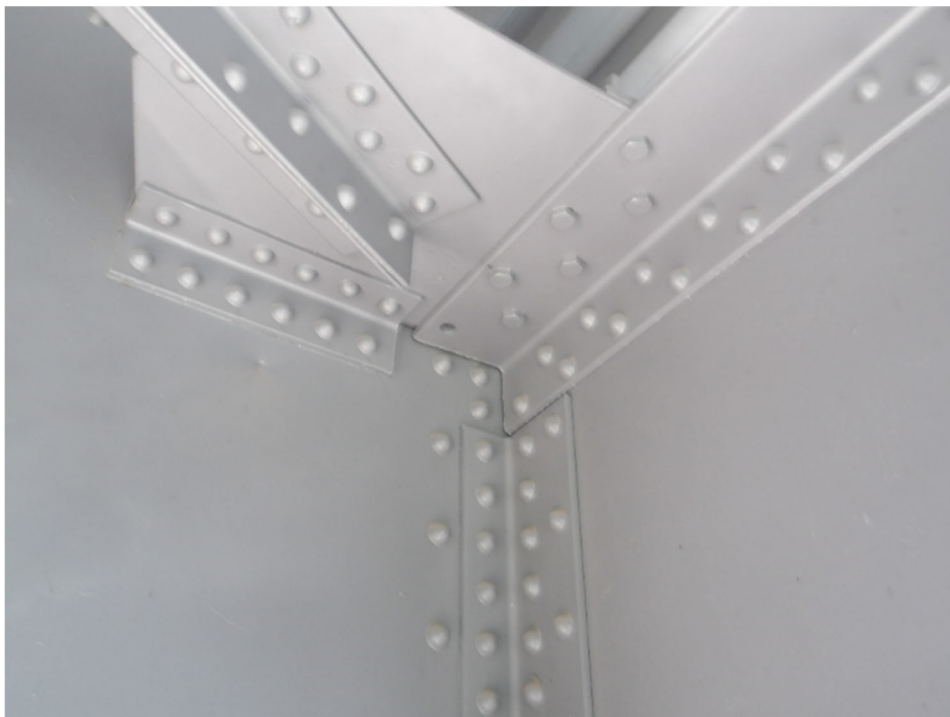
Photo 58- Typical missing bolt at connection of floorbeam angle to outrigger connection.
