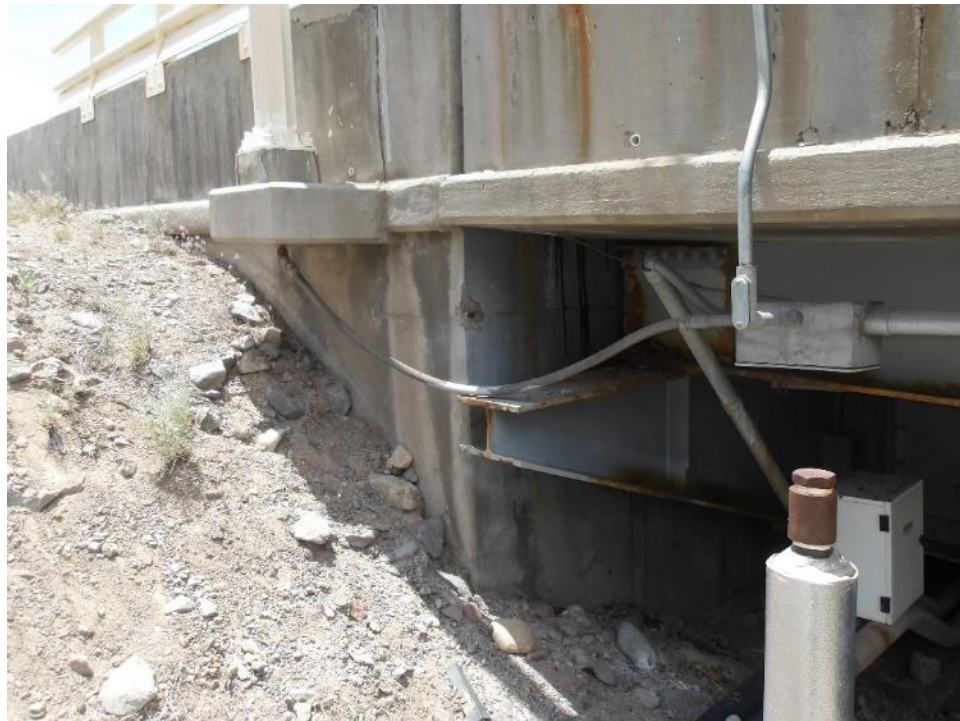
Photo 71- East wingwall at south abutment. Small spall with exposed reinforcement.
