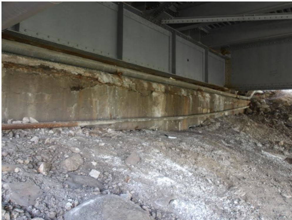
Photo 65- Delamination, spalling and exposed rebar at south abutment top strut. Minor erosion of soil around abutment.
