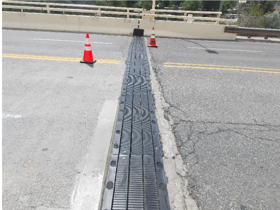
Photo 104- Deterioration of asphalt and concrete on the approach side at the north abutment joint.
