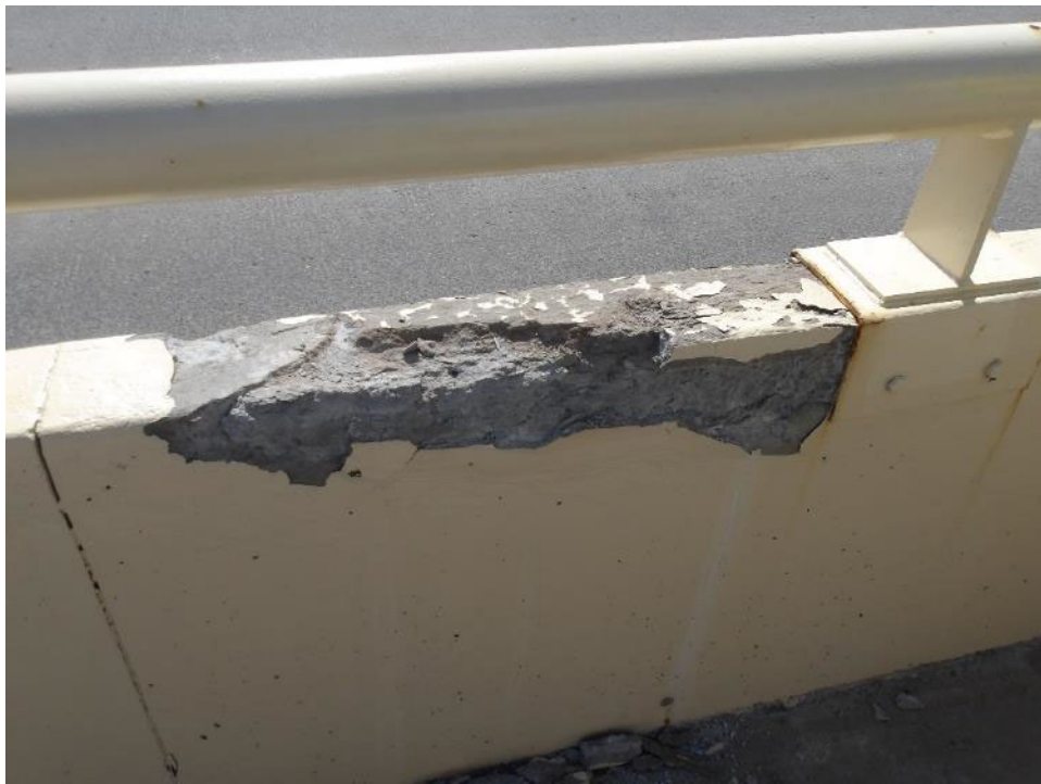
Photo 110- Large (3'xFull Widthx1") spall in the west concrete barrier rail at midspan.
