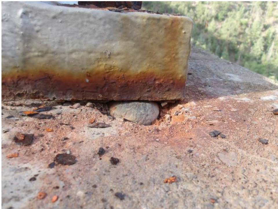
Photo 93- 1/2" deep undermining at the northwest portion of the bearing pad at concrete pier column 3, west.
