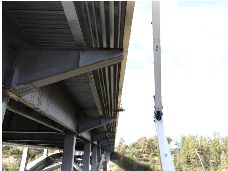
Photo 50- General view of outriggers in satisfactory condition, taken on west side at arch column 11.
