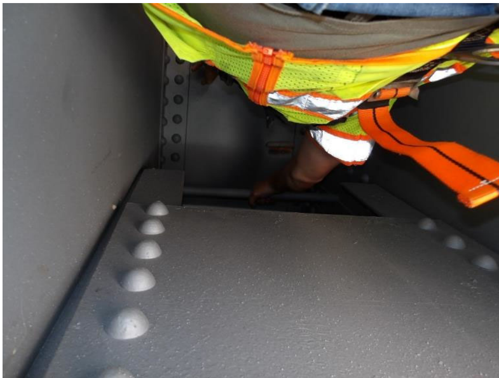
Photo 46- Hands-on inspection of top plate of spandrel girder and through anchor bolts for outriggers.
