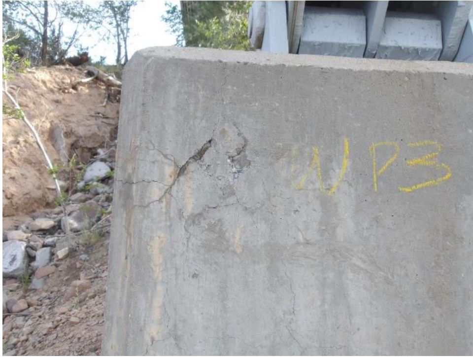
Photo 94- 8"x8" area of delamination with small spalls and associated cracking (hairline to 1/16") at southern face of concrete pier column 3, west.
