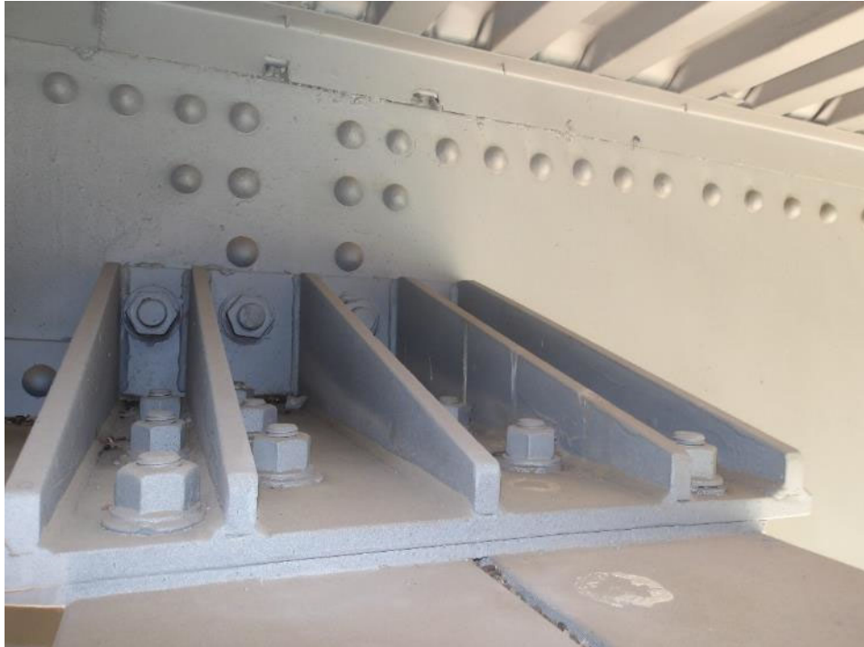
Photo 53- Typical connection of outrigger to floorbeam on interior side in good condition.
