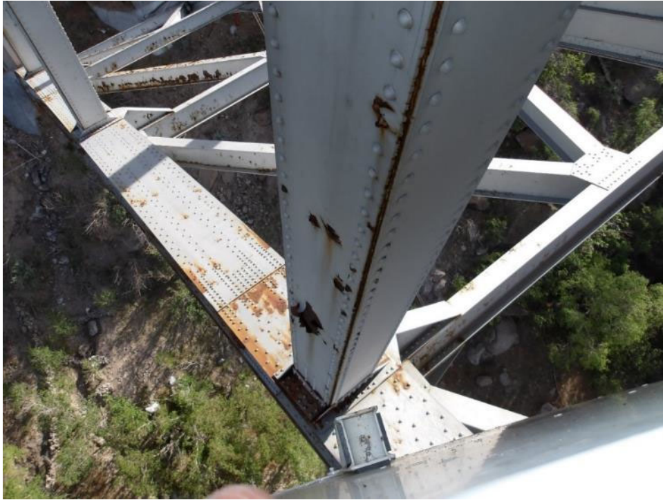
Photo 33- Surface corrosion and paint failure at arch column 11, west.
