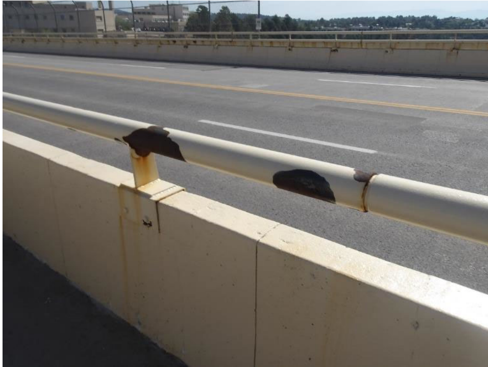
Photo 111- Paint failure along the western rail at midspan (TYP).
