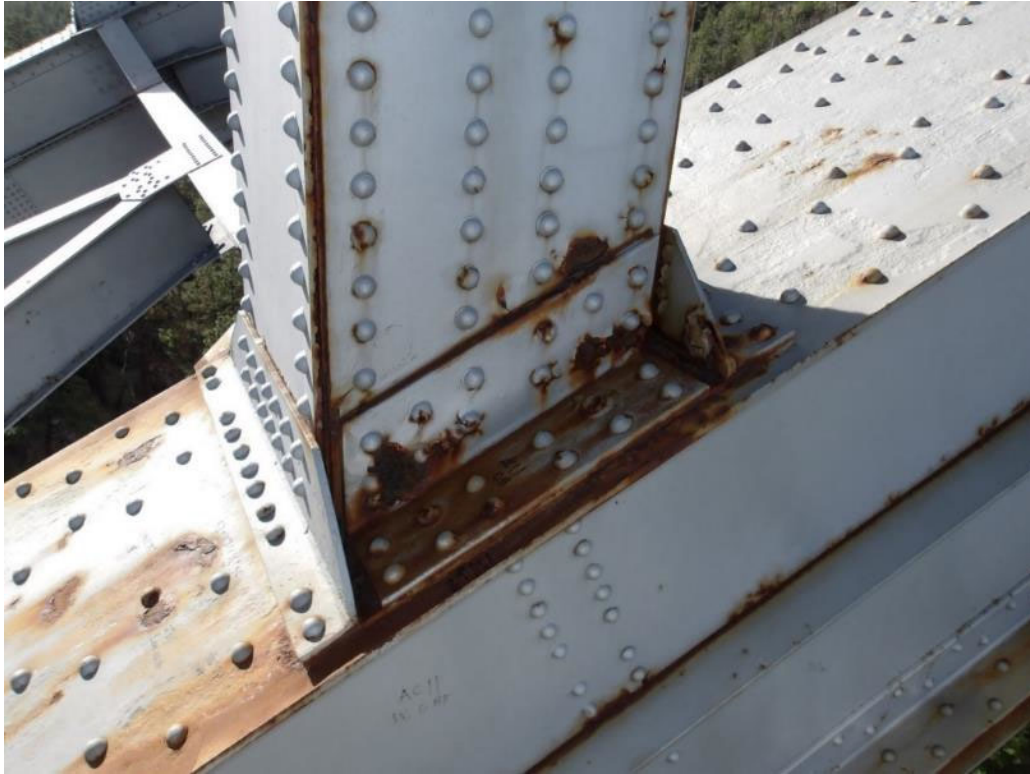
Photo 37- Heavy corrosion and minor thickness loss ( 1/32'' ) at the steel angle connection of arch column 11W.
