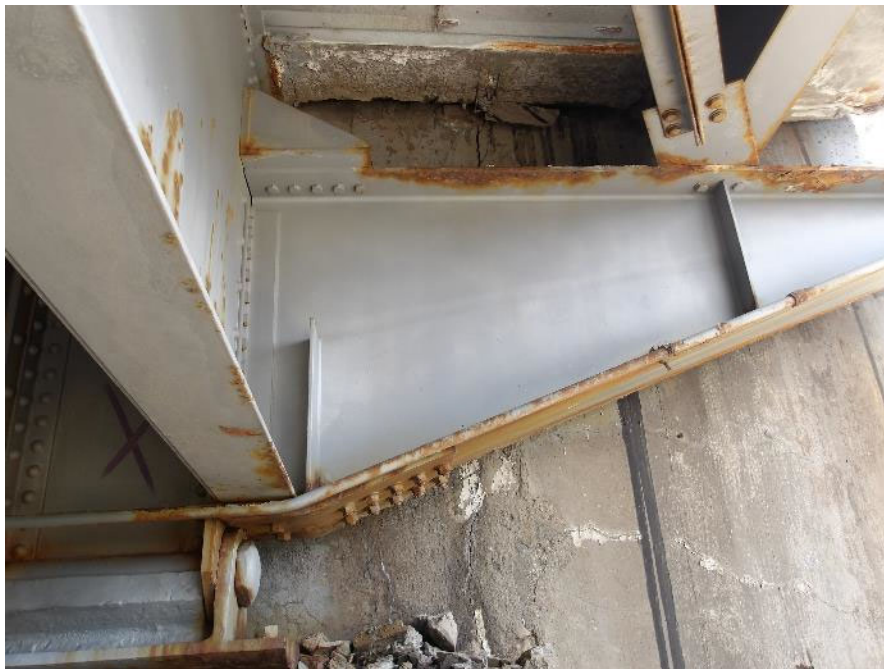
Photo 77- Medium width vertical crack and hairline horizontal cracking on east face of backwall at north abutment.
