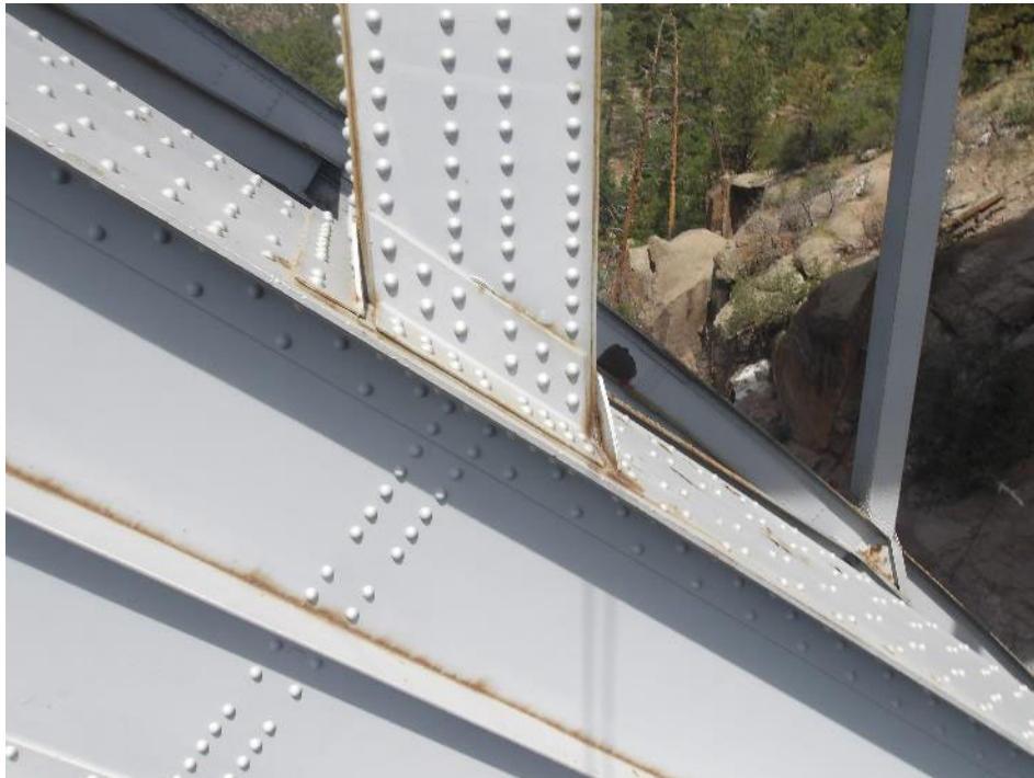
Photo 36- Arch column 13E, minor corrosion at base.
