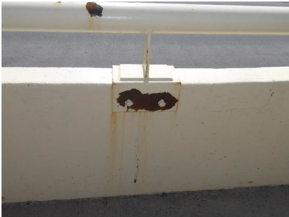
Photo 112- Paint failure at the west guardrail-concrete barrier rail connection.
