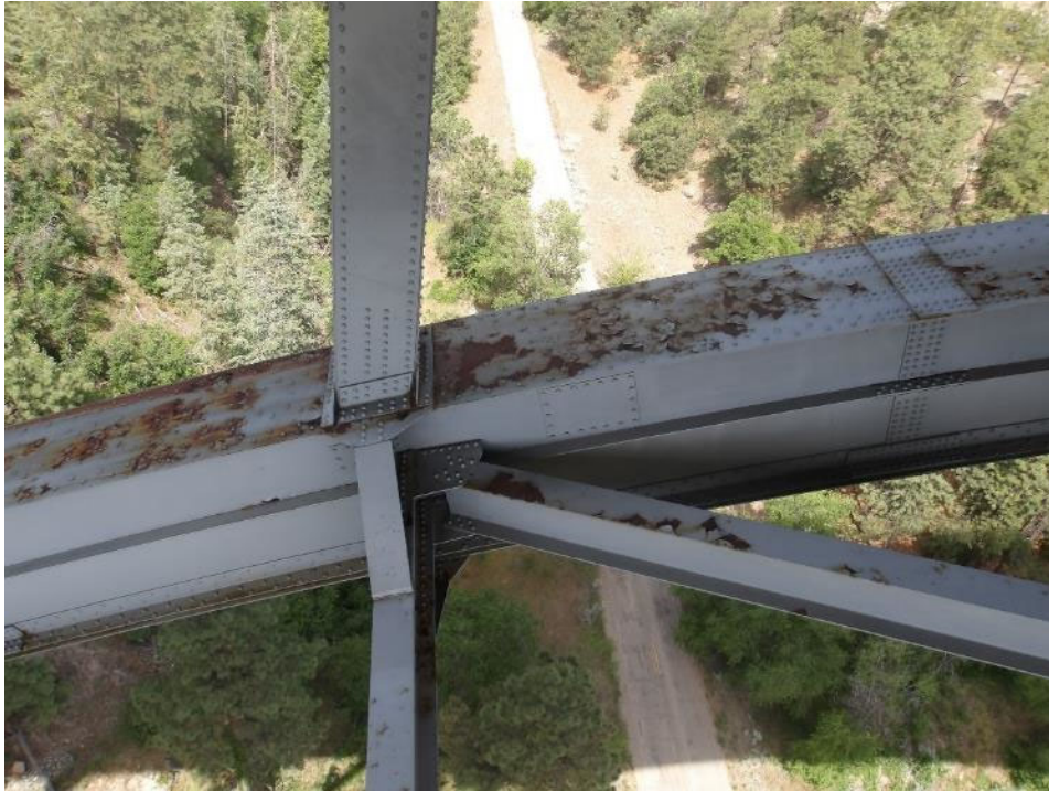
Photo 21- Minor corrosion on top plate of west arch at column 5.
