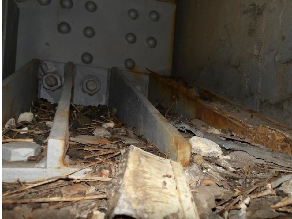
Photo 55- East interior outrigger connection at south abutment, debris buildup and minor corrosion.
