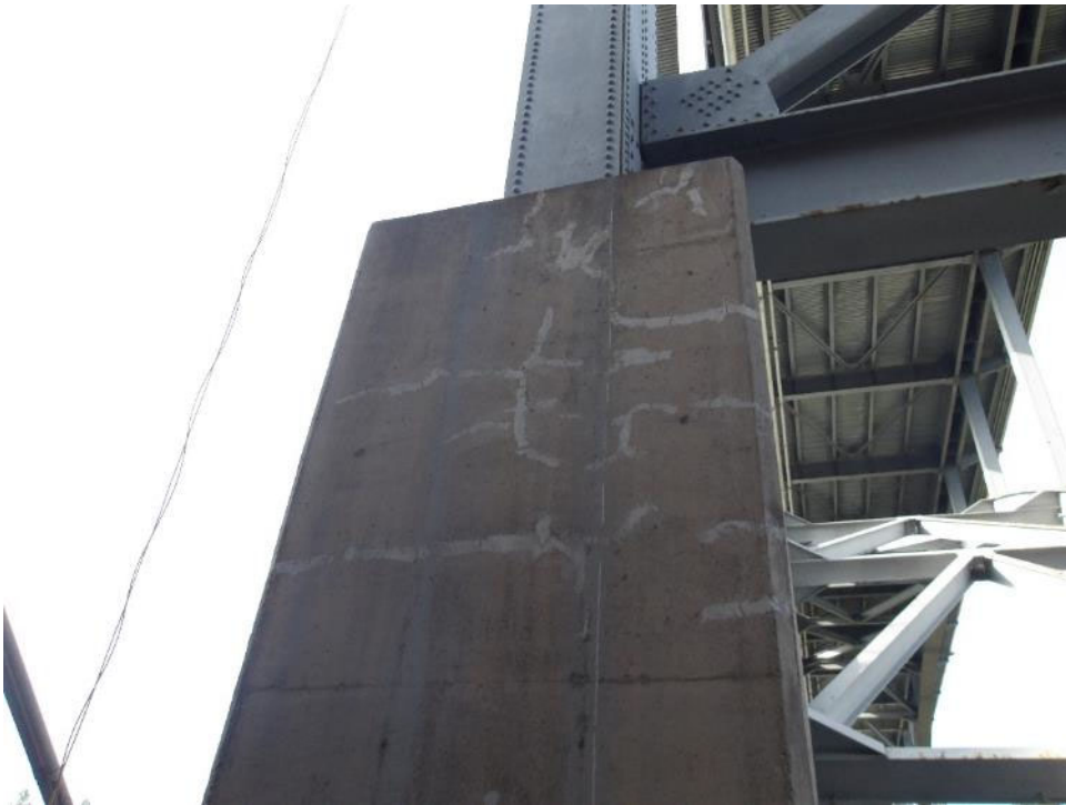
Photo 95- North face of northeast skewback column with patched hairline cracking.
