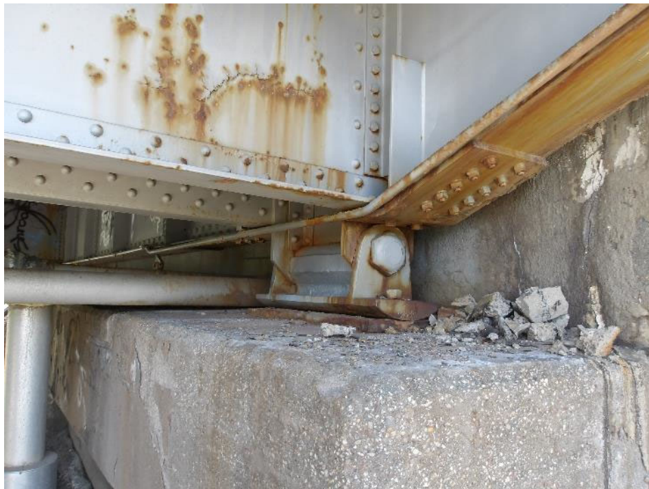
Photo 87- Northeast rocker bearing with paint failure corrosion.
