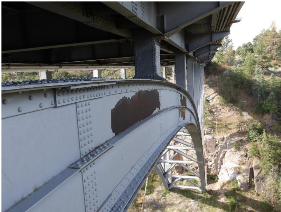
Photo 20- West arch rib at column 7, peeling paint and minor surface corrosion with no measurable section loss.
