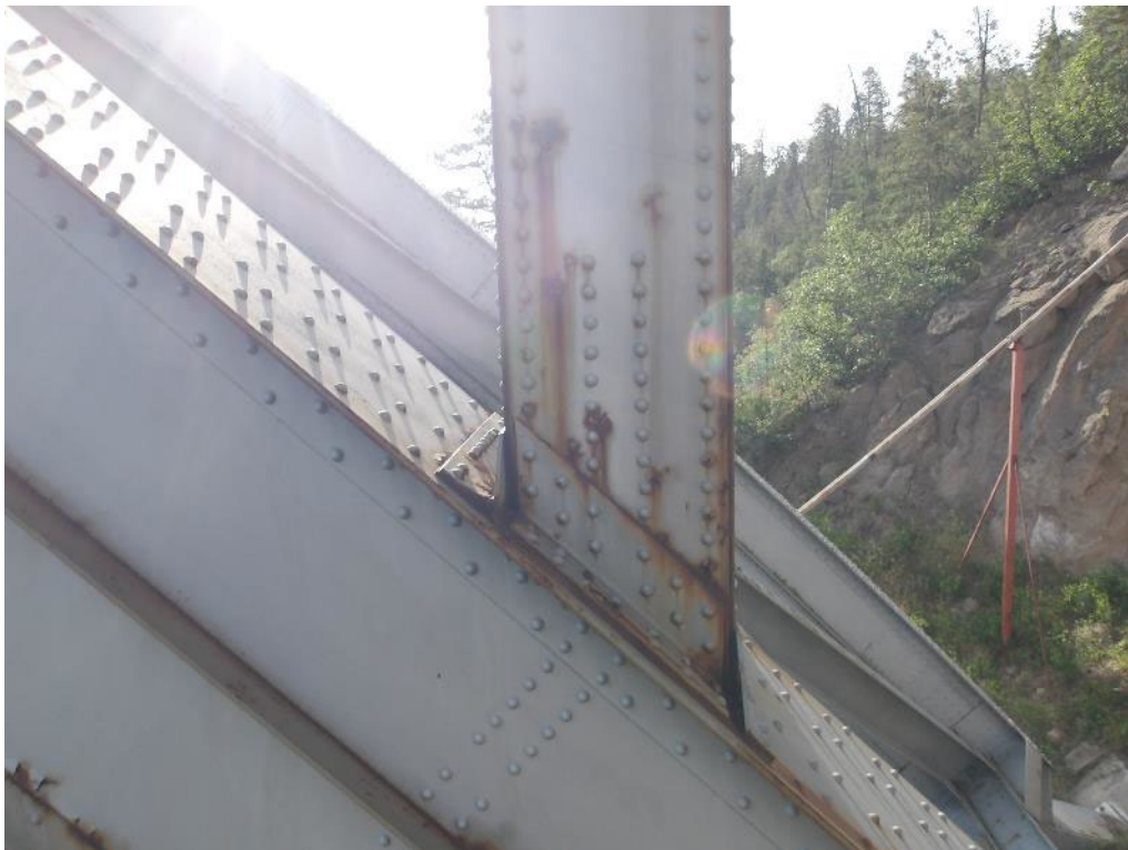
Photo 40- Moderate corrosion on W side of arch column 1W.
