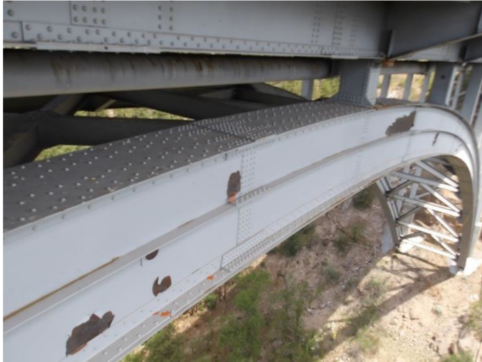
Photo 19- East arch rib at column 7, peeling paint and minor surface corrosion with no measurable section loss.
