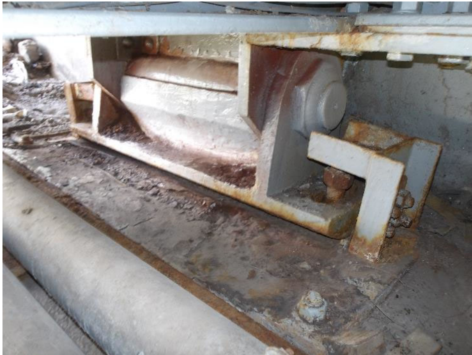
Photo 85- Corrosion and rust staining at southeast bearing with debris accumulation on the abutment seat.
