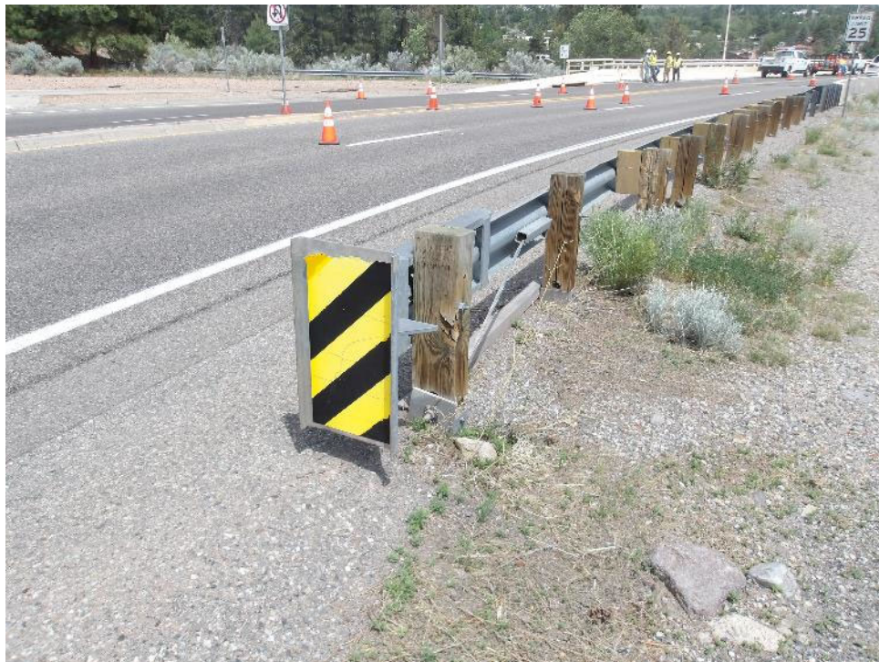
Photo 119- Southeast end terminal. Note new timber blocking place at posts.
