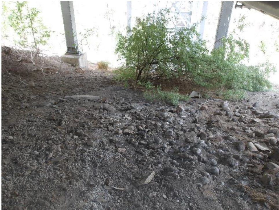
Photo 73- South abutment embankment, looking at pier 1 from south abutment. Minor erosion down slope and around piers.
