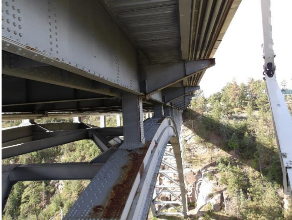
Photo 43- General view of spandrel girder in satisfactory condition, looking at arch column 10W. Note minor corrosion and pack rust at splice location.
