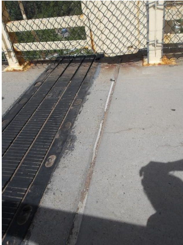
Photo 17- Missing joint material and debris accumulation at north end of pedestrian walkway.
