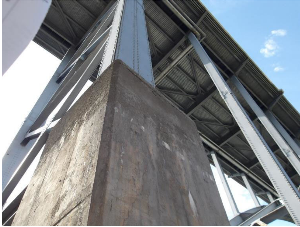
Photo 96- Spalling and debonding (6"x full width of column) of the concrete at the west face of northwest skewback column. This condition extends 2' into the north face of the column.
