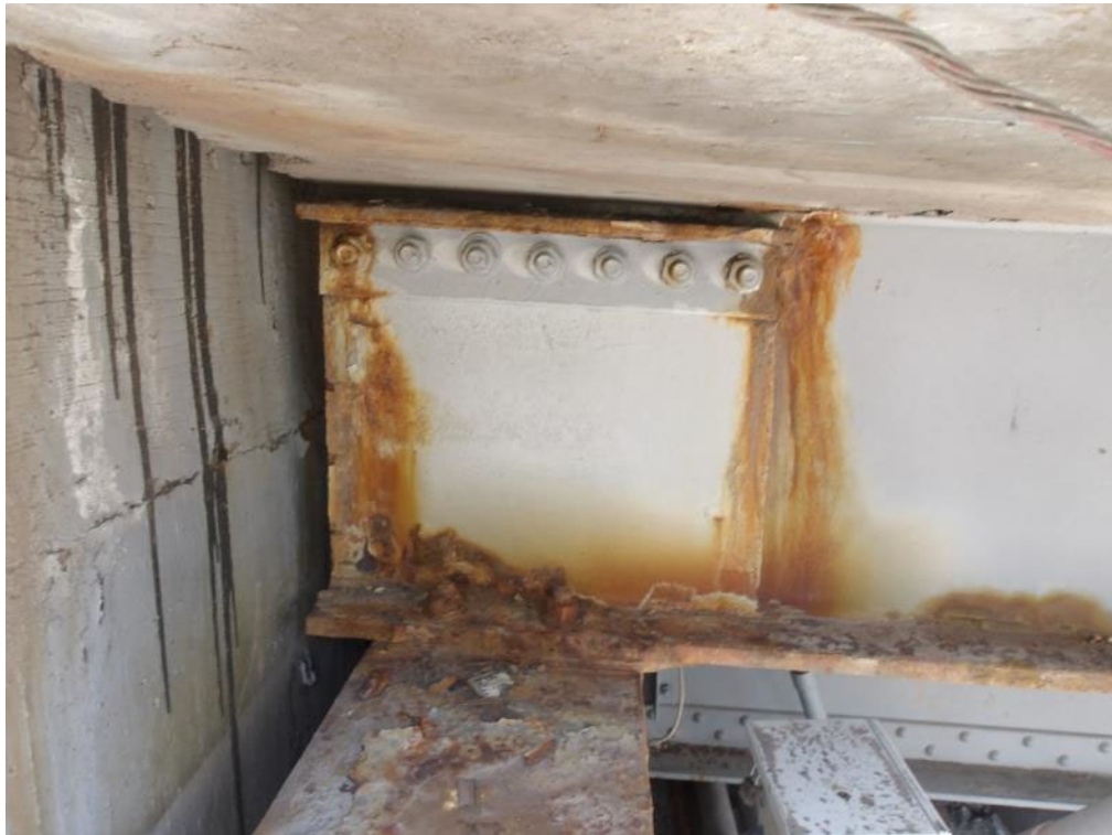
Photo 64- East exterior stringer at south abutment, moderate corrosion in bottom flange and web.
