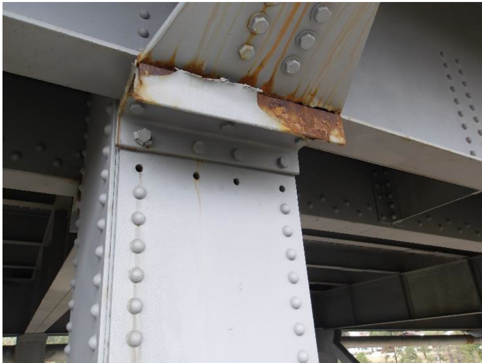
Photo 42- Mis-punched holes at top of arch column 14.
