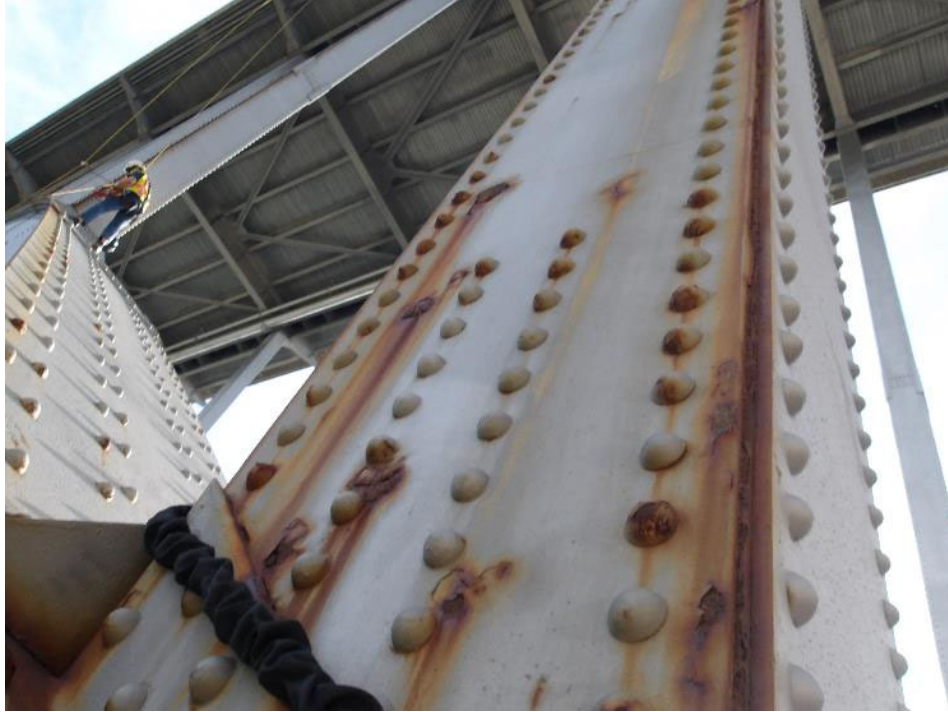
Photo 35- Arch column 1W, minor corrosion and paint failure at base.
