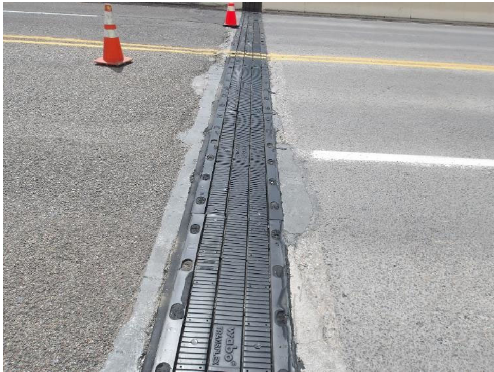
Photo 3- South expansion joint looking west. Note small spalls and delaminations (up to 1') at both edges of the deck joint.
