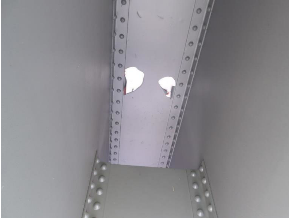
Photo 45- General view of inside top plate and angles of spandrel girder with small areas of failed paint with no corrosion, otherwise in good condition.
