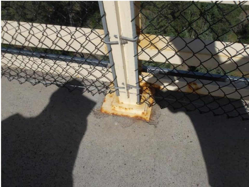
Photo 14- Corroded base plate with small spalls on surrounding walkway.
