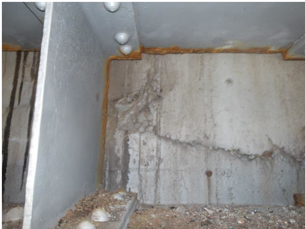
Photo 69- 6"x1' spall between stringers 4 and 5 at the south abutment.
