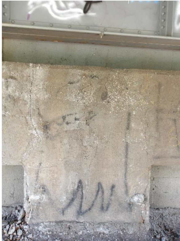
Photo 76- Vertical cracking and small spalls at center of north abutment.
