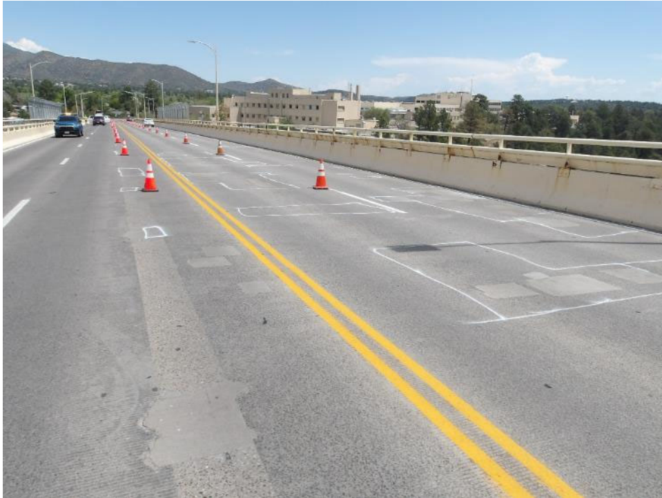
Photo 1- Elevation view of deck, looking north. White outlines indicate locations of deck delaminations.
