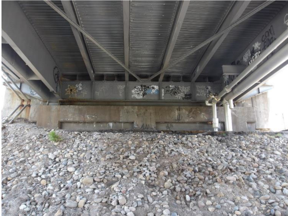
Photo 74– Elevation view of north abutment. Debonding of concrete protective coating is present throughout the abutment.
