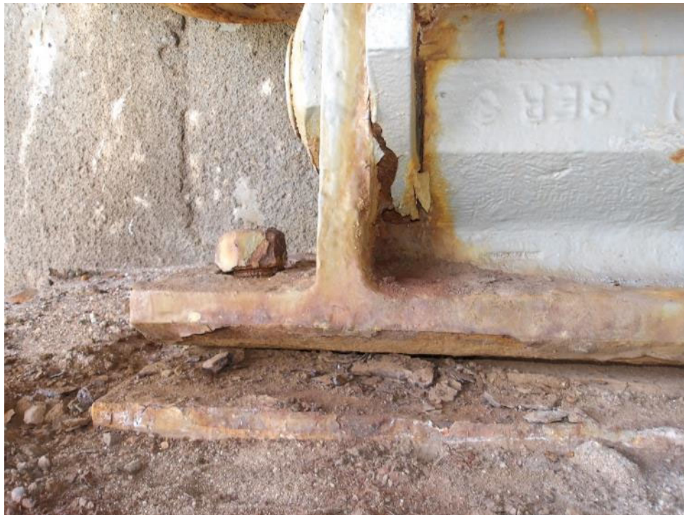
Photo 86- Northwest rocker bearing with paint failure and laterally displaced bolt with partially threaded nut.
