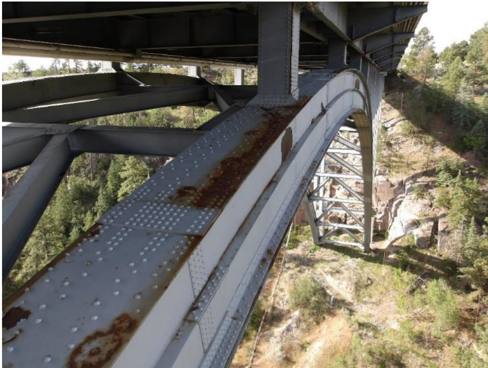
Photo 24- Minor corrosion on top plate of west arch between columns 10 and 9.
