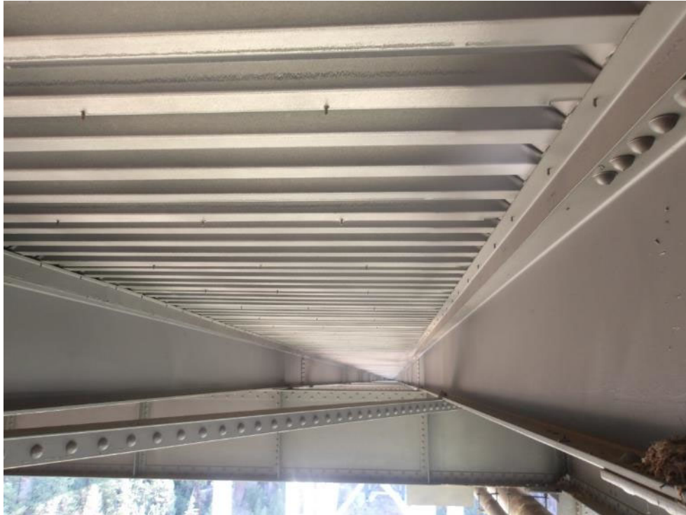
Photo 61- General view of the interior stringers in good condition.
