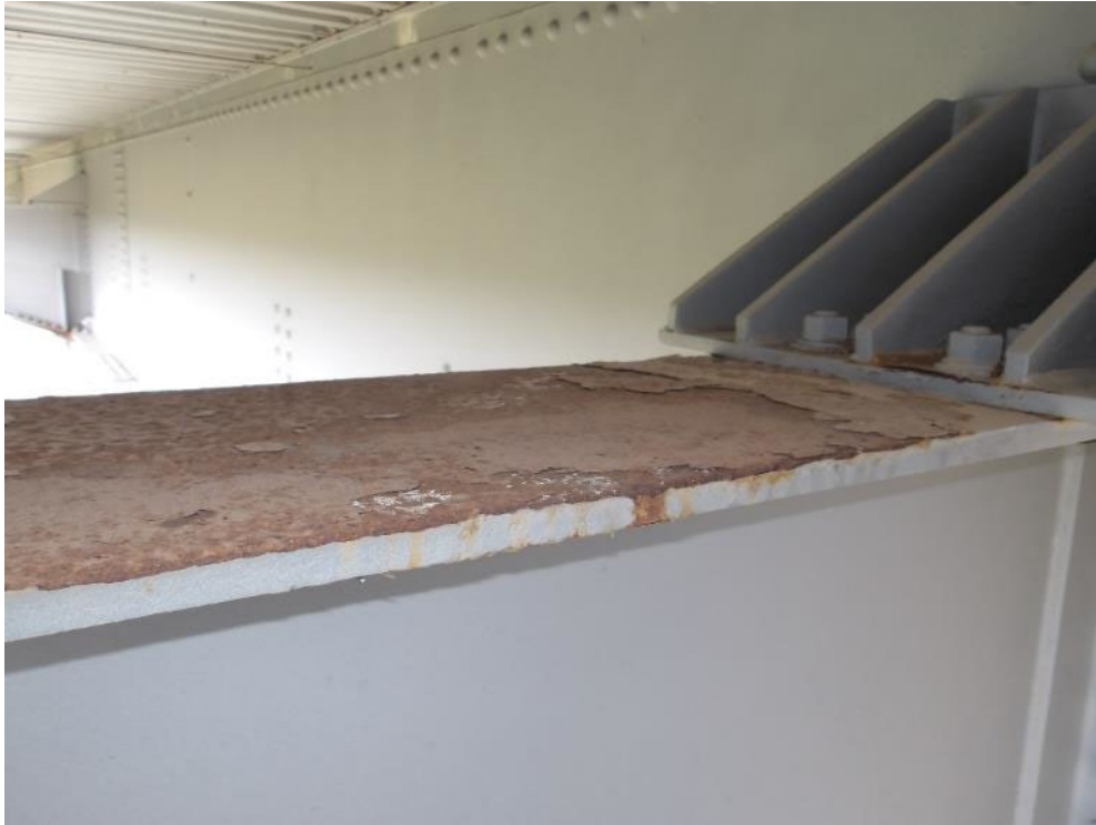
Photo 51- Top of outrigger at arch column 6 on east side, minor surface corrosion, no measurable section loss.
