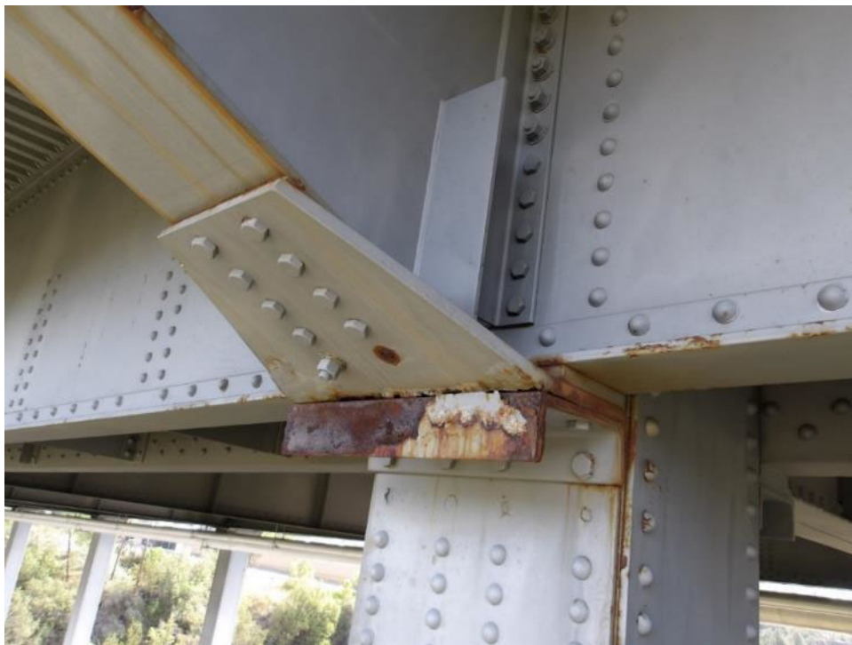
Photo 52- Missing nut and broken bolt at outrigger gusset plate at arch column #8, west. Moderate corrosion and pack rust between channel and bottom of outrigger.
