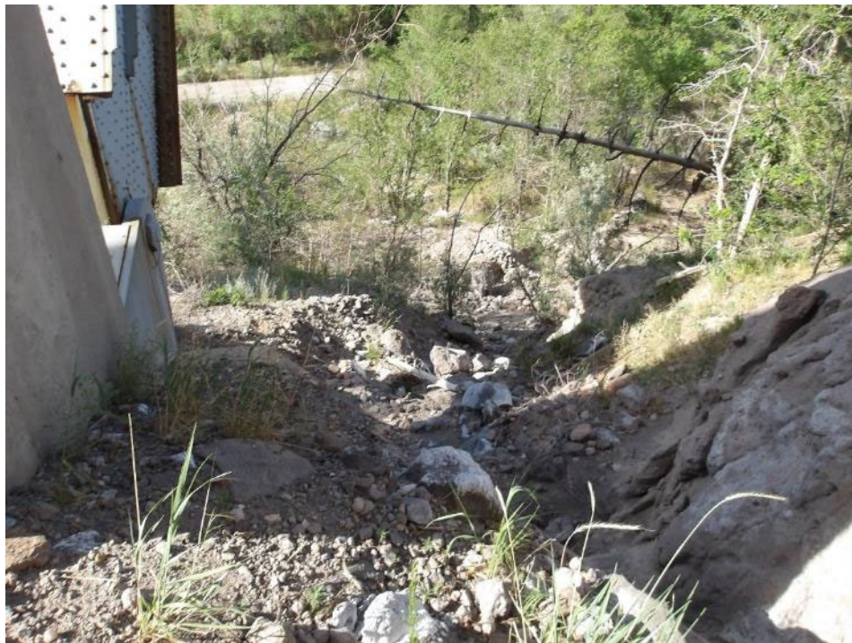
Photo 97- View of erosion running down canyon wall immediately west of the northwest skewback column.
