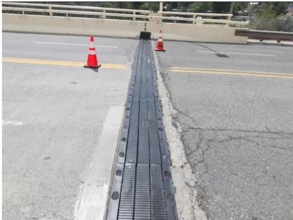
Photo 2- North expansion joint looking west; small spalls and delaminations (up to 1') along both edges of the deck joint.
