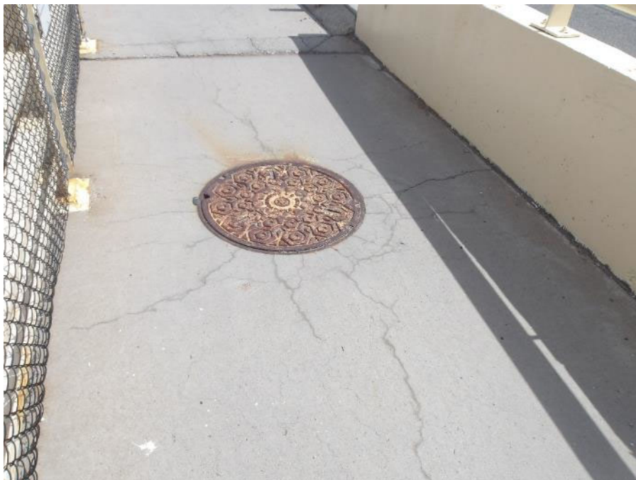
Photo 12 – Map cracking at manhole cover at north approach of pedestrian walkway. Map cracking is typical throughout the pedestrian walkway.
