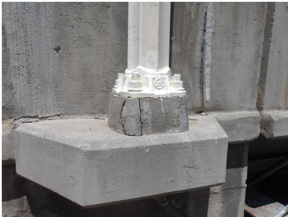
Photo 9- Repainted light pole and support with cracking at light pole foundation.
