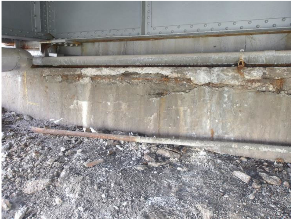
Photo 66- Delamination, spalling and exposed rebar at south abutment.
