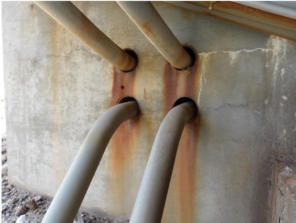
Photo 78- Rust staining and horizontal crack with efflorescence on west backwall at north abutment.
