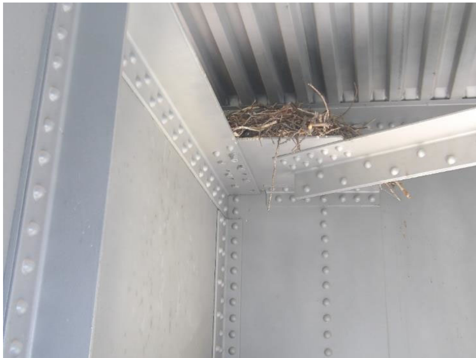
Photo 60- Bird nest on top of connection plate and floorbeam top flange, noted in multiple locations on bridge, east side floorbeam at south skewback column shown.
