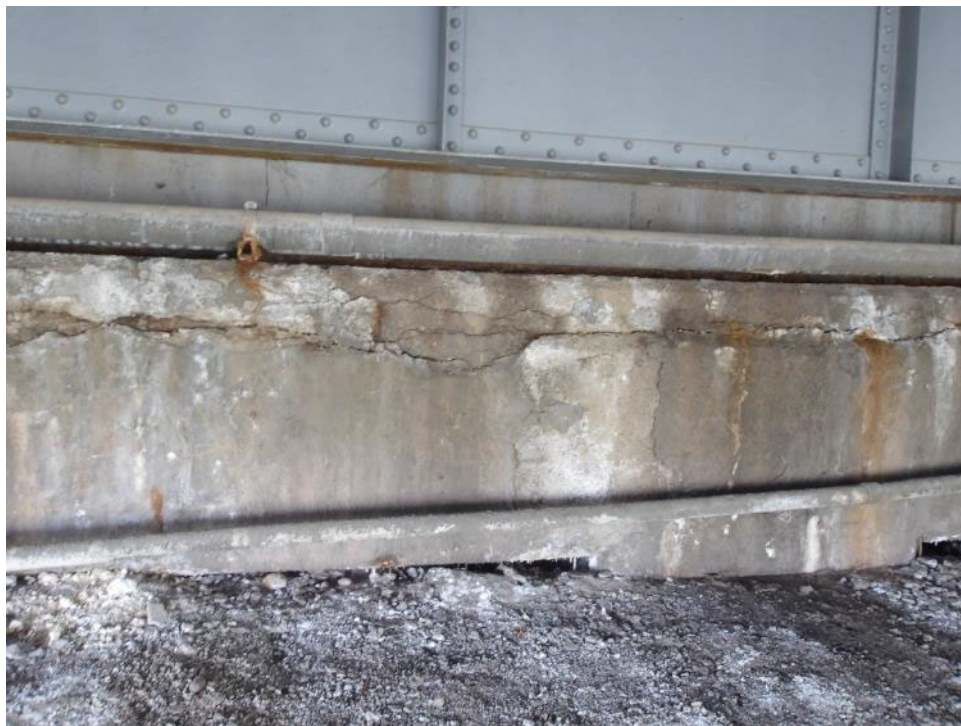
Photo 67- Efflorescence leaking down the face of the south abutment top strut.
