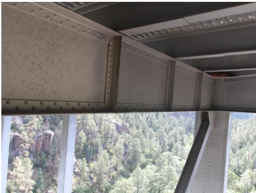
Photo 56- Floorbeams are generally in good condition. Floorbeam at south skewback shown.
