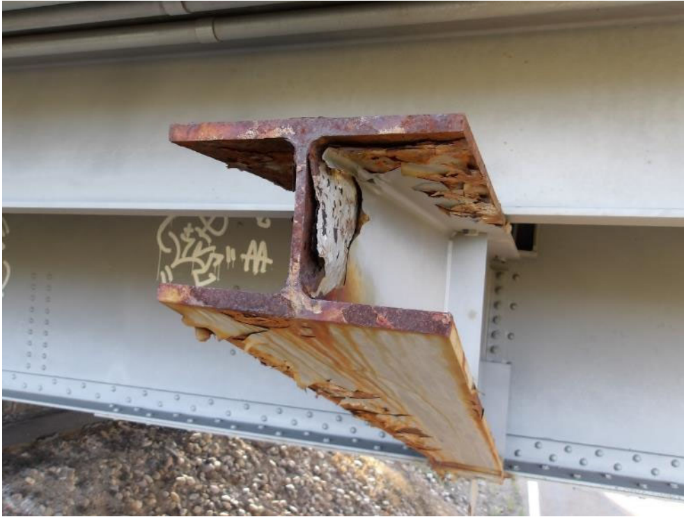
Photo 47- End of outrigger at FB27 west side, moderate corrosion and minor section loss in zero stress area.
