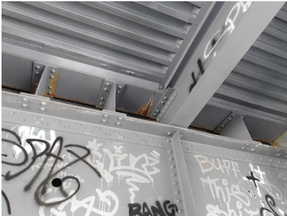
Photo 81- Cracked steel plate at north abutment.
