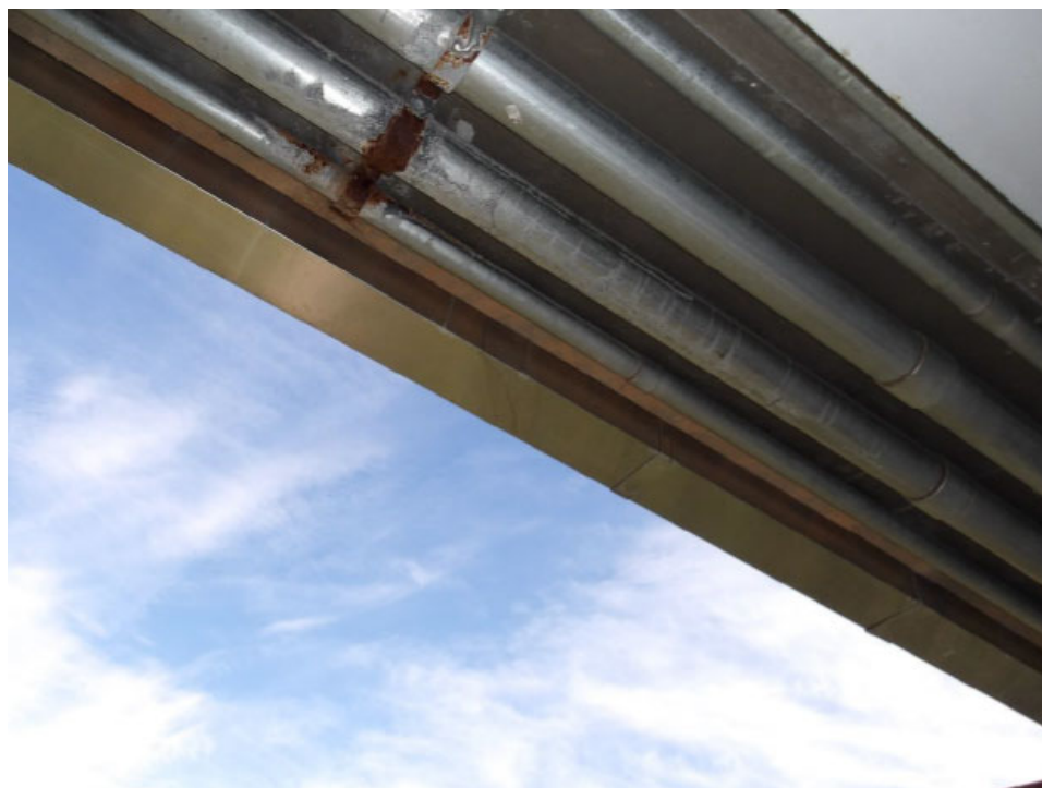
Photo 10- Utility pipes at west overhang. Heavy corrosion at the utility pipe clips. This defect is typical at all utility pipe clips at the west overhang.
