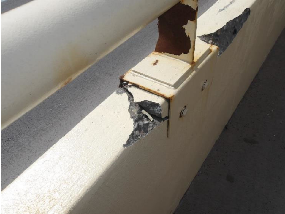
Photo 115- Spall and cracking of concrete at the west guardrail-concrete barrier rail connection towards the north end of the pedestrian walkway.
