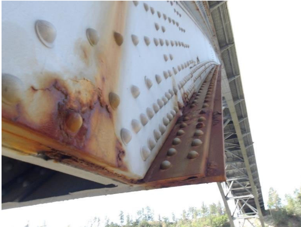
Photo 27- Minor corrosion at north end of west arch at the bearing.
