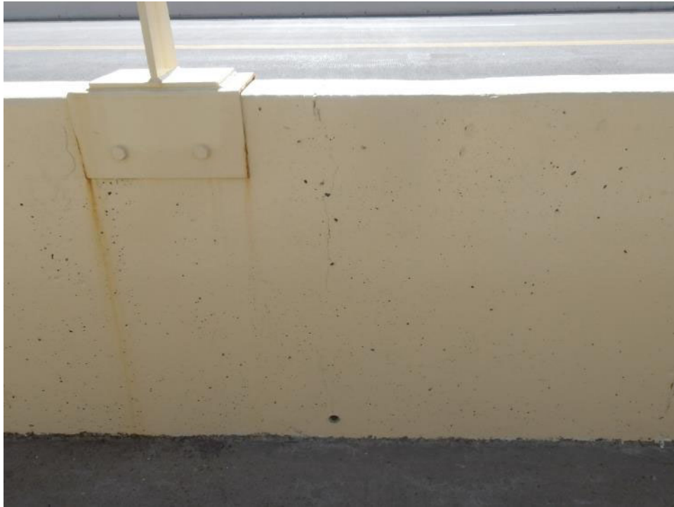
Photo 107- Vertical hairline crack in the west concrete barrier rail emanating from drain hole at bottom (TYP).
