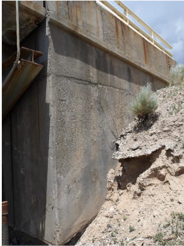
Photo 80- East wingwall at north abutment, hairline cracking. Undermining at south end of wall, wrapping around to the backwall.
