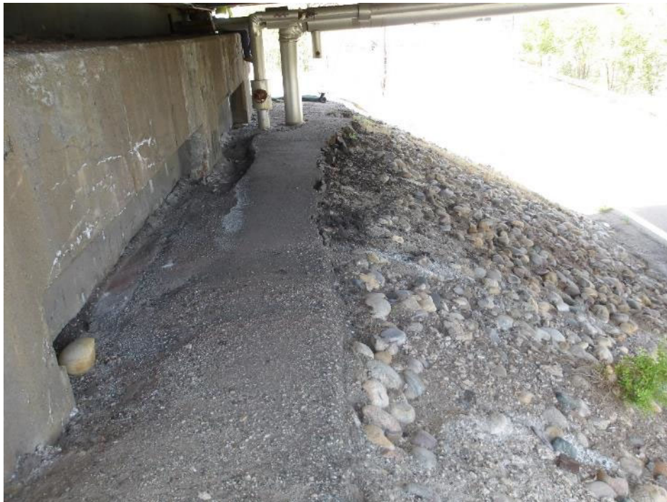
Photo 83- Erosion of asphalt at north abutment.
