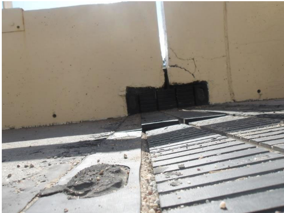
Photo 4— \frac{3}{4} " vertical displacement in south expansion joint at pedestrian walkway.
