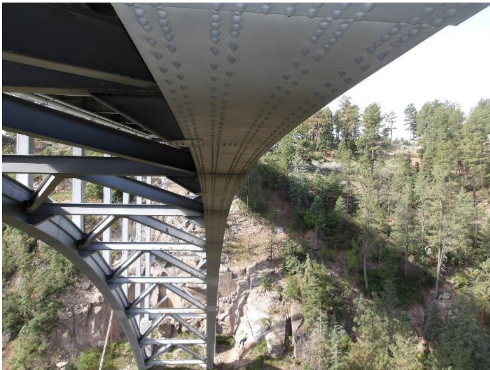
Photo 26- Bottom of steel arch in good condition, at west arch center span looking south.
