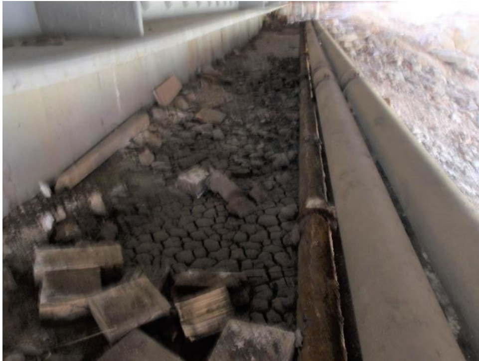
Photo 68- Top of south abutment strut. Three pipes with anchorages into the strut exist. The strut is covered in dirt and debris.
