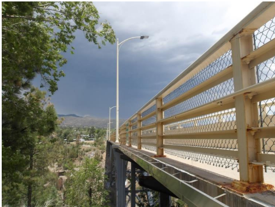
Photo 18- Drainage system (gutter) on west side of deck.
