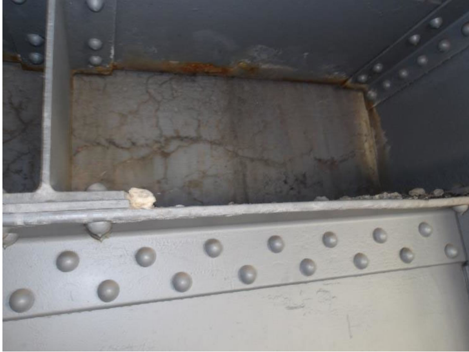
Photo 70- Cracking along southern abutment between stringers 2 and 3. Typical at the southern abutment.
