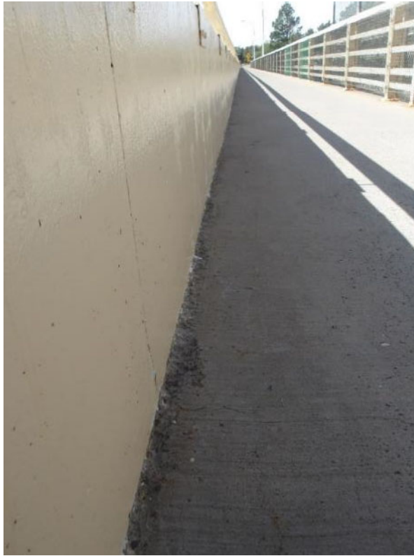
Photo 15- Undermining of the concrete bridge barrier towards the north end of the raised section of the fence.
