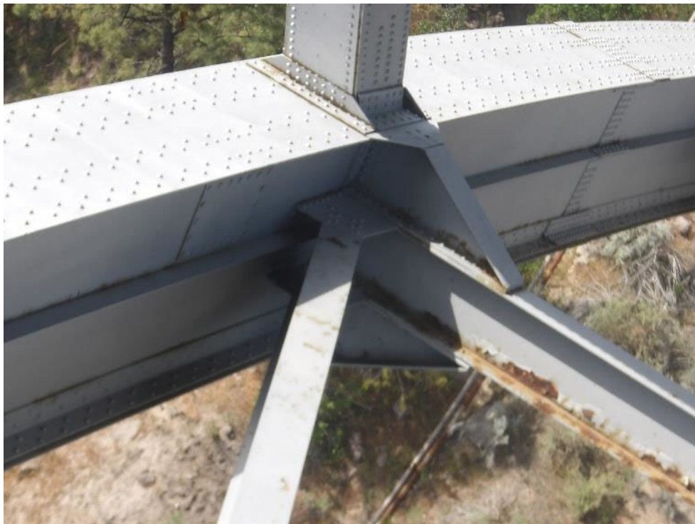
Photo 30- Bracing connection at arch column 4 on E arch, paint failure and minor corrosion, typical.
