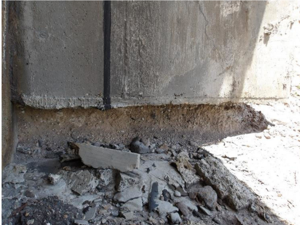
Photo 82- 48"x6" area of undermining at the east back wall of the north abutment.
