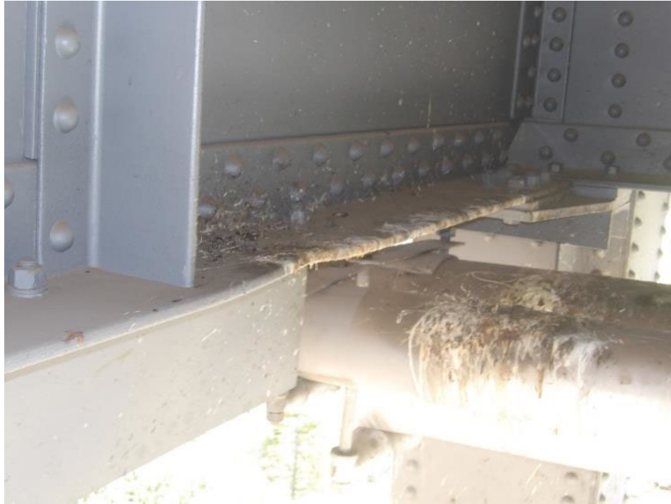
Photo 59- Typical minor deformation in bottom flange angle of floorbeam, east end of FB at column S1 shown.
