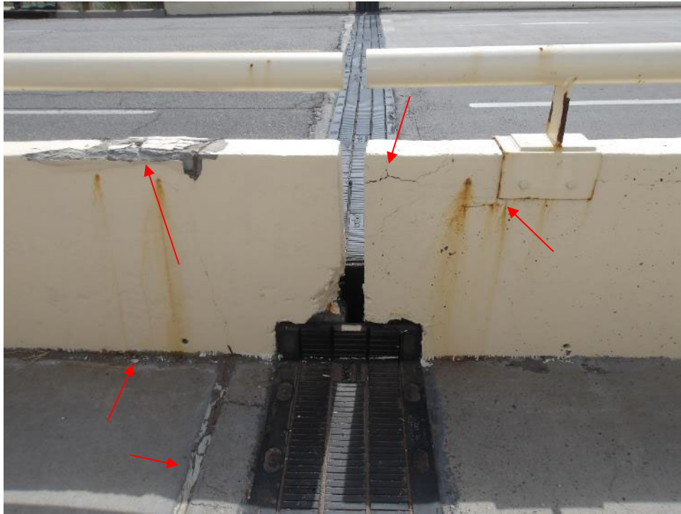
Photo 109- Spall (2'x Full Width x 1/2"), 1/8" cracks, section loss, and rust staining at the west concrete barrier rail at the north joint. Note undermining of concrete barrier rail and missing joint material.
