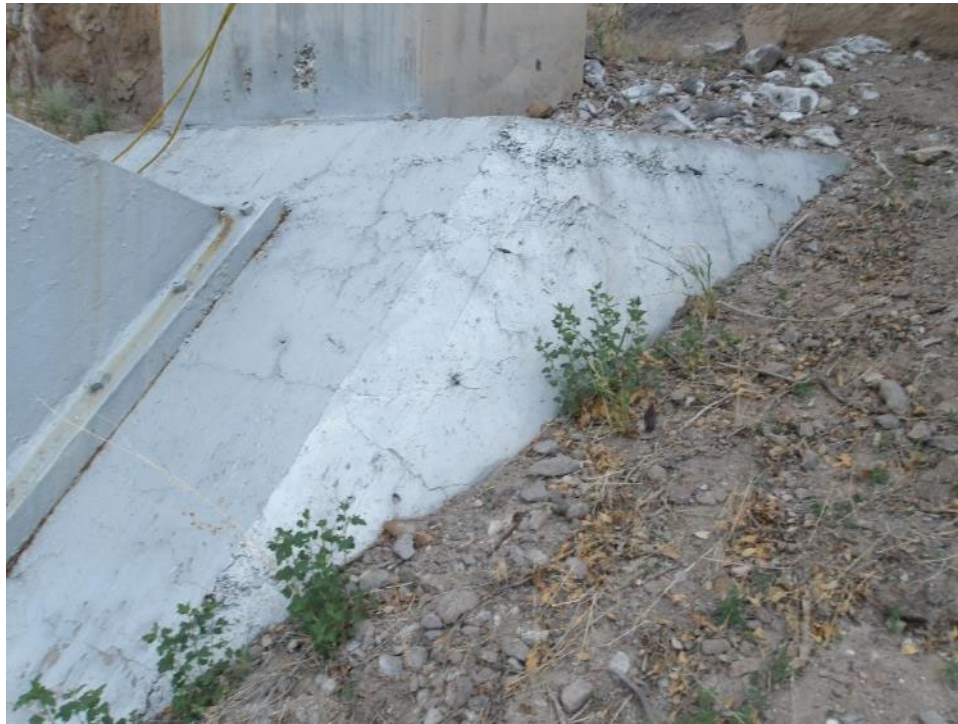
Photo 98- Map cracking throughout the east face of the northeast arch base.
