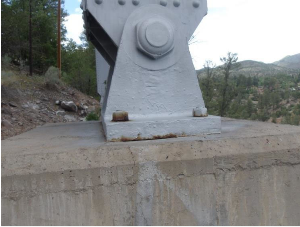
Photo 90- Minor paint failure of the eastern bolts and bottom edge of the bearing at concrete pier column 2, east. Note vertical hairline crack along eastern face and pier cap. This crack extends down the height of the pier column.
