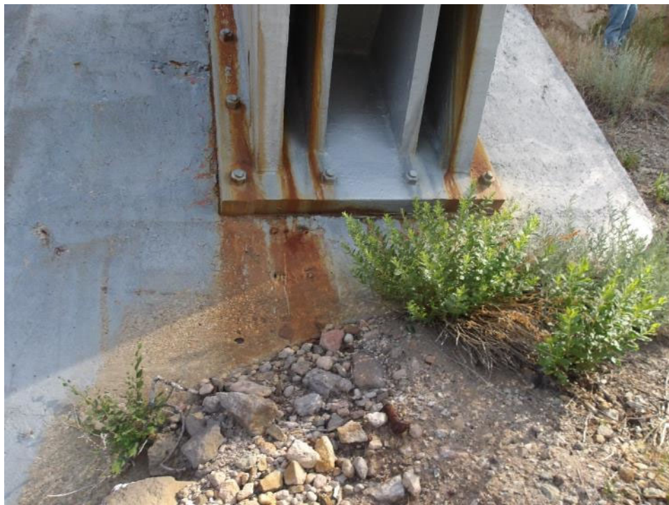
Photo 99- Map cracking and rust staining at south face of northwest anchor base.
