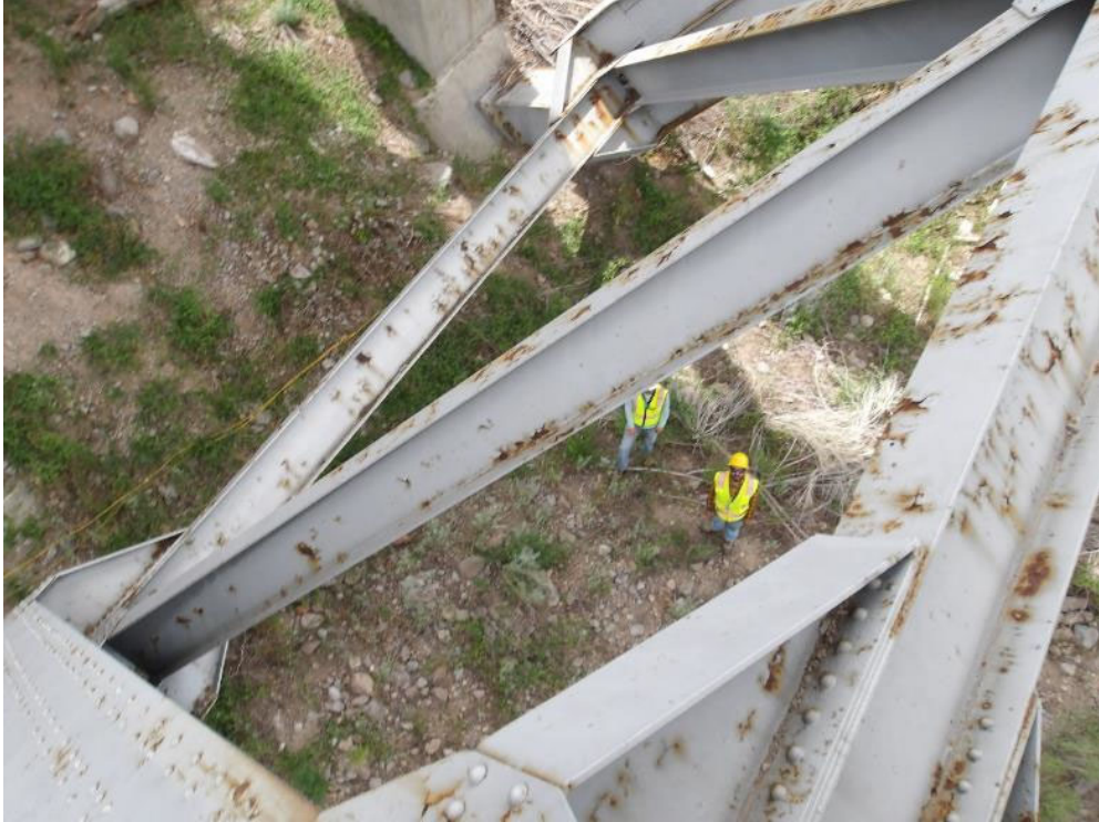
Photo 29- General condition of bracing with minor corrosion and paint peeling at south end, looking west from arch column 1.
