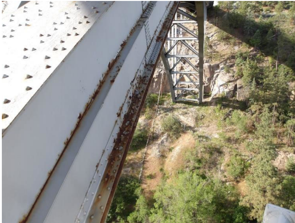
Photo 23- Minor corrosion on top of bottom flange of west arch rib at column 11.
