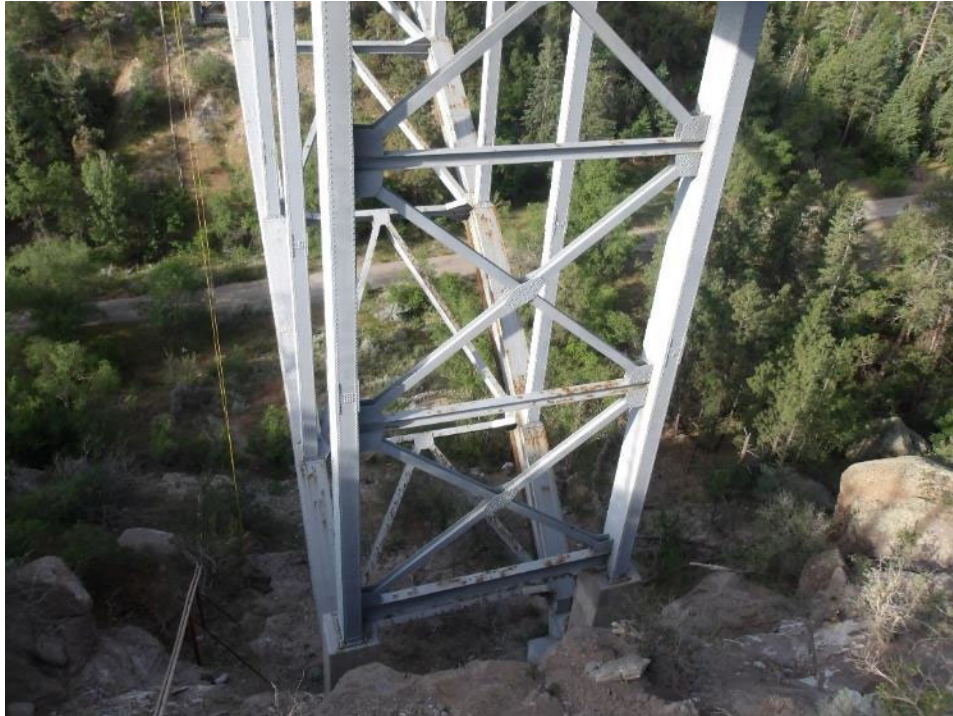
Photo 100- View of North skewback columns. Minor paint peeling and corrosion on bracing members.
