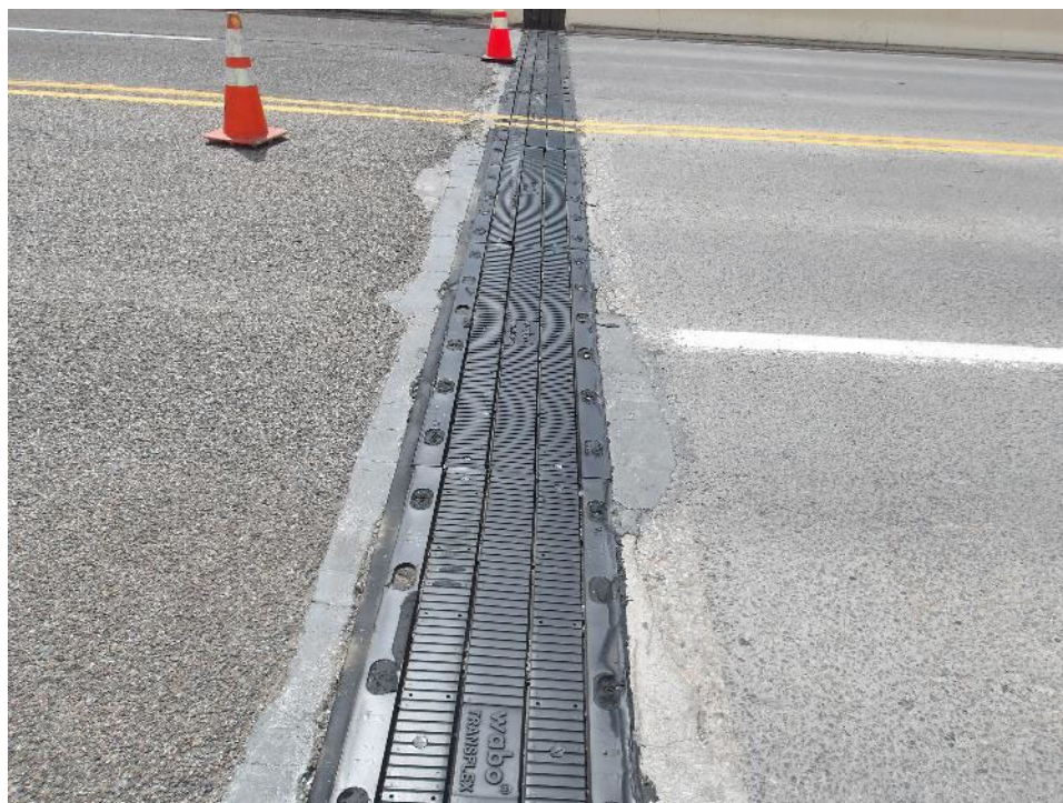
Photo 106- Deterioration of asphalt and concrete on the approach side at the south abutment joint.
