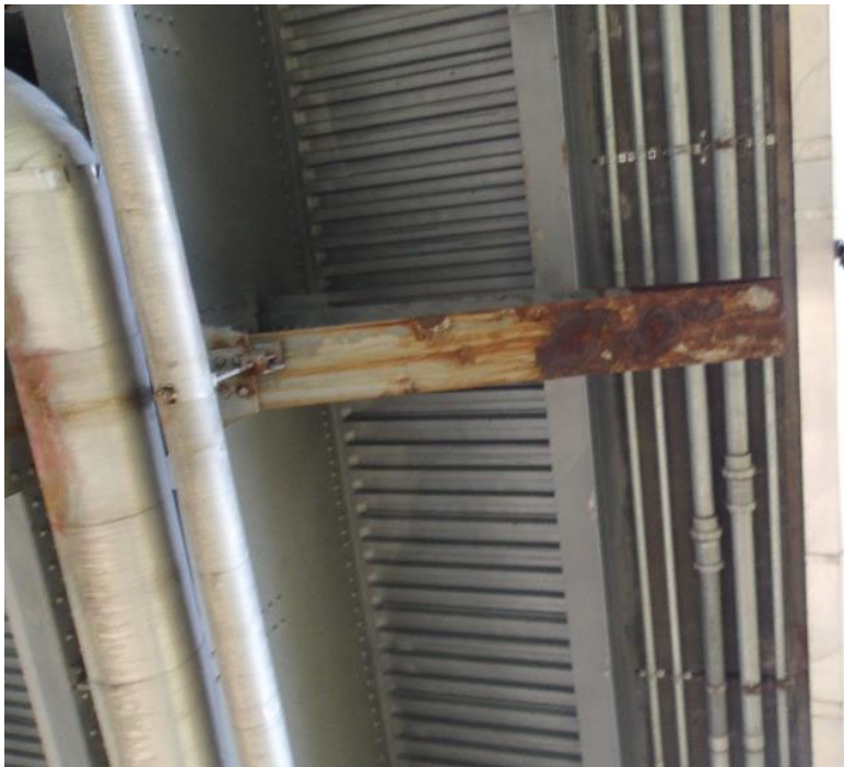
Photo 48- End of outrigger at column 1W west side, moderate corrosion and section loss in zero stress area past the stringer. Minor corrosion with no section loss from stringer to spandrel girder.
