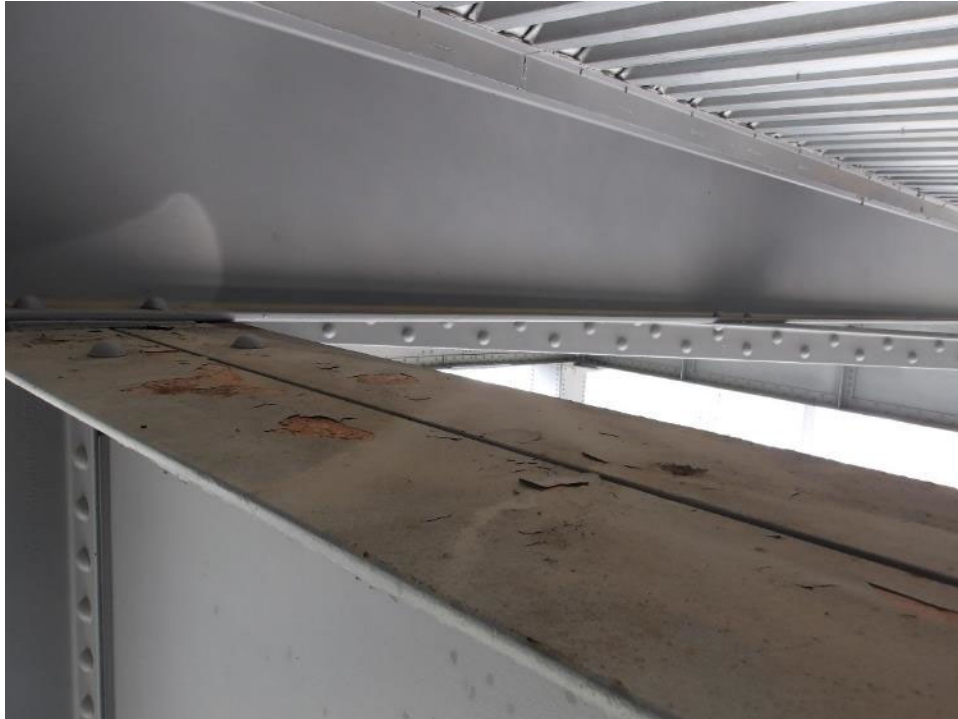
Photo 57- Minor paint peeling on top flange of floorbeam typical.
