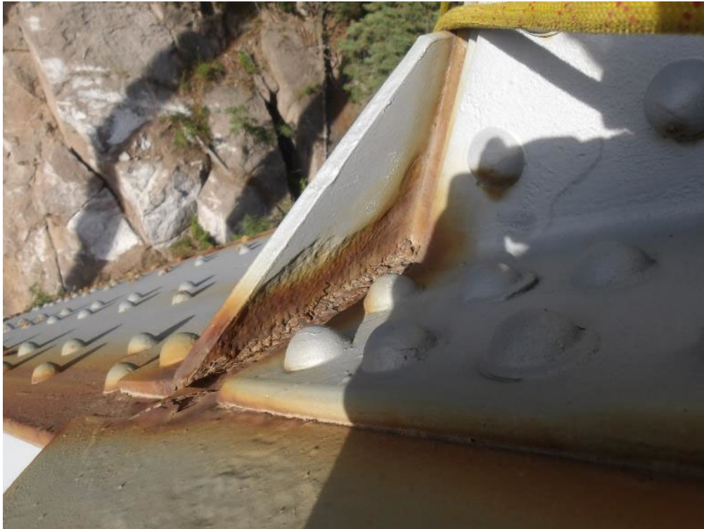
Photo 38- 1/16'' thickness loss to vertical gusset plate at arch column 2W.
