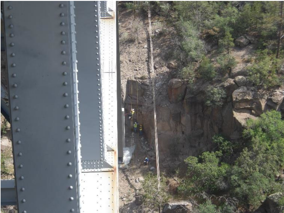
General Photo 8 – Use of rope access for inspection.
