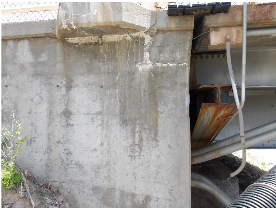
Photo 79- West wingwall at north abutment, hairline map cracking. Efflorescence around light pole pedestal and concrete cutout for joint.
