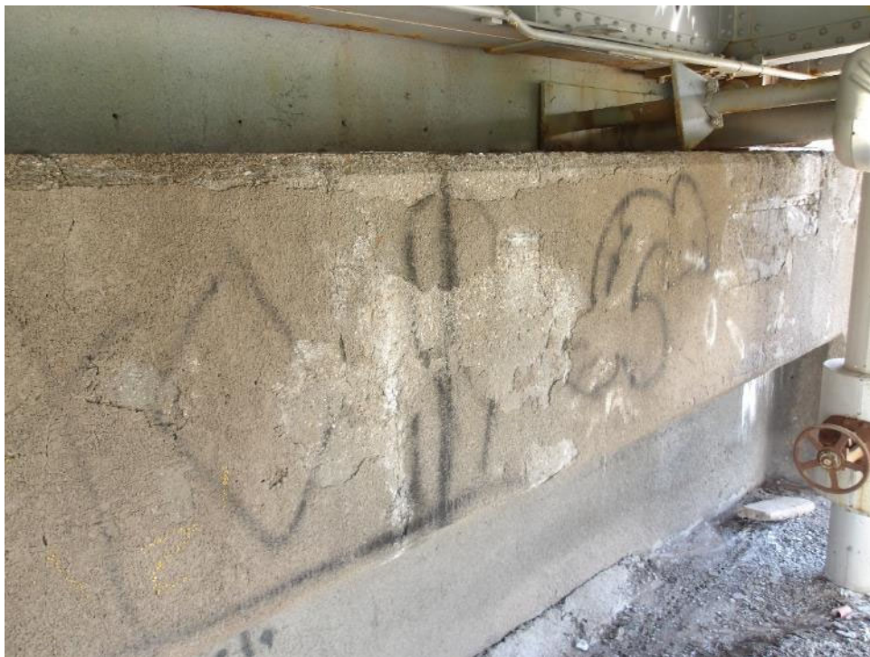
Photo 75- Debonding of concrete protective coating at north abutment. Also, hairline vertical and horizontal cracking along the top strut.
