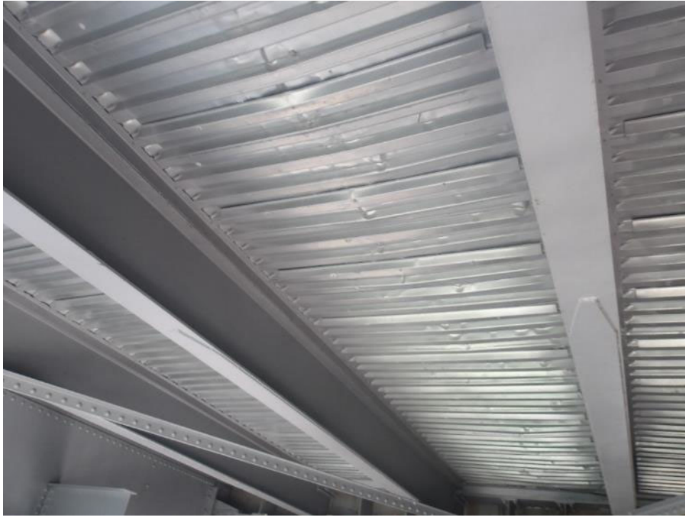
Photo 7- Minor damage throughout the stay-in-place forms at span 1. Typical up to bay 4.
