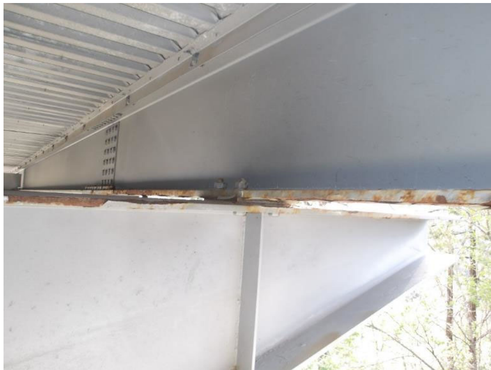
Photo 62- General condition of exterior stringer with peeling paint and surface corrosion on the bottom flange.
