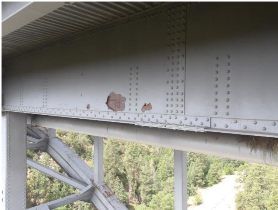
Photo 44- General view of spandrel girder in satisfactory condition, east face near arch column 13E. Paint peeling and minor corrosion.
