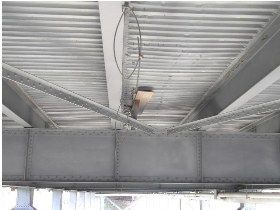
Photo 6– Temporary support at failed stay in place forms at Floorbeam S14.
