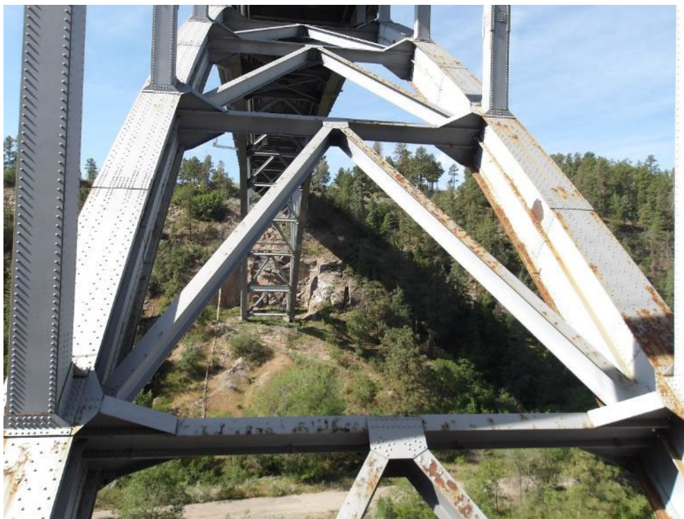
Photo 28- General condition of bracing with minor corrosion and paint peeling at north end, looking south from skewback column.
