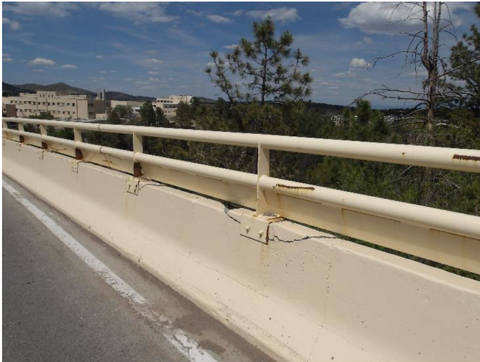
Photo 116- Impact damage on the east bridge rail near the south abutment has caused cracking and spalling of concrete with complete separation of concrete at 6 connections.
