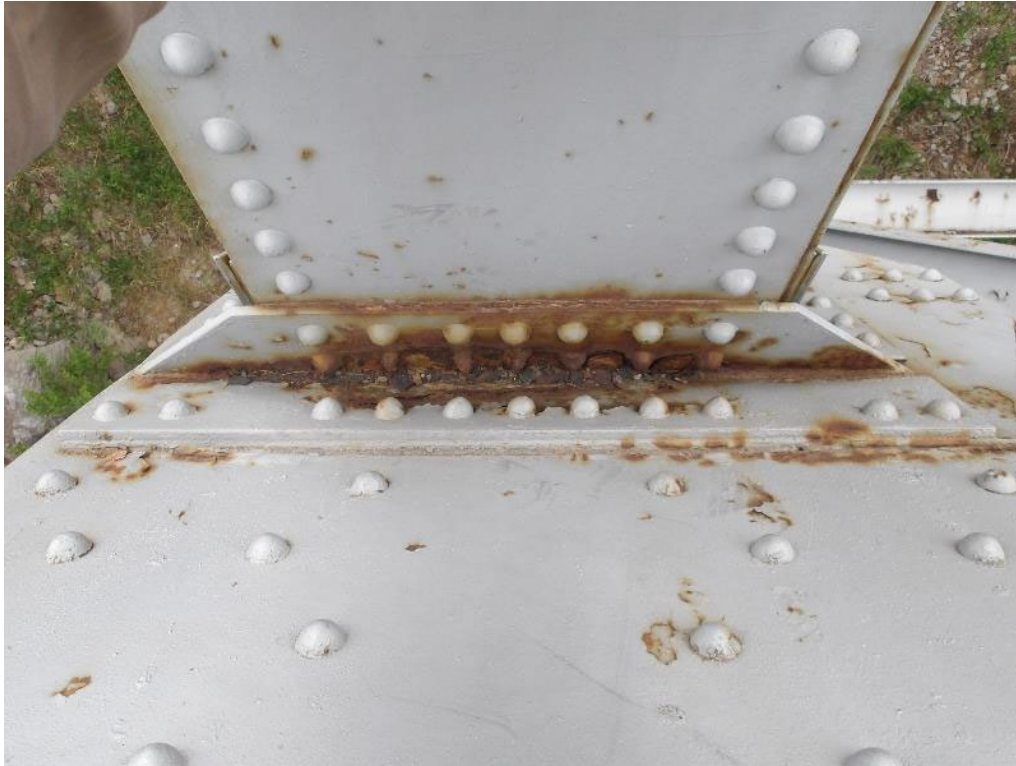
Photo 39- Moderate corrosion and section loss to rivet heads on N side of arch column 1E.
