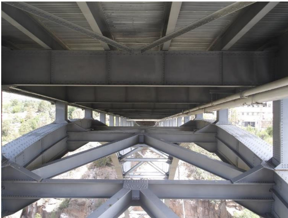
Photo 32- General view of bracing at center of arch in good condition.
