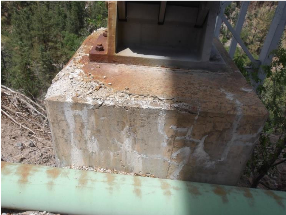
Photo 91- Large spall at the southwest corner and along the western and southern top edges of concrete pier column 2, west. Photo is looking north.
