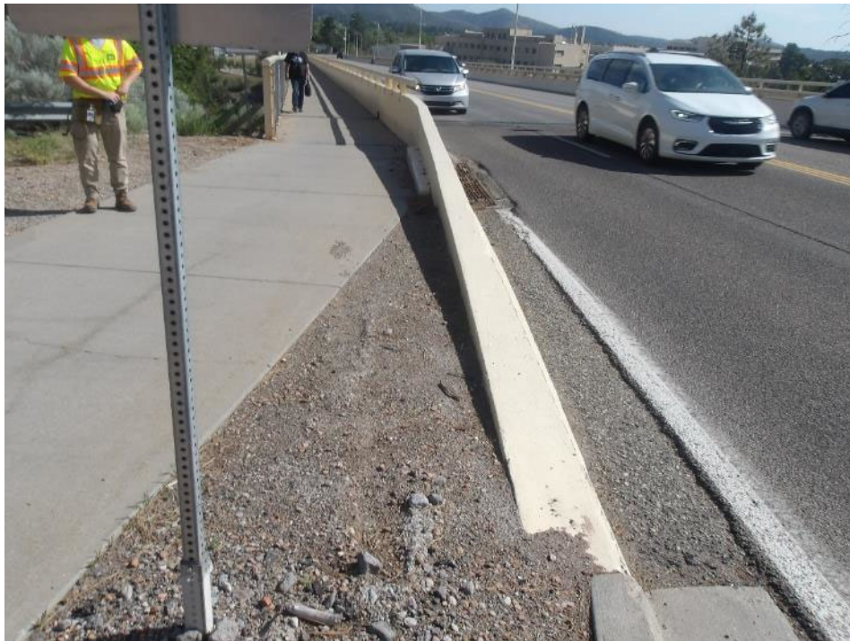
Photo 120- Southwest approach concrete barrier rail transition, looking south.
