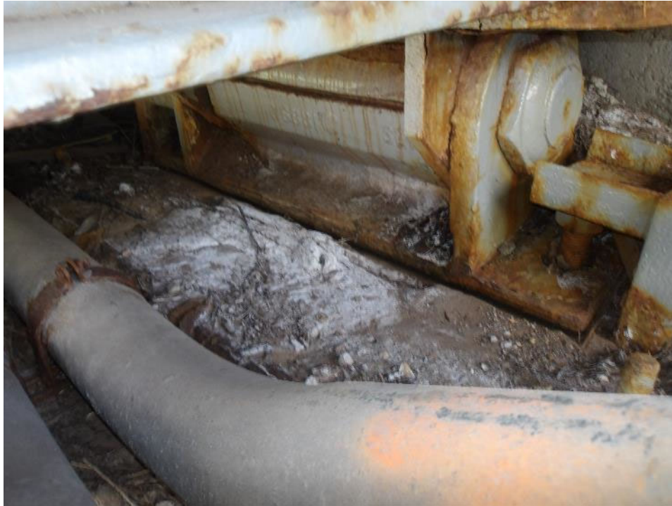
Photo 84- West bearing at south abutment with corrosion, rust staining and debris buildup.
