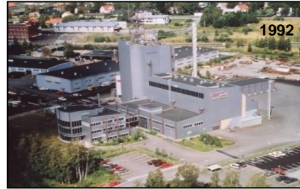
80 ton per day Gasification Plant in Finland using biomass & coal
