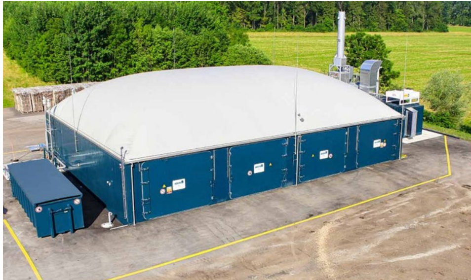
Figure 9. Small plant digester system (Photo from Bekon)
