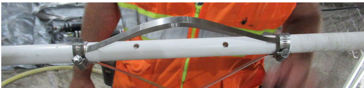
Figure 4. Conveyance pipe for down-going hole, perforated to allow grout to fill it.
