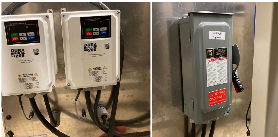
Figure D3. 480 V VFDs and local disconnect.
