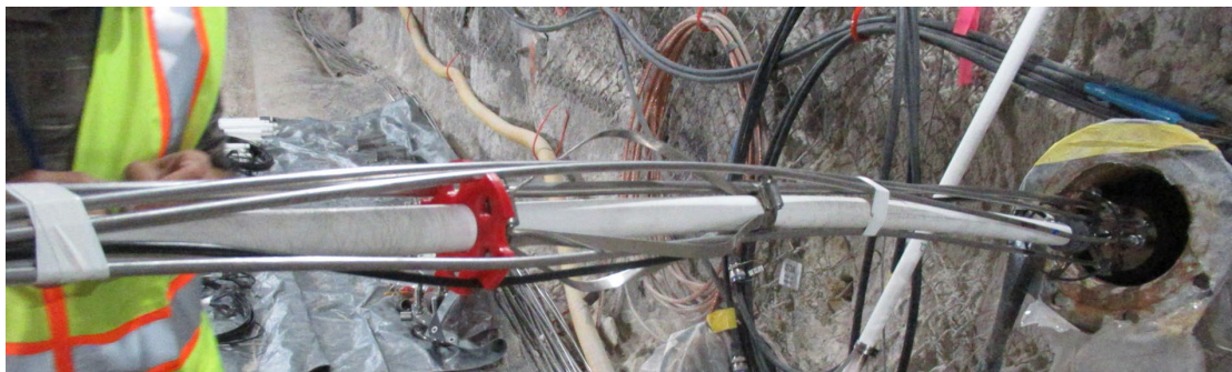
Figure 3. Conveyance pipe, centralizer, and spacer.
