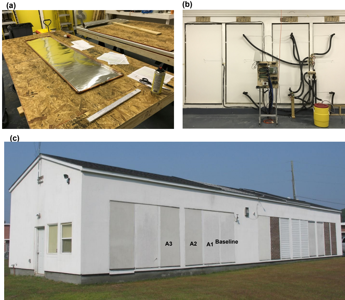
Figure 2. Field installation of TABE wall panels at the Charleston NET facility: (a) panel preparation and (b) panel installation; and (c) exterior of the NET facility.
