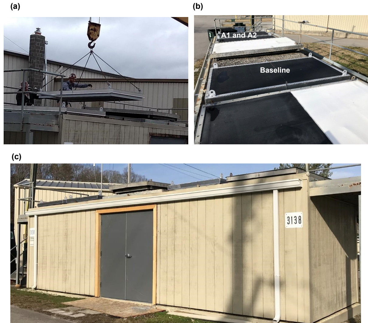
Figure 1. Field installation of TABE roof panels at the RTRA in Oak Ridge: (a) lifting panels into place and (b) after installation; and (c) exterior of the RTRA test facility.
