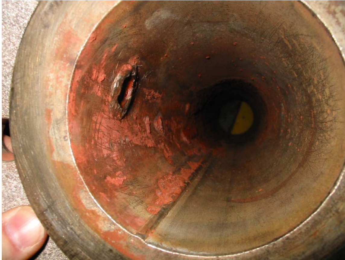
Figure 5.21. Interior of transition line section #3 (post cleaning).
