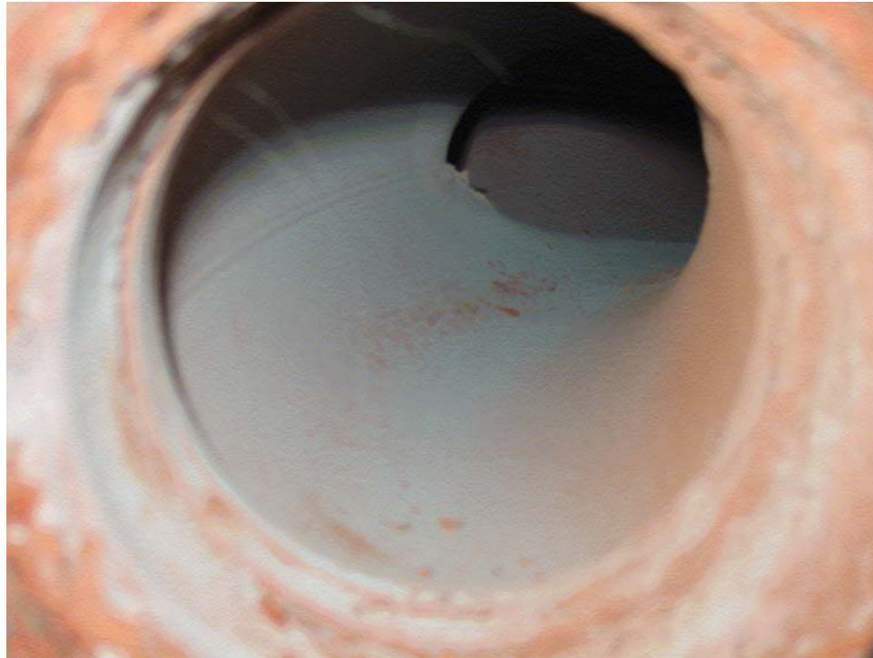
Figure 5.9. Transition line section #1 outlet.
