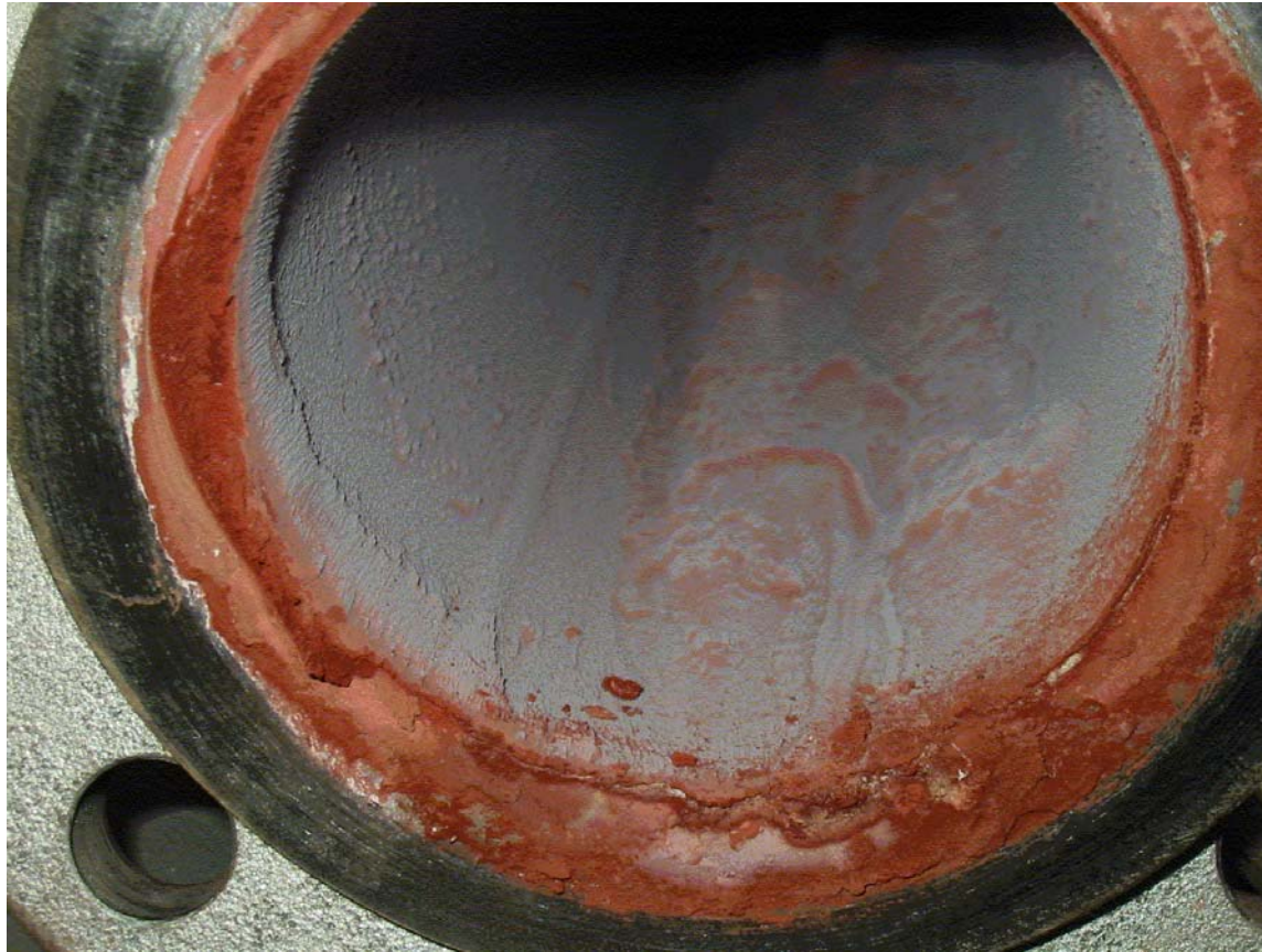
Figure 5.14. Transition line section #3 outlet.
